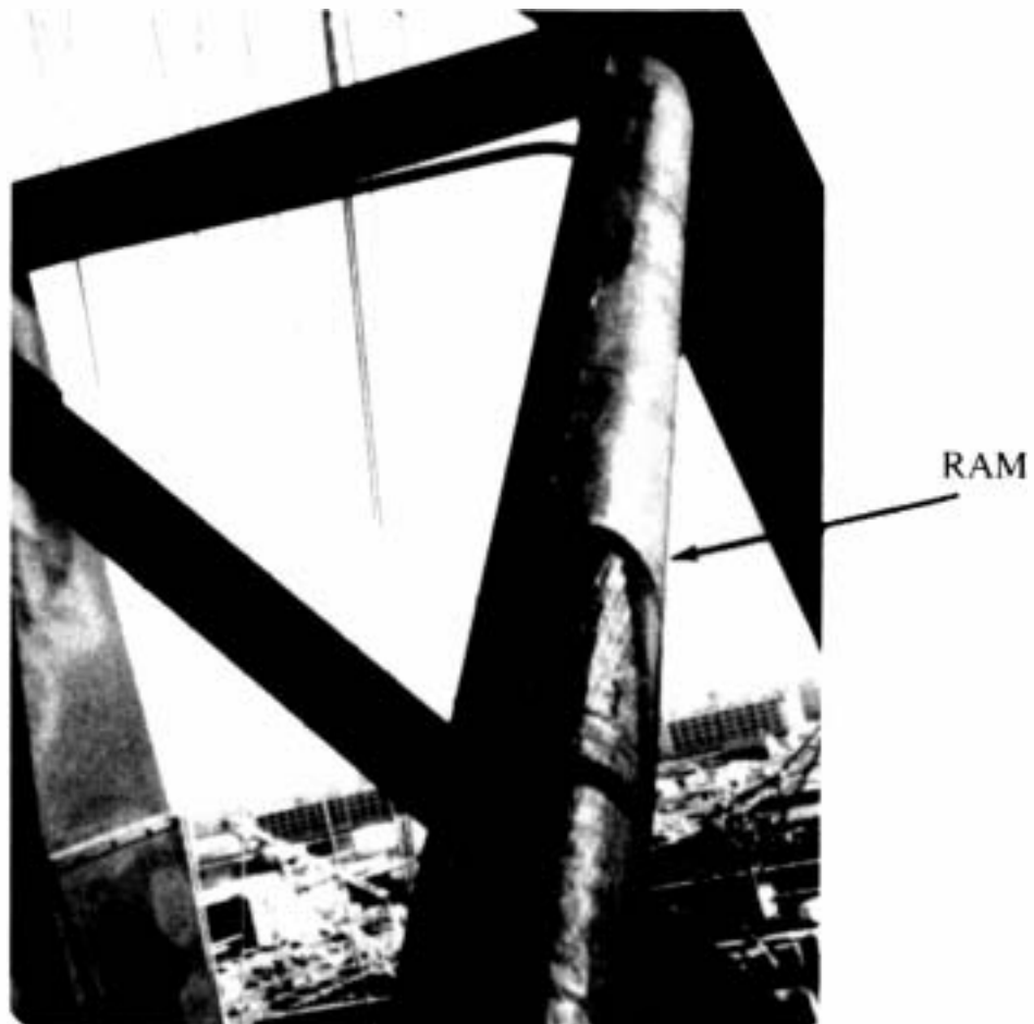
Figure 4-24 RAM Wrapping on Mast Legs to Reduce Reflective Surfaces
