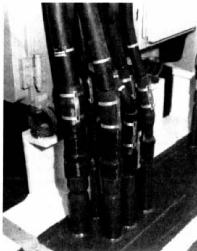
Figure 4-19(b) Flexible Conduit Shielding Topside Cable Runs
