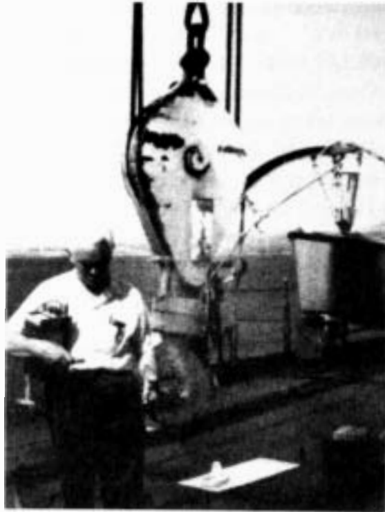
Figure 5-4 Uninsulated Cargo Hook
