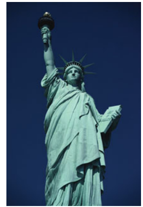
FIGURE 4-25 Recognizable Green Patina from the Oxidized Copper on the Statue of Liberty
