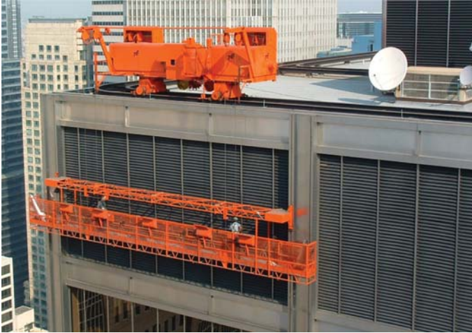
Figure 4. Rooftop carriage supporting a platform. The carriage is supported by parallel rails that run along the roof perimeter.
