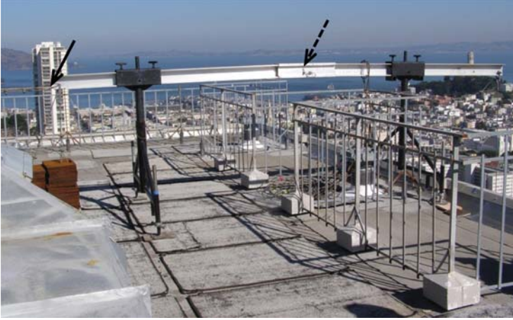
Figure 2. Portable, contractor-supplied outrigger. Note the tieback cable (black arrow) at the interior end of the outrigger (dashed black arrow). In this case, the outrigger is provided by the contractor and is considered temporary, and its design is not covered by this guideline. The tieback cable would be attached to a tieback anchorage that is covered by this guideline.
