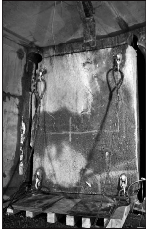
Figure 6. Cut slurry wall panel prepared for removal
