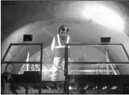
Photograph 7. Application of membrane—yellow first coat
