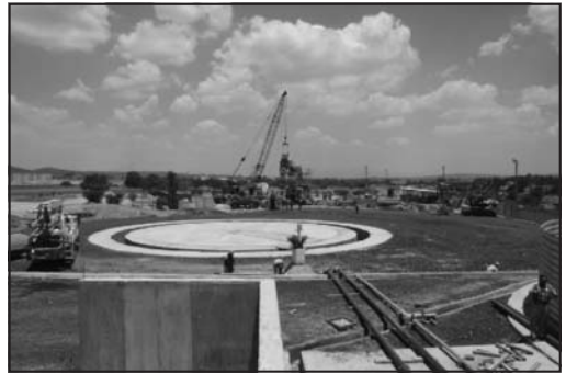
Figure 11. Slurry wall construction, Shaft 20, November 2009
