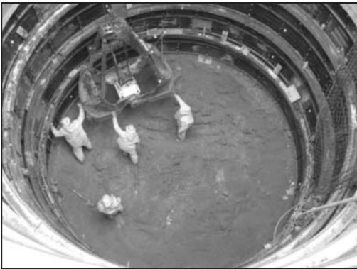
Figure 13. Shaft excavation with clamshell bucket
