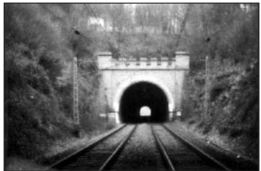
Figure 1. Portal of Buedenholz Tunnel
