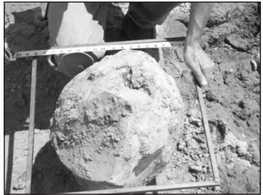
Figure 4. City's construction management team measures obstruction
