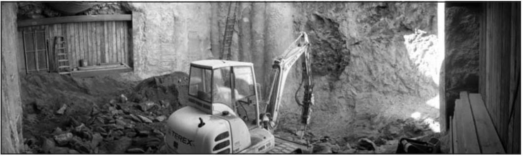
Figure 9. Photo of the diversion structure after completion of the secant pile walls and jet grouting
