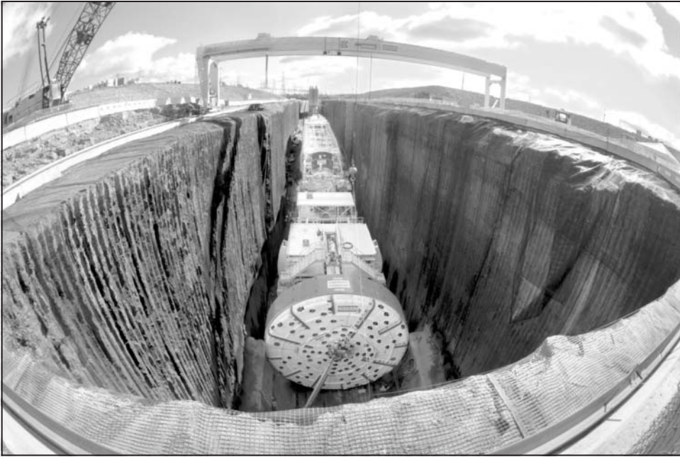
Figure 5. TBM and back-up assembled in launch chamber
