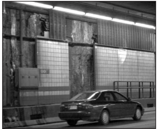
Figure 3. In some tunnels it is necessary to remove precast panels to inspect the tunnel wall
