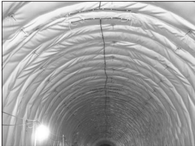
Figure 4. Waterproofing membrane installation
