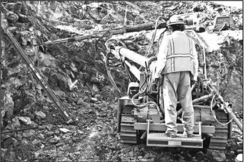
Figure 5. Photographic record of Contract No. 2 surface excavation
