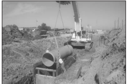
Figure 10. Pipe installation in open trench section
