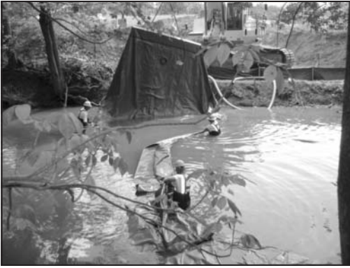
Figure 7. Placing portable dam in Mill Creek before inflating with water
