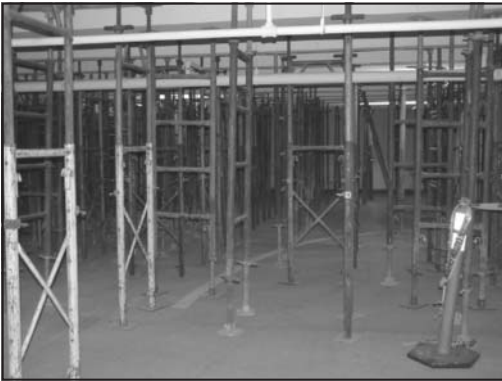
Figure 4. Floor jacks beneath the P3 portal area
