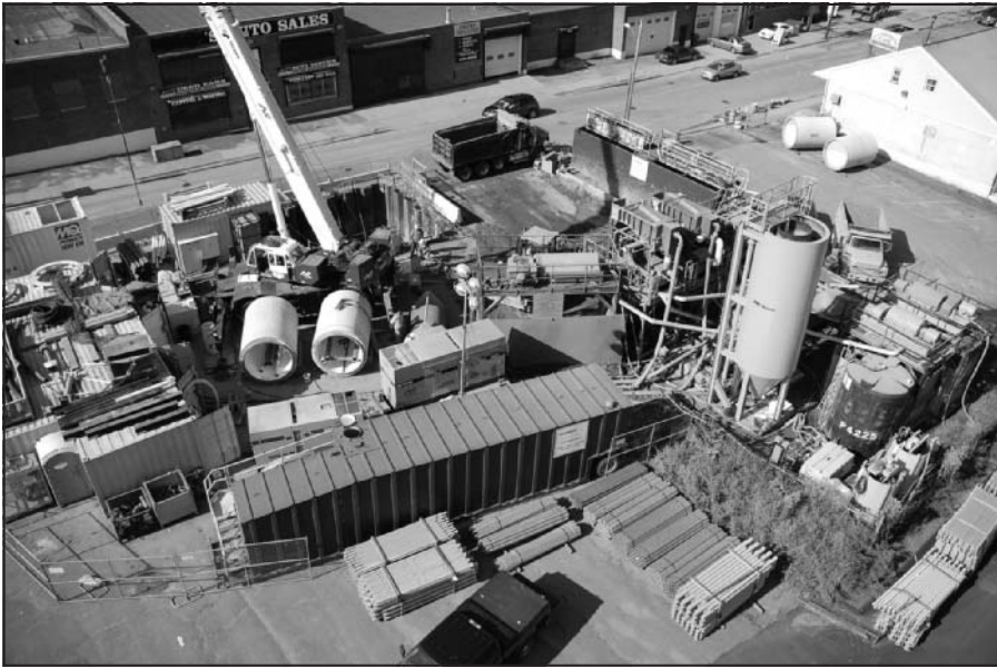
Figure 3. Shaft with equipment layout for tunneling
