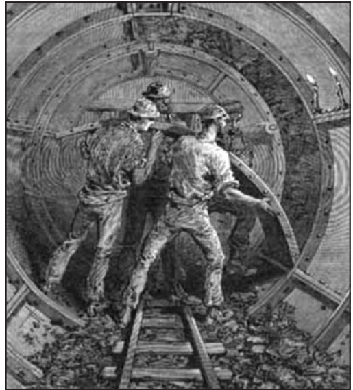
Figure 1. Construction of the Tower Subway, London, 1869, using cast iron segments
