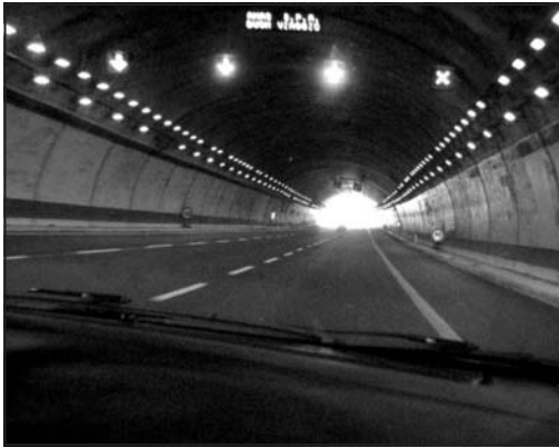
Figure 2. Driving along the finished external bore of Cassia tunnel
