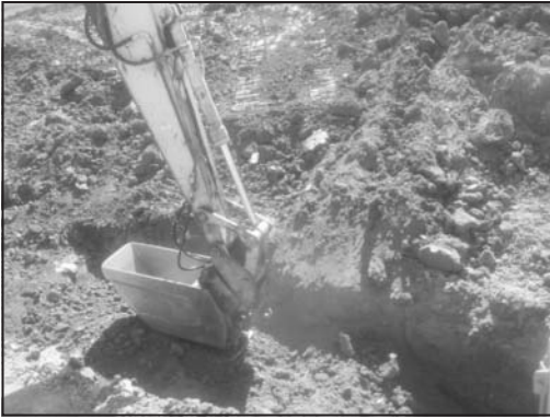
Figure 11. Compacting backfill with bucket plate compactor
