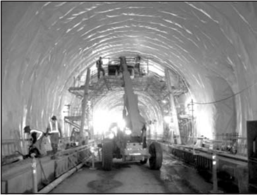
Figure 12. Staging waterproofing membrane on scaffolds
