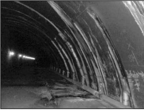
Figure 6. EJMT typical efflorescence and leakage showing drainage pipes in arch/radius wall
