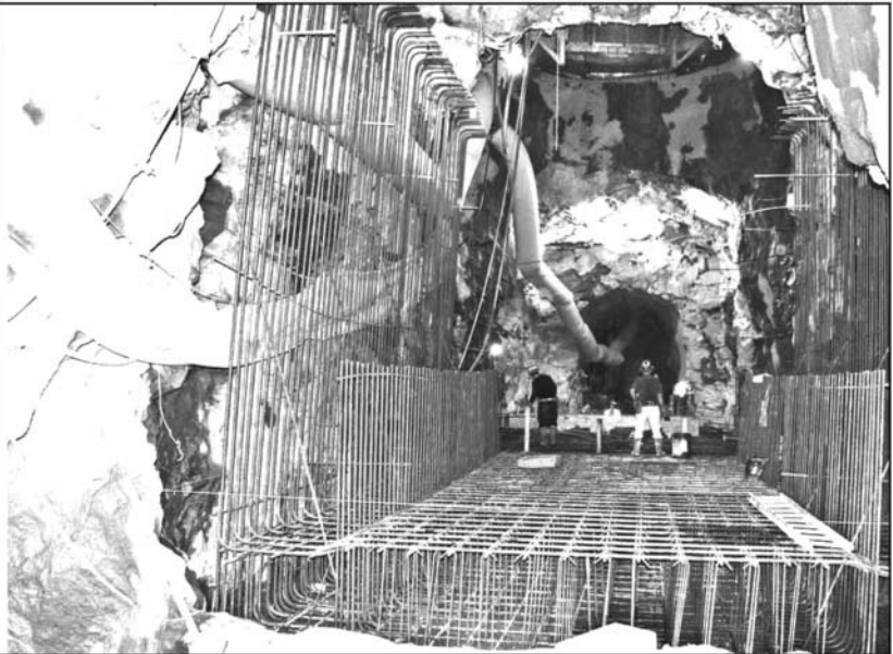
Figure 10. Photographic record of Contract No. 5 south connector tunnel
