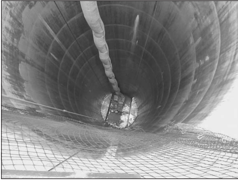
Figure 8. Preparatory work for ground freezing at the exit shaft
