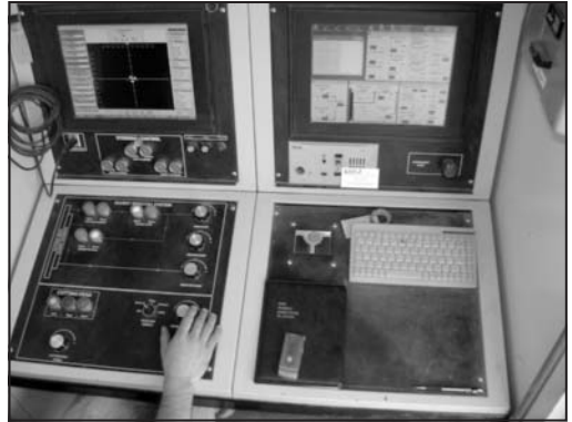
Figure 15. MTBM control panel
