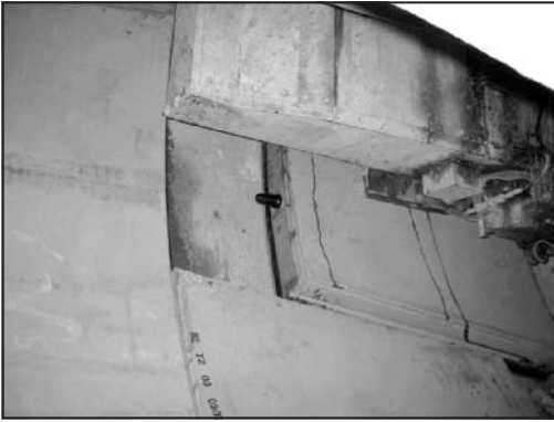
Figure 7. Segment installation with dowel system on circumferential joint
