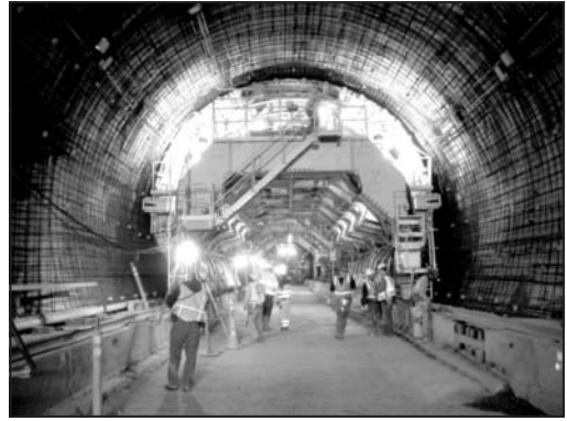
Figure 13. Final arch liner form set in the northbound tunnel
