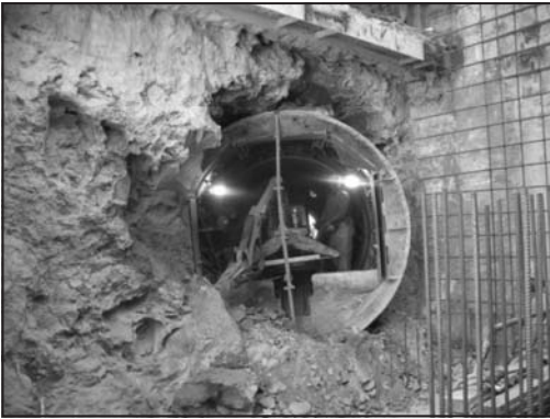
Figure 10. Tunnel shield breaking through the jet grouting at the diversion structure
