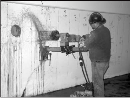
Figure 2. Pre-coring spiling holes from P2
