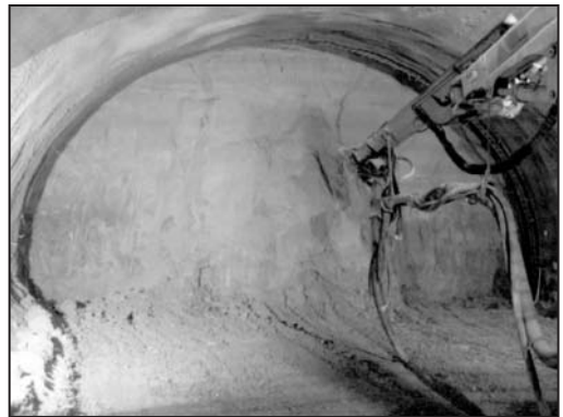
Figure 2. Tunnel face of the tunnel in loess clay
