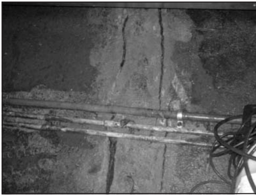
Figure 4. Existing cracks
