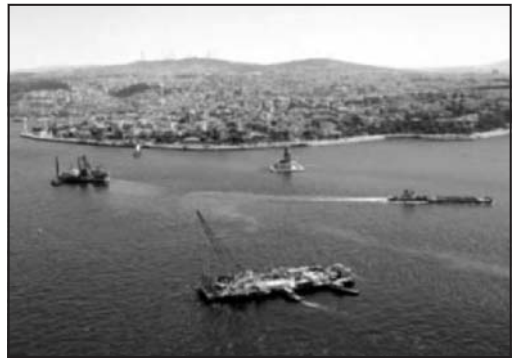
Photo 4. Work at the installation location on the sea (front: ground improvement, distance: dredging)
