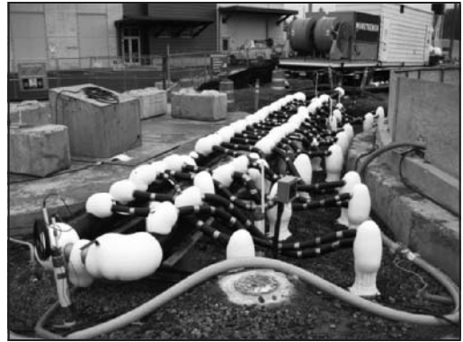
Figure 3. Activated freeze system
