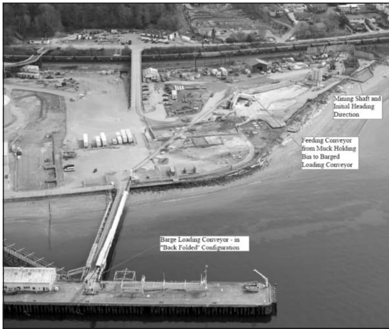
Figure 4. Photograph showing the overall layout of the main shaft location and muck handling system
