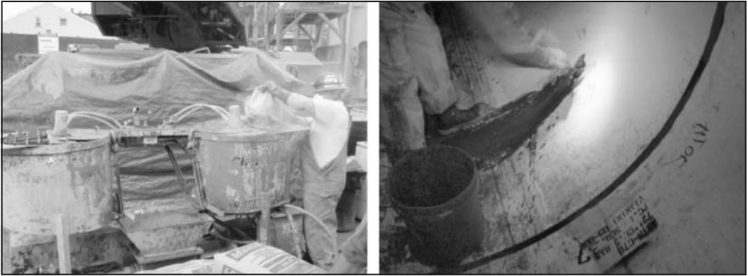
Figure 8. Contact grouting of the pipe: (a) batching; (b) verification
