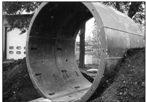
Figure 10. Polymer concrete segments
