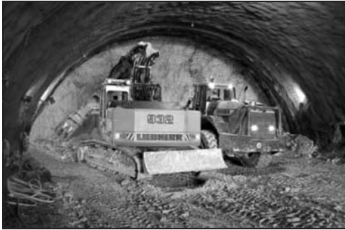
Photograph 1. LaserShell™ application with Multi Shot TunnelBeamer™
