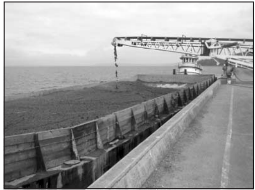
Figure 1. Photograph showing low angle belt conveyor and muck barge modified for fluid muck
