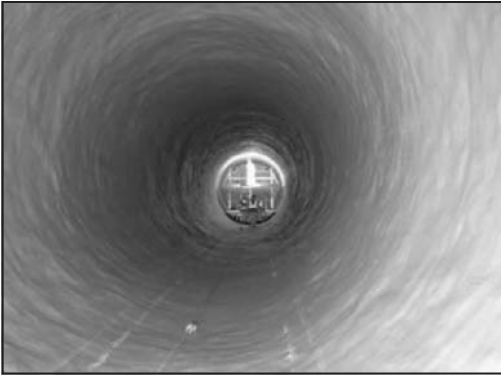
Photograph 5. Honor Oak (London, UK) water tunnel. Successful application on an uneven but closed surface.
