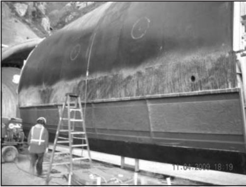
Figure 8. Textured panels attached to arch tunnel forms
