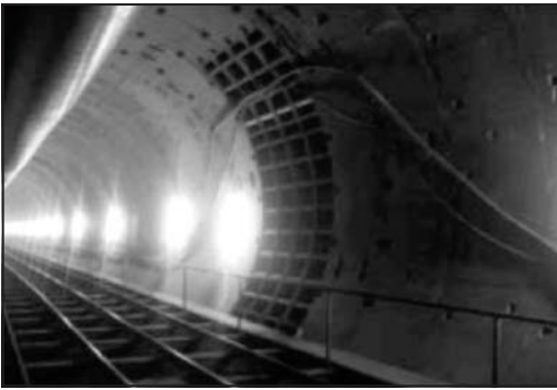
Photo 9. View of steel segments at completion of construction
