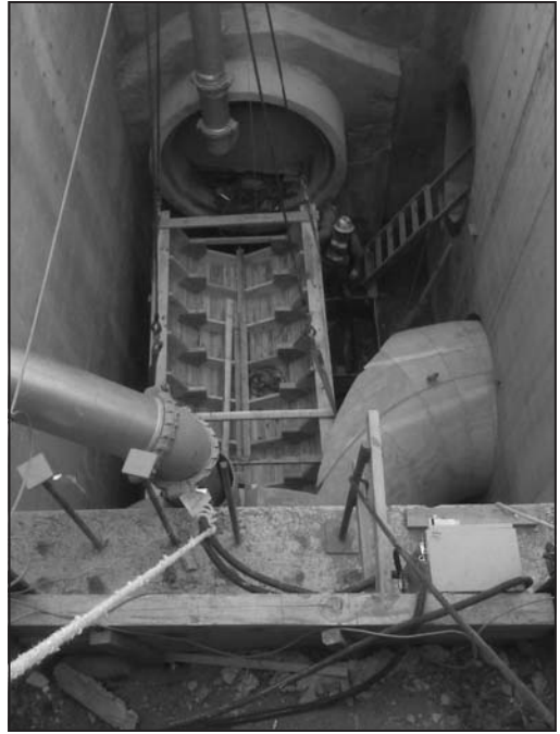
Figure 9. Flow-through pipe formwork
