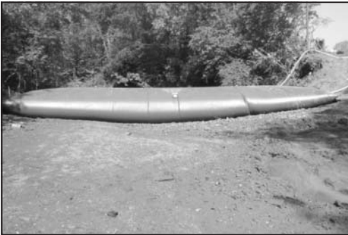
Figure 8. Portable dam inflated with water at Mill Creek crossing
