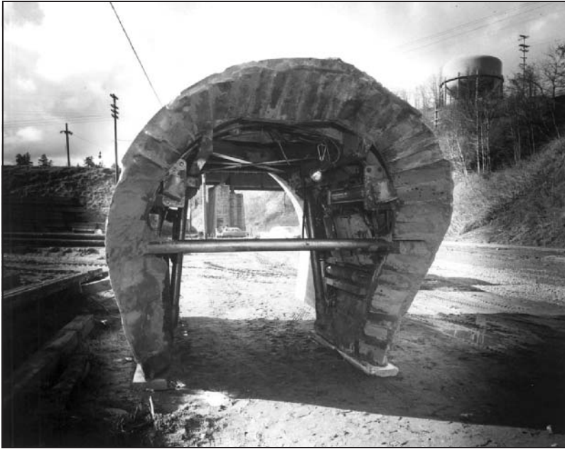
Figure 3. Front view of Portsmouth Tunnel open-face pneumatic shield with overhanging canopy (photo used with permission of the City of Portland Archives and Records)
