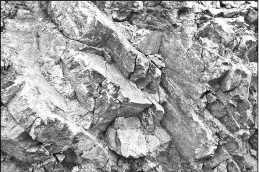
Figure 6. Photographic record of Contract No. 2 surface excavation
