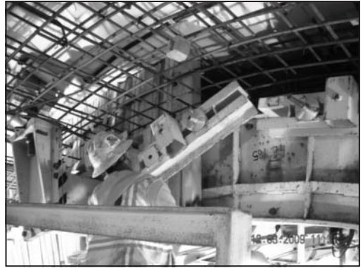
Figure 10. Fantail bulkhead braced by C-channel and coil rod
