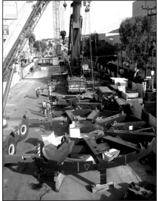
Figure 15. Assembling cutterhead sections with pedestal—Mexico MX12
