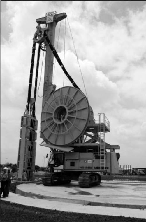
Figure 12. Hydro excavator machine, shaft 20
