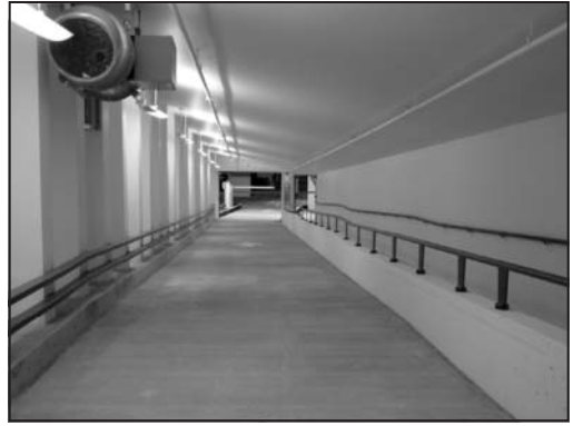
Figure 8. West side of completed tunnel
