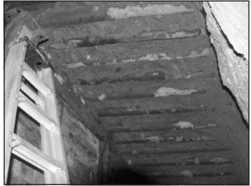
Figure 3. Exposed spiling inside tunnel portal
