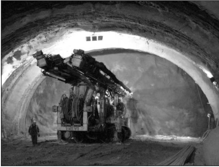
Figure 20. Soilmec SM 605 DT mobilized at tunnel face
