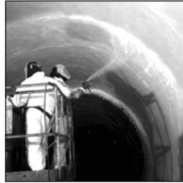
Photograph 8. Application of membrane—white second coat
