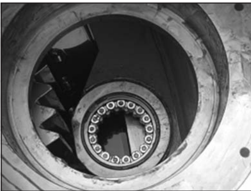
Figure 16. Installation of drive pinions—Mexico MX12
