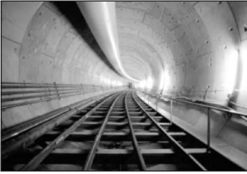
Photo 8. View of RC segments at completion of construction
