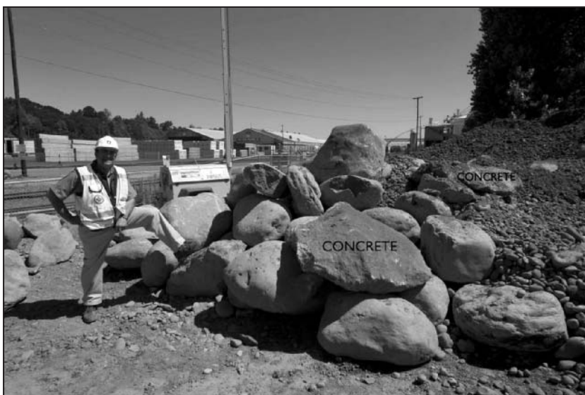
Figure 5. Catastrophic glacial flood boulders encountered within the Swan Island Pump Station shaft excavation (photograph by Sue Bednarz, Jacobs Associates)
