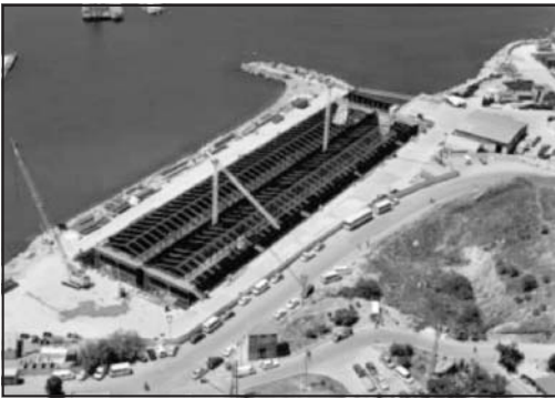
Photo 2. Element construction in temporary dry dock
