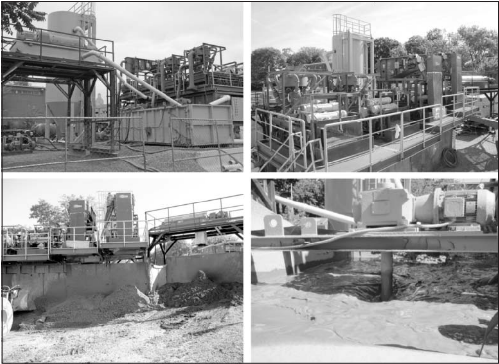
Figure 4. Slurry processing system
