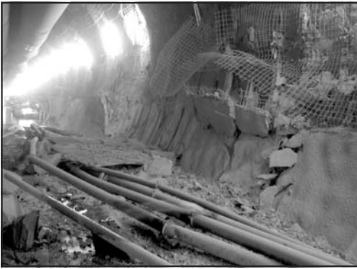
Figure 7. Single-track tube east/north. Left: damage of the support's shotcrete. Right: invert heaves.
