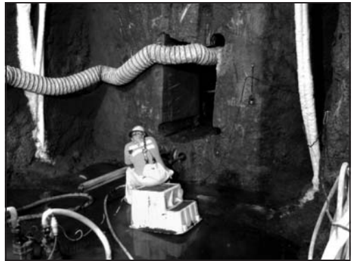
Figure 9. Access panel to the active Confluent Shaft to check for water presence
