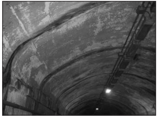
Figure 5. Icicles forming at deteriorated tunnel joints
