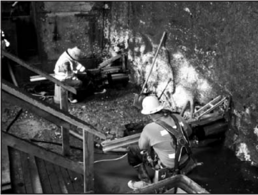
Figure 5. Coring in preparation for wire saw cutting
