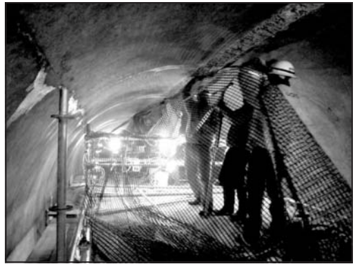
Figure 5. Installation of base layers
