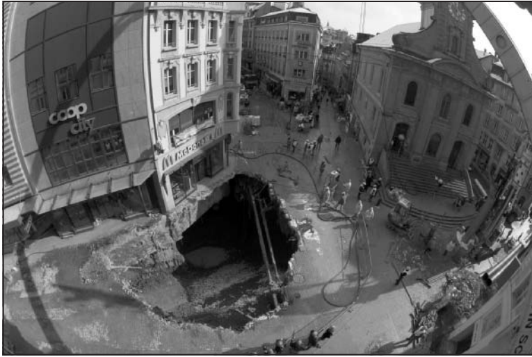
Figure 21. Sinkhole at Placa St-Laurent above Saint Laurent tunnel in Lausanne, Switzerland
