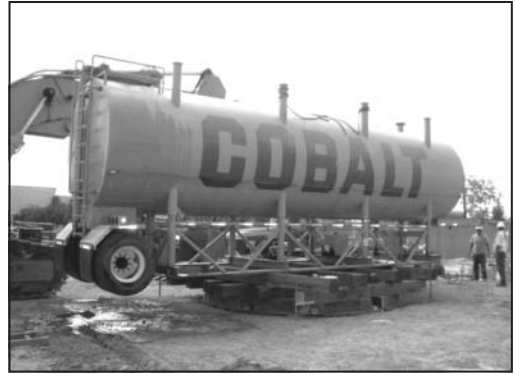
Figure 5. Load testing of two-ring small-diameter shaft (July 2008); filled water tanker resting on a timber mat on top of the shaft, weight of 54,000 kg (60 ton)
