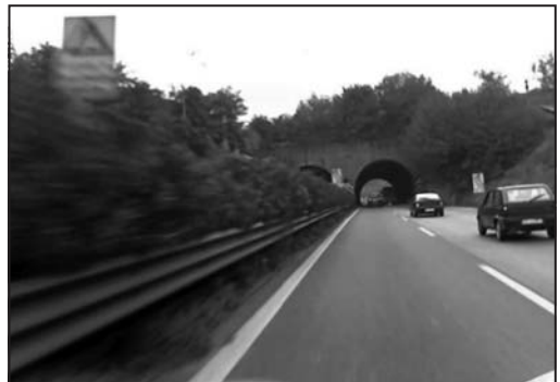
Figure 1. Driving along the old inner bore of Cassia tunnels
