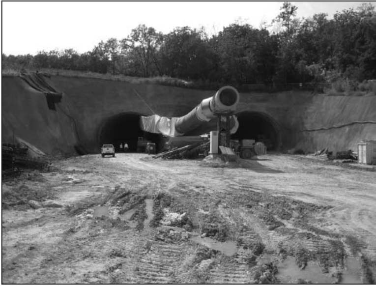
Figure 1. Tunnel portal Tunnel A
