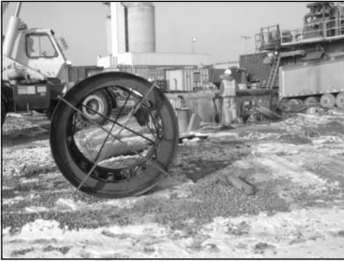
Figure 17. Intermediate jacking station
