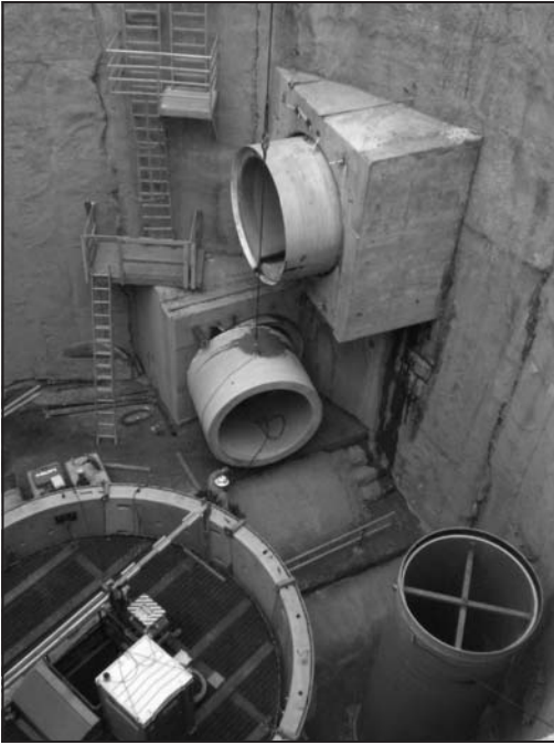
Figure 4. Stacking of OF36 and OF37 pipelines in Alder shaft
