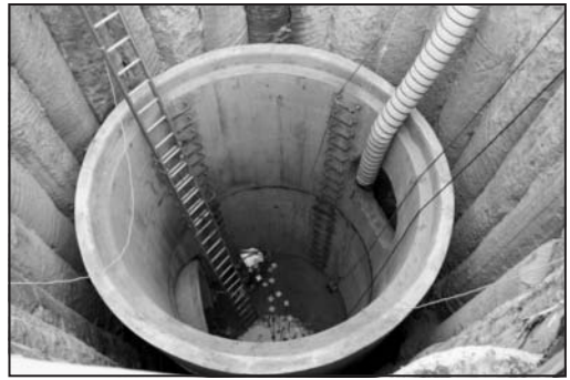
Figure 7. OF38 precast concrete diversion structure
