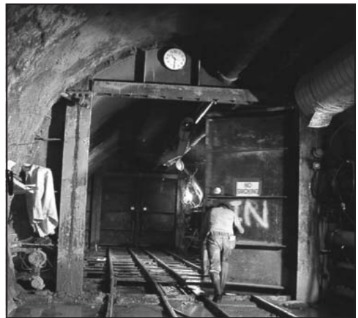
Figure 10. Air lock at Orme Street III sewer project (Atlanta, Georgia)
