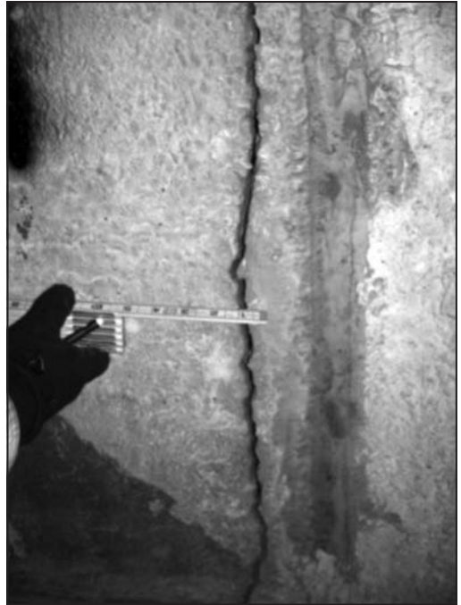
Figure 7. Crack in pre-cast panel, adjacent to neoprene construction joint, in EJMT
