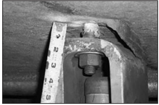
Figure 2. Condition of an anchor found after inspection. Central Artery Tunnel, Boston, MA
