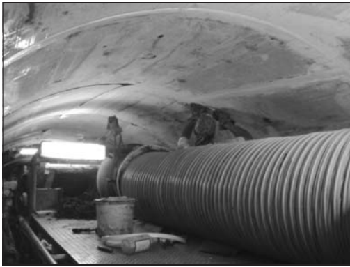
Figure 3. Work area with fresh air duct
