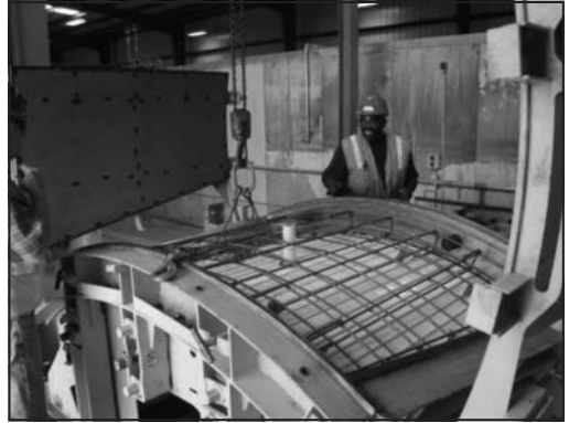
Figure 4. Placement of steel reinforcement cage
