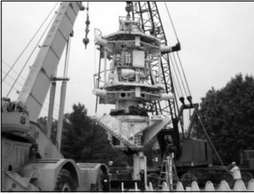
Figure 7. Vertical boring machine (VBM) designed by The Kassouf Company, utilized for shaft excavation through shale
