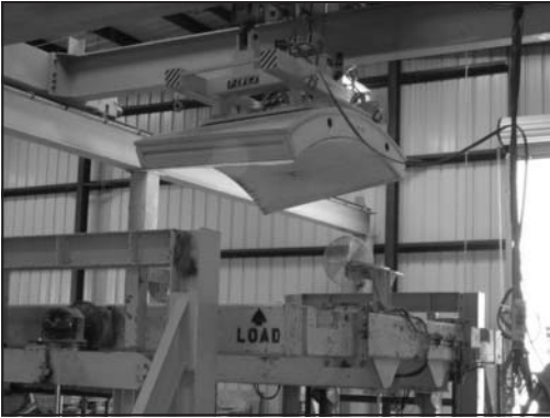
Figure 5. Demolding of segments from forms
