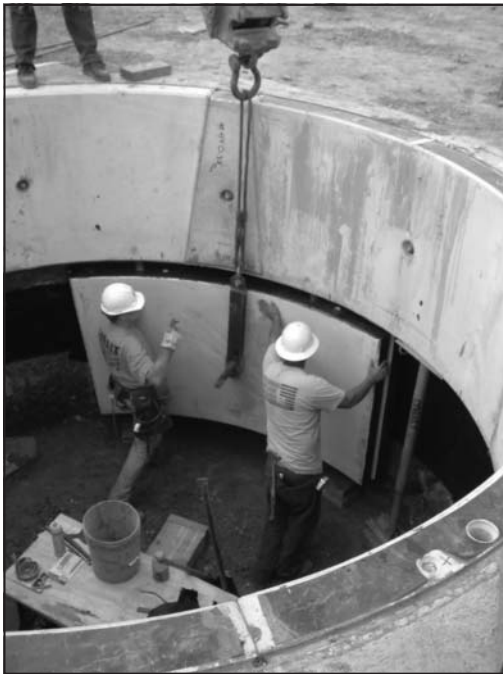
Figure 1. Underpinning with second ring of segments
