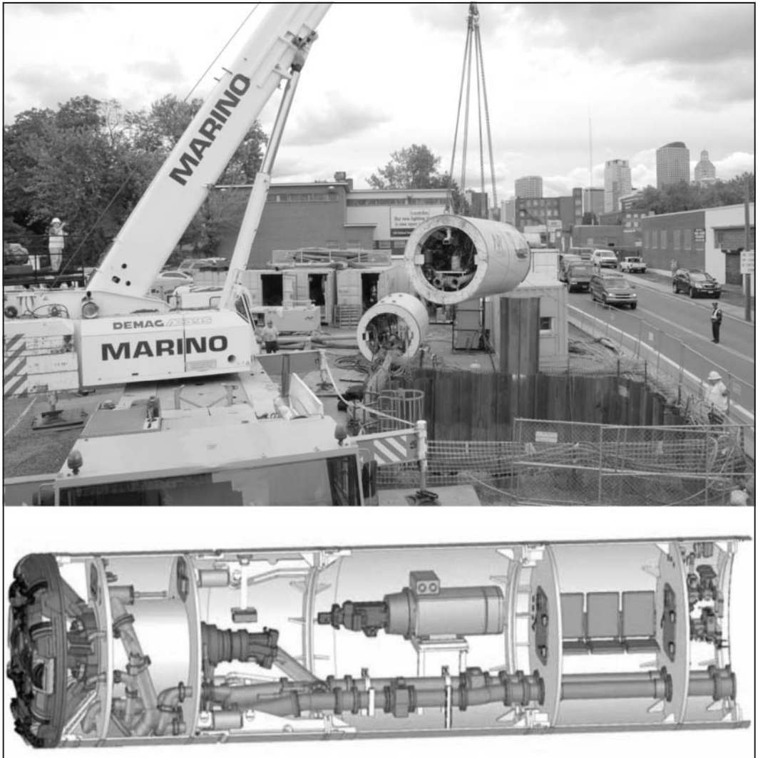
Figure 5. a. Slurry machine being lowered into jacking shaft; b. schematic (Herrenknecht)
