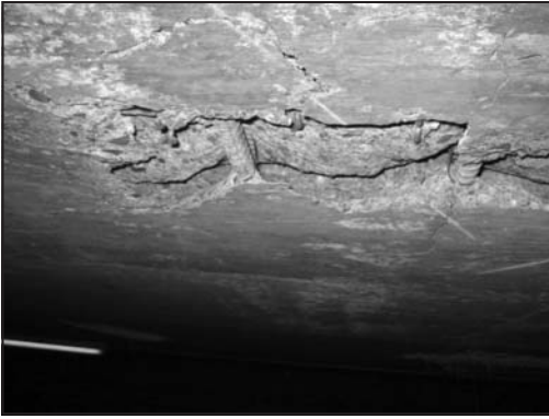
Figure 4. Crack on tunnel roof. Hanging Lake Tunnel, I-70, Colorado
