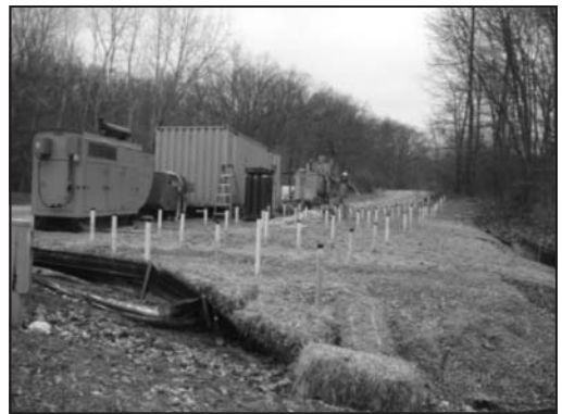
Figure 5. Permeation grouting setup
