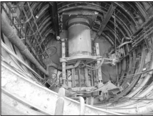
Figure 18. Jacking RCP pipe and advancing the MTBM
