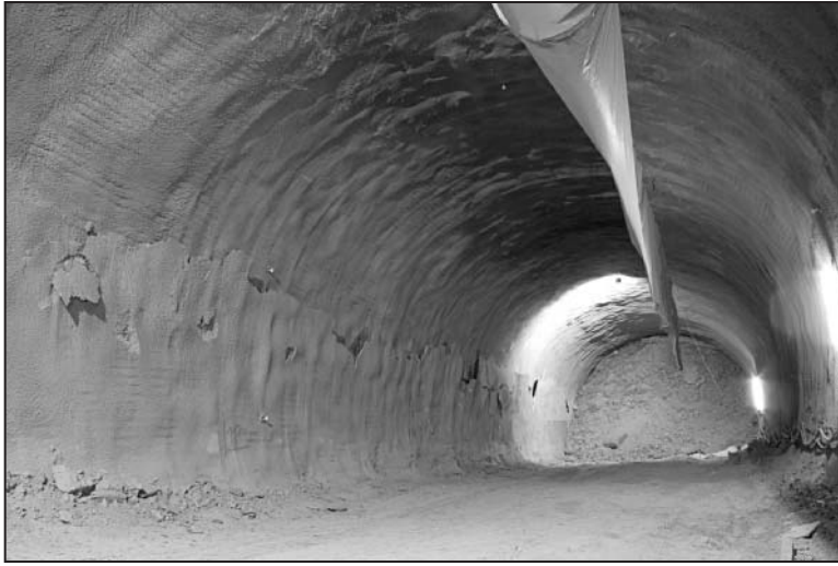
Figure 3. Cracks in the shotcrete lining between the first and second collapse
