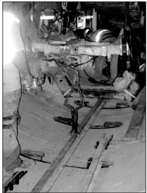
Figure 10. Track laying process
