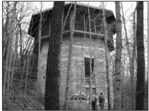
Figure 9. Exterior view of ventilation structure atop West Rock Ridge
