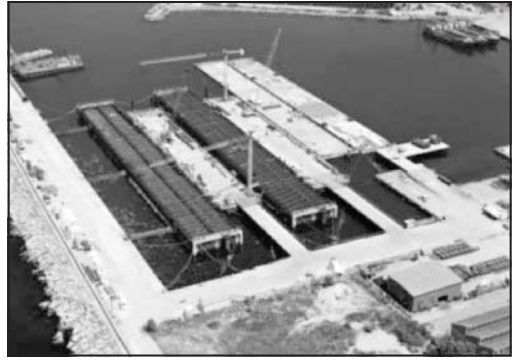
Photo 3. Element construction at marine mooring facility
