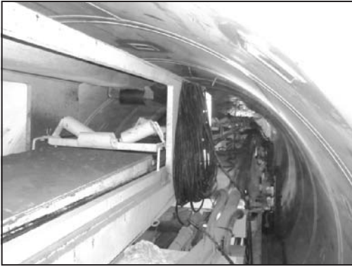
Figure 13. Rear PVC welding station and continuous conveyor tailpiece
