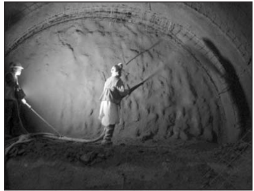
Figure 7. Shotcrete application at face
