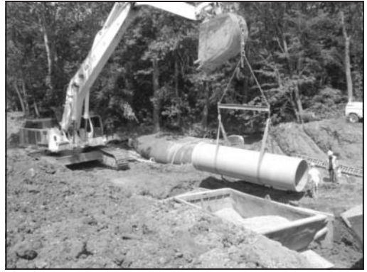
Figure 9. Installing pipe at Mill Creek crossing
