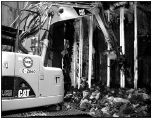
Figure 7. Excavation of frozen soil
