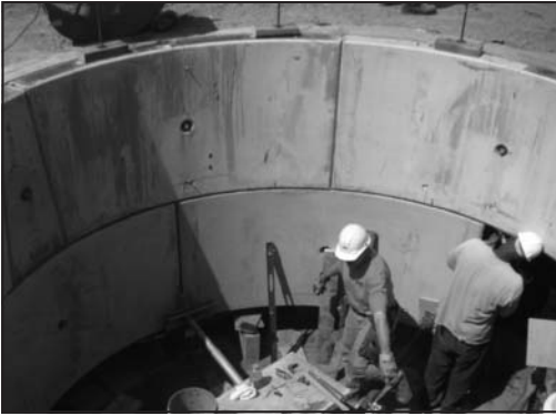
Figure 4. Construction of small-diameter shaft (July 2008)
