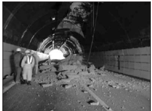
Figure 9. Highway tunnel lining falling from tunnel crown: 2004 Niigata earthquake, Japan
