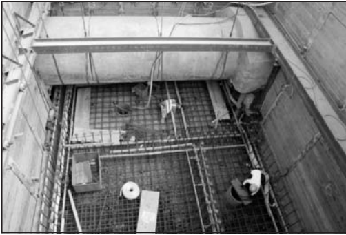
Figure 8. OF46 diversion pipe base slab layout
