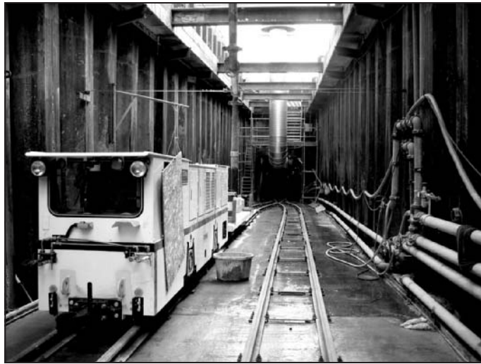
Figure 4. Double tracks in the start shaft
