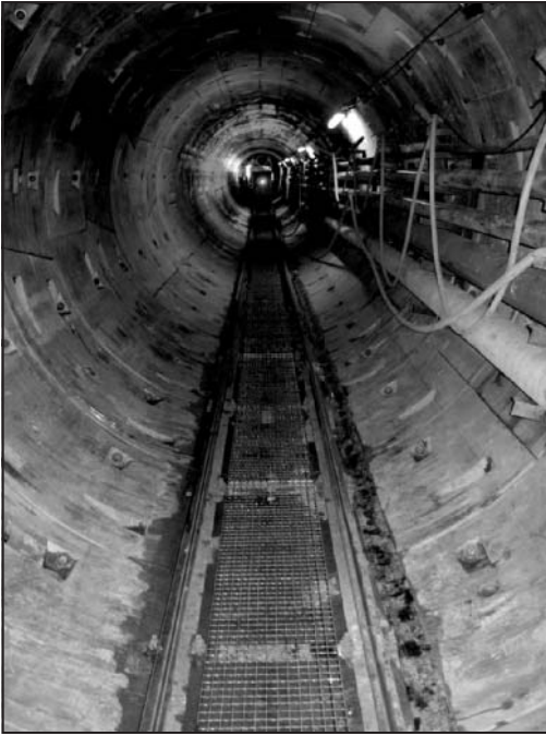
Figure 6. Inside view of tunnel
