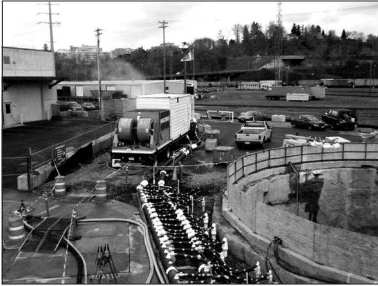
Figure 2. Freeze plant set-up
