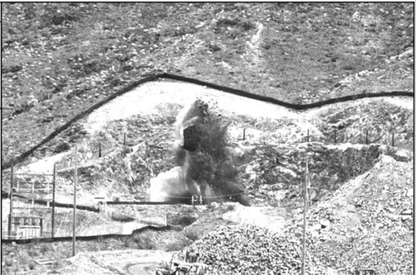
Figure 7. Photographic record of Contract No. 2 surge shaft
