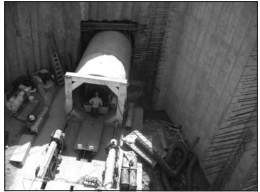
Figure 11. Pushing of the RCP into the completed tunnel
