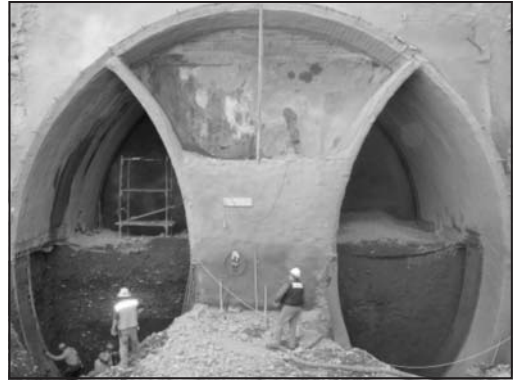
Figure 17. Typical excavation sequence for Santiago's La Cisterna station
