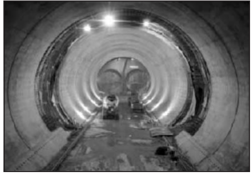
Photo 12. View of crossover tunnel lining
