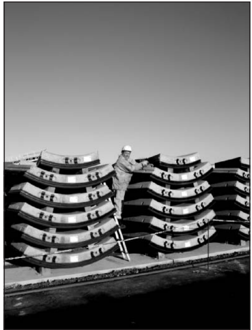
Figure 5. Precast concrete segments
