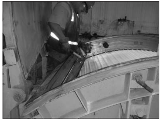
Figure 4. Placement of PVC T-Lock ® liner in form
