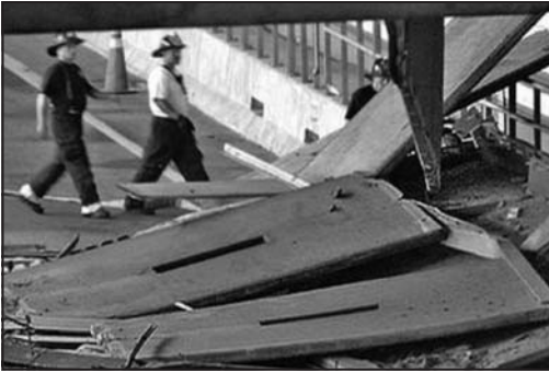
Figure 1. Suspended ceiling collapse in the Central Artery Tunnel, Boston, MA
