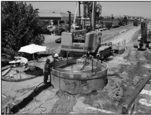
Figure 3. Blind auger drilling for manhole construction
