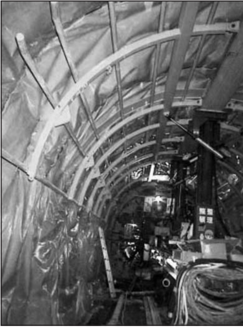
Figure 11. HDPE Agrisuregrip lining being installed
