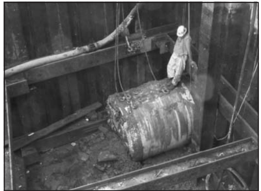
Figure 10. Photo showing MTBM breaking through the receiving shaft
