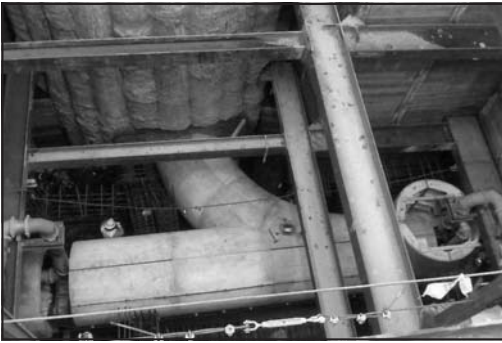
Figure 6. OF28 “Y” diversion structure
