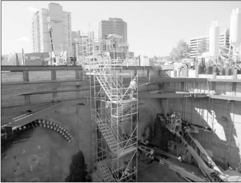
Figure 5. View of NATM tunnel east portal in relation to high-rise buildings near the alignment
