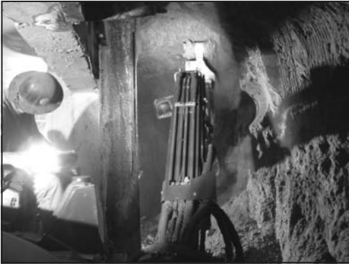
Figure 7. Boom mounted NDCO used during portal development
