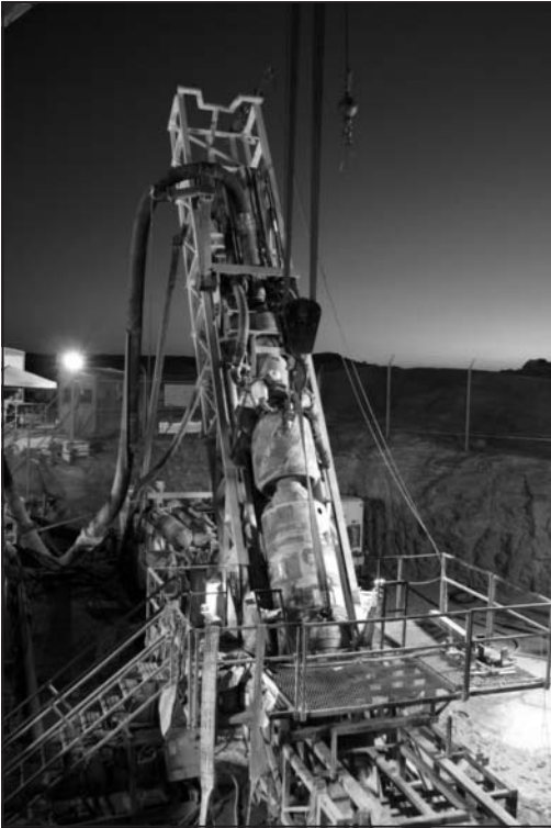
Figure 3. The RD-20 drill rig during drilling of the new 43-inch diameter inclined shafts
