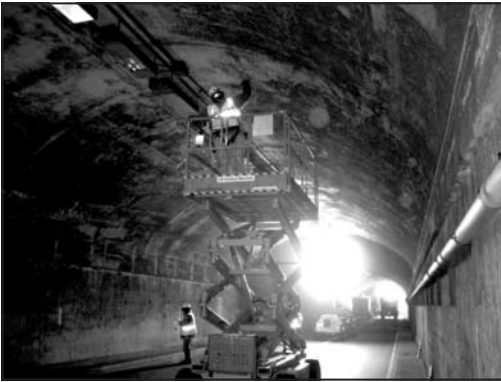
Figure 7. Crews performing structural hands-on and visual inspection
