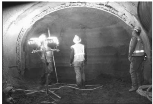
Figure 7. Photograph of typical tunnel excavation showing freshly exposed massive sedimentary bedrock, widely spaced joints, a lattice girder, and a flash-coat of shotcrete
