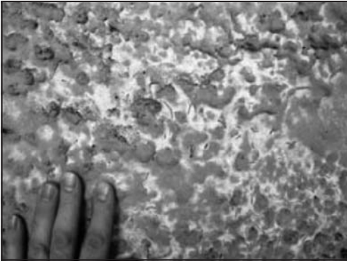
Photograph 3. “Mud cracking,” pinholes, and uneven coverage of a one coat water based sprayed membrane, applied over “as shot” shotcrete
