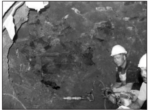
Figure 6. Photo of hand-mined tunnel face
