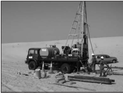
Figure 4. Drilling for a T-03 borehole
