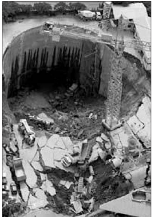
Figure 20. Collapsed Capri shaft in Sao Paulo, Brazil
