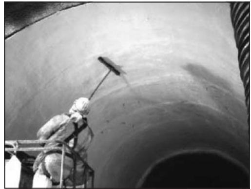
Photograph 9. Integrity testing in a SCL tunnel
