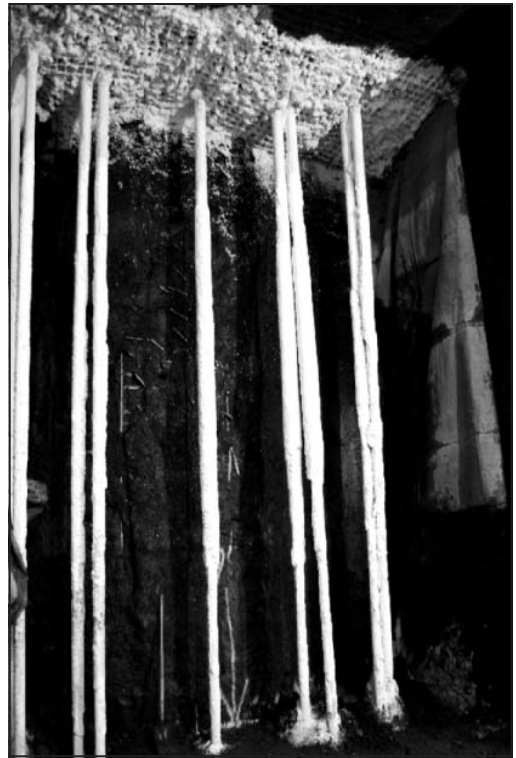
Figure 8. Exposed pipes showing insulation above and shotcrete on walls
