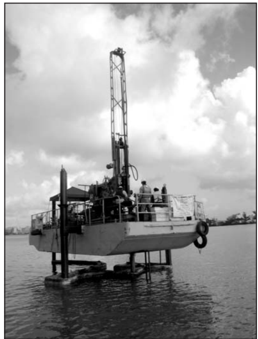
Figure 4. Water boring investigation from a barge for the Port of Miami Tunnel, Miami, FL
