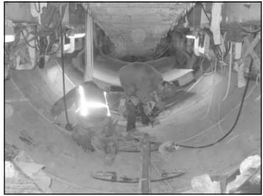
Figure 4. Heat welding of seams
