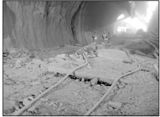
Figure 7. Single-track tube east/north. Left: damage of the support's shotcrete. Right: invert heaves.
