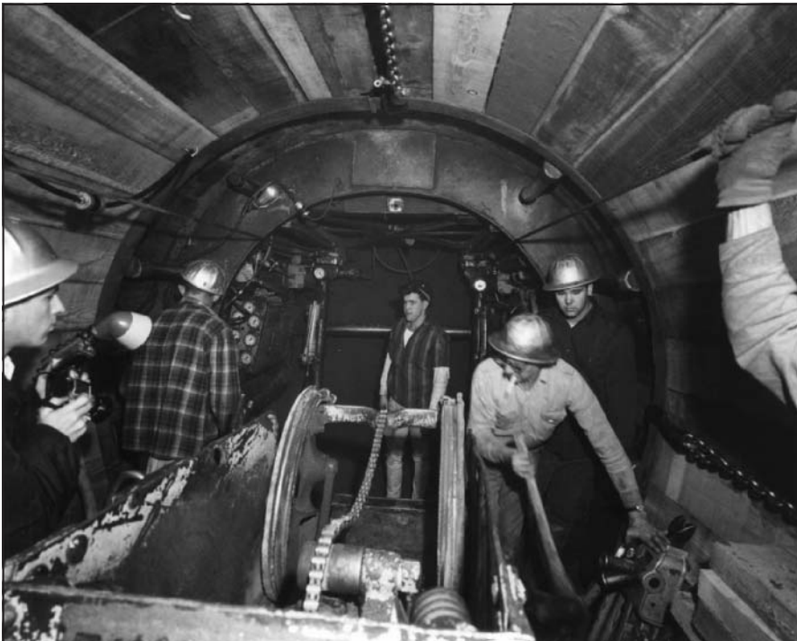
Figure 4. Workers inside the Portsmouth Tunnel shield during tunnel excavation (photo used with permission of the City of Portland Archives and Records)
