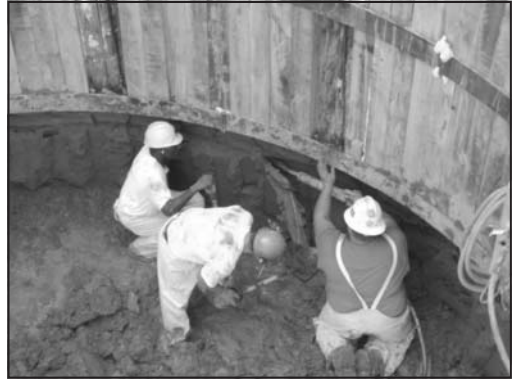
Figure 14. Shaft excavation by hand with pneumatic shovels
