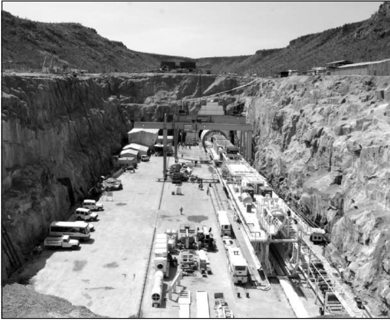
Figure 7. Assembly proceeding in the granite open cut
