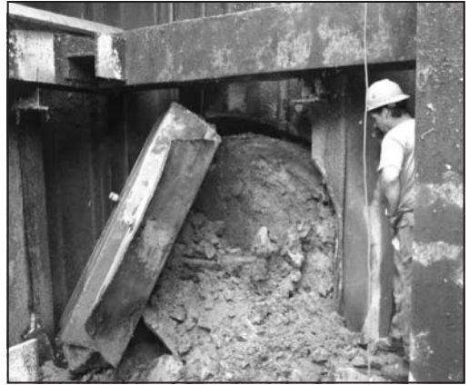
Figure 9. Tunnel shield breaking through the jet grouting at the diversion structure
