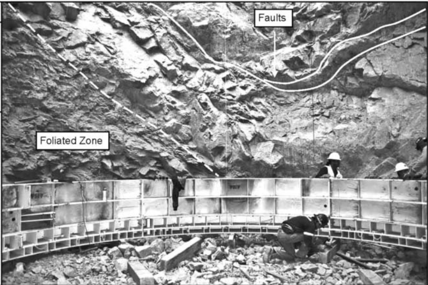
Figure 8. Photographic record of Contract No. 2 surge shaft
