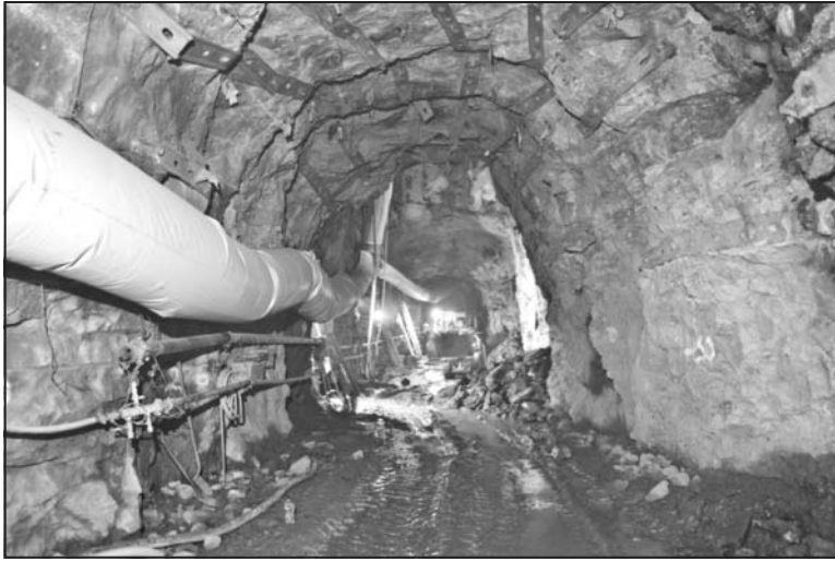
Figure 1. Photo of Southern Nevada Water Authority Contract No. 5 connector tunnel
