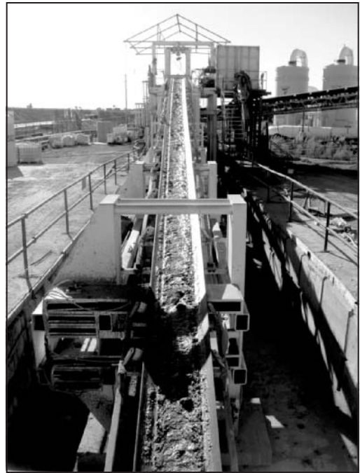
Figure 4. Surface setup conveying muck
