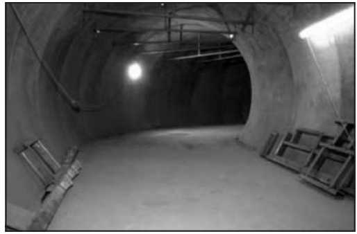
Photograph 2. Finished LaserShell™ SCL in Heathrow T5 underground works
