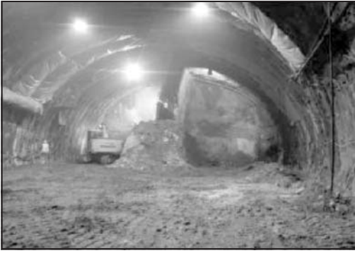
Photo 11. View of excavation of the crossover tunnel
