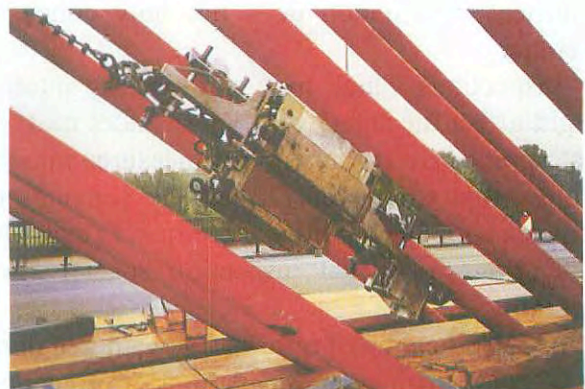
Fig. 2-17: Tendon anchorage after removal of sheath, (Vollrath, Tathoff 1990, [152])
