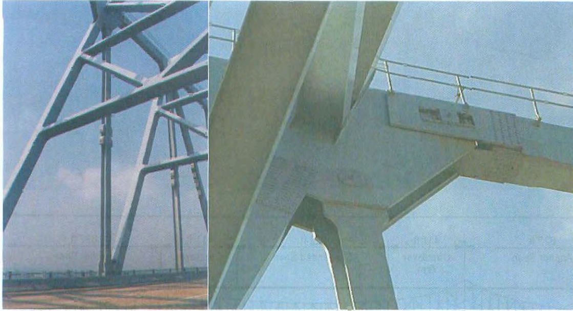
Fig. 11-54: View of truss elements including a closeup view of a pin-and-hanger
