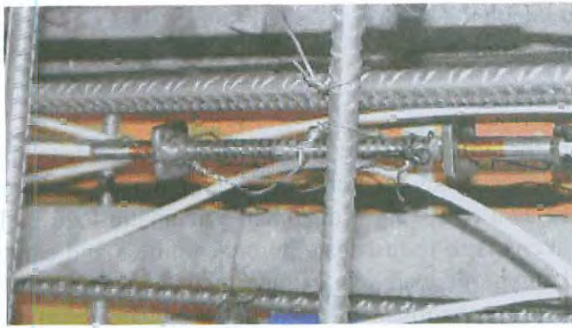
Fig. 5-30: Placement of a FBG-Sensor
