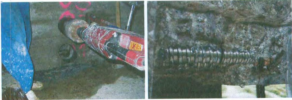
Fig. 11-48: Cutting of prestressing tendons
