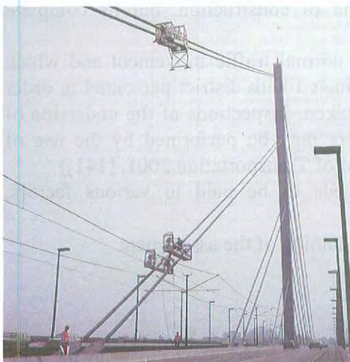
Fig. 2-18: Bridge inspection, (Vollrath, Tathoff 1990, [152])
