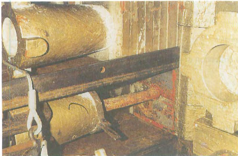
Fig. 2-17: Tendon anchorage after removal of sheath, (Vollrath, Tathoff 1990, [152])
