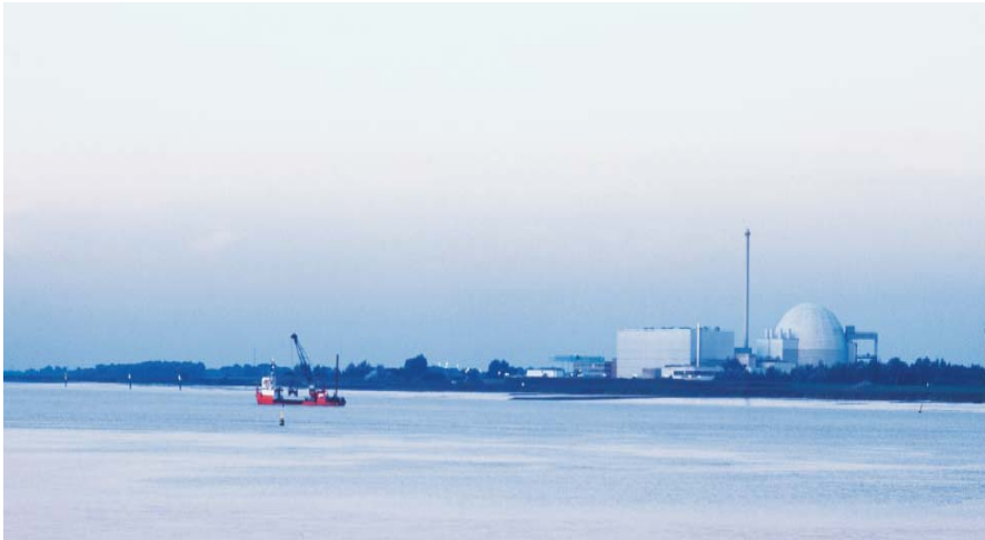
Fig. 1: Unterweser nuclear power station
