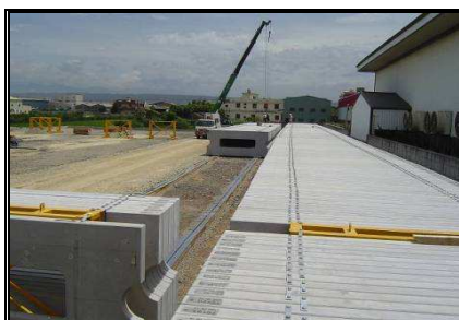
Fig. 7 Slab storage area
