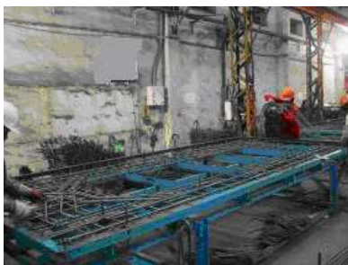
Fig. 4 Platform for steel cage
