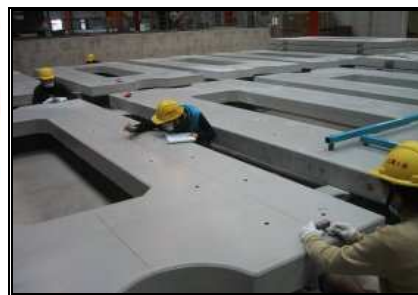
Fig. 5 Check of slab tracks
