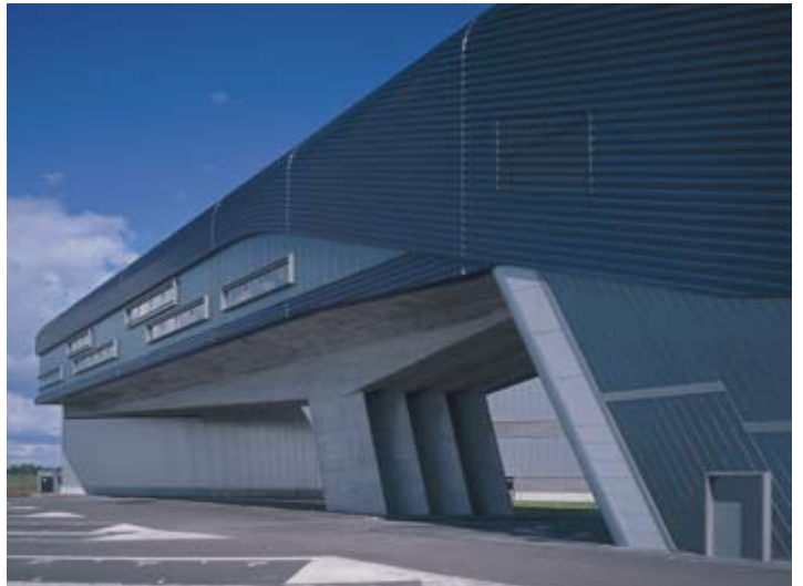
TOP: View of entry canopy under construction BOTTOM: View of completed entry canopy
