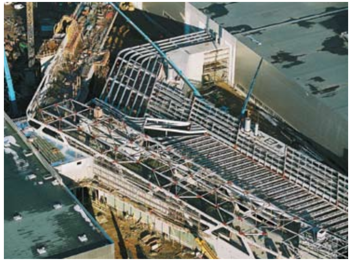
Roof framing under construction
