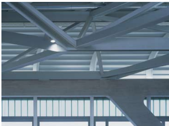
LEFT: Interior view with space frame
