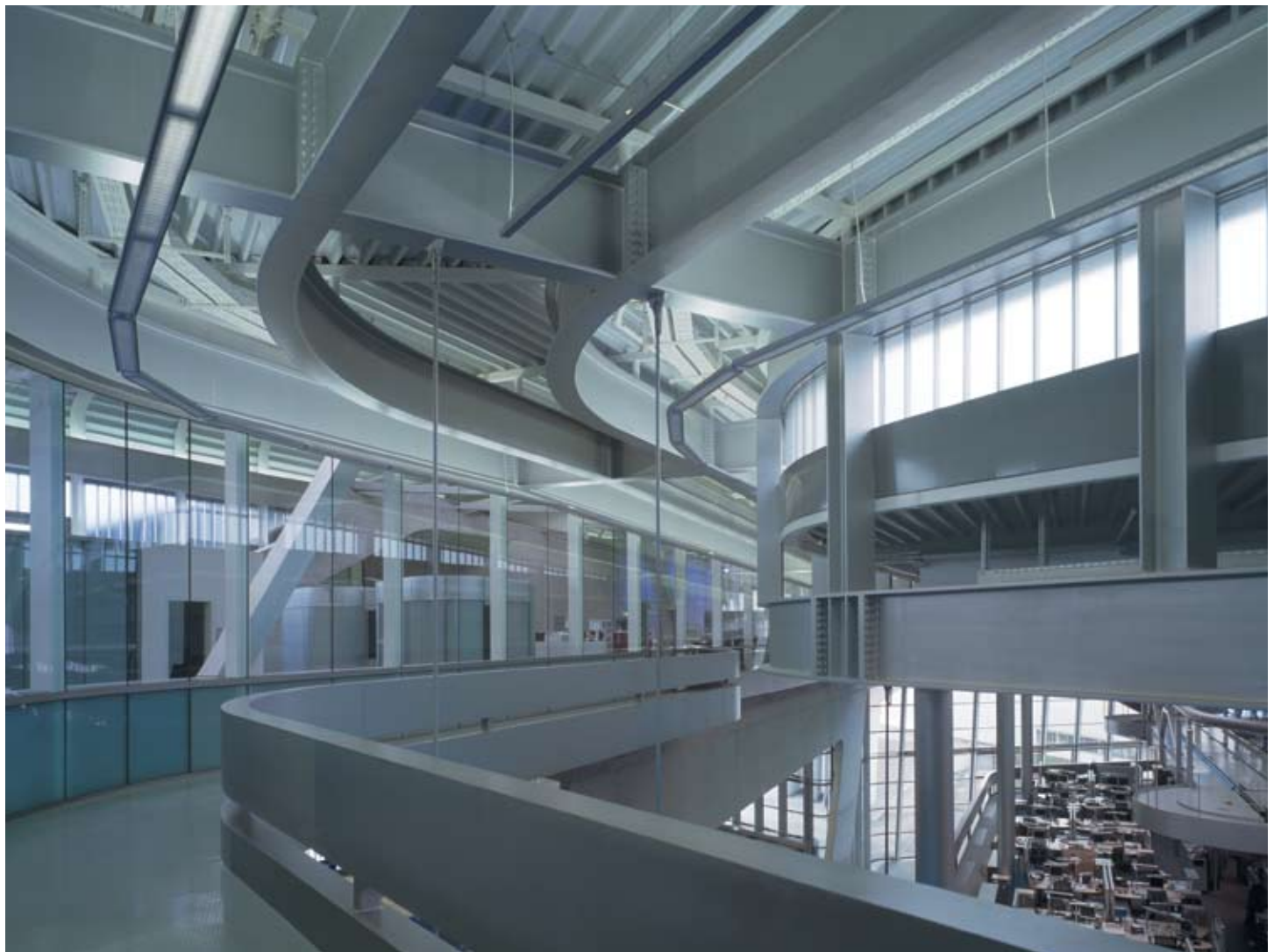
Completed roof framing
