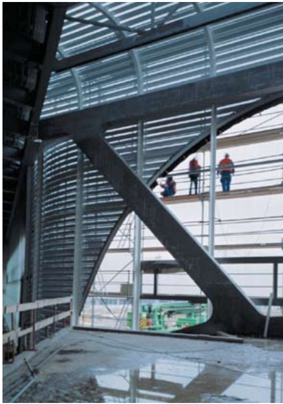
LEFT: Cladding installation
