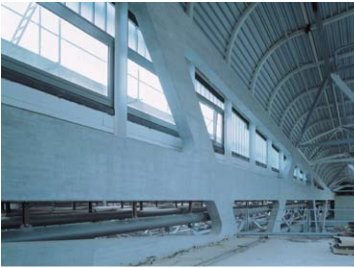
TOP: Concrete walls under construction
