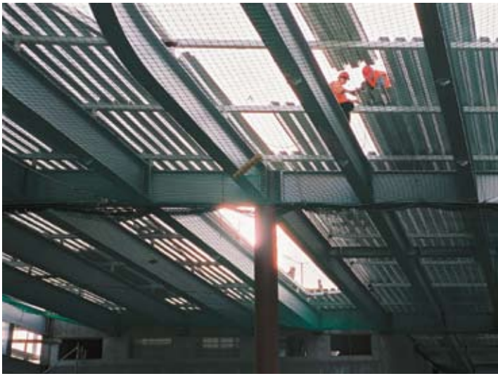
TOP: Installation of roof deck BOTTOM: Aerial view of central building
