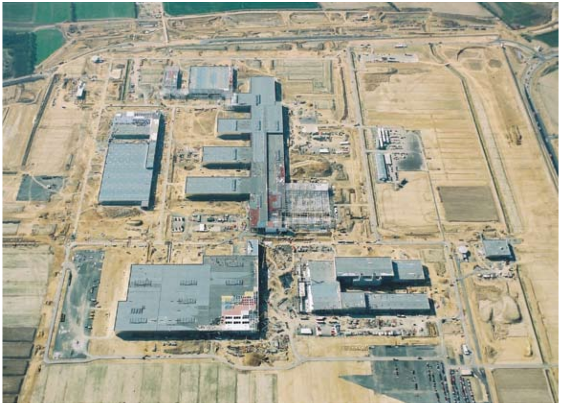
Aerial view of plant under construction
