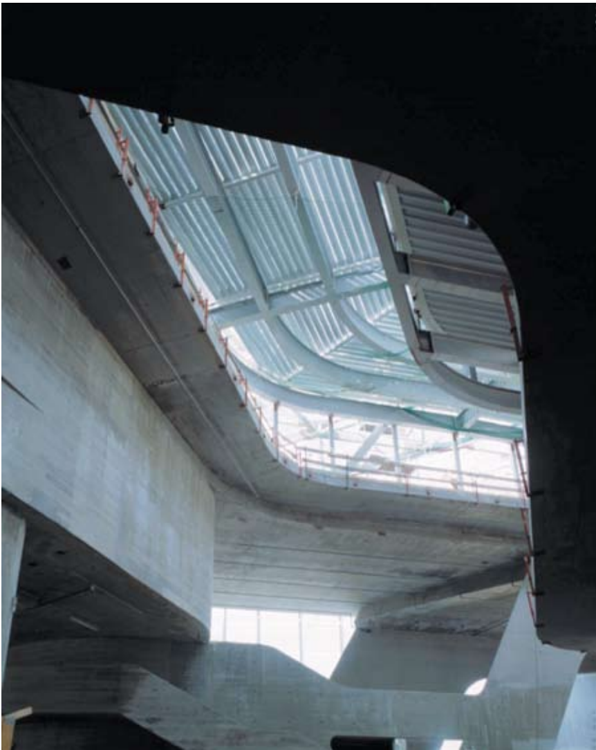
Interior construction view with roof framing
