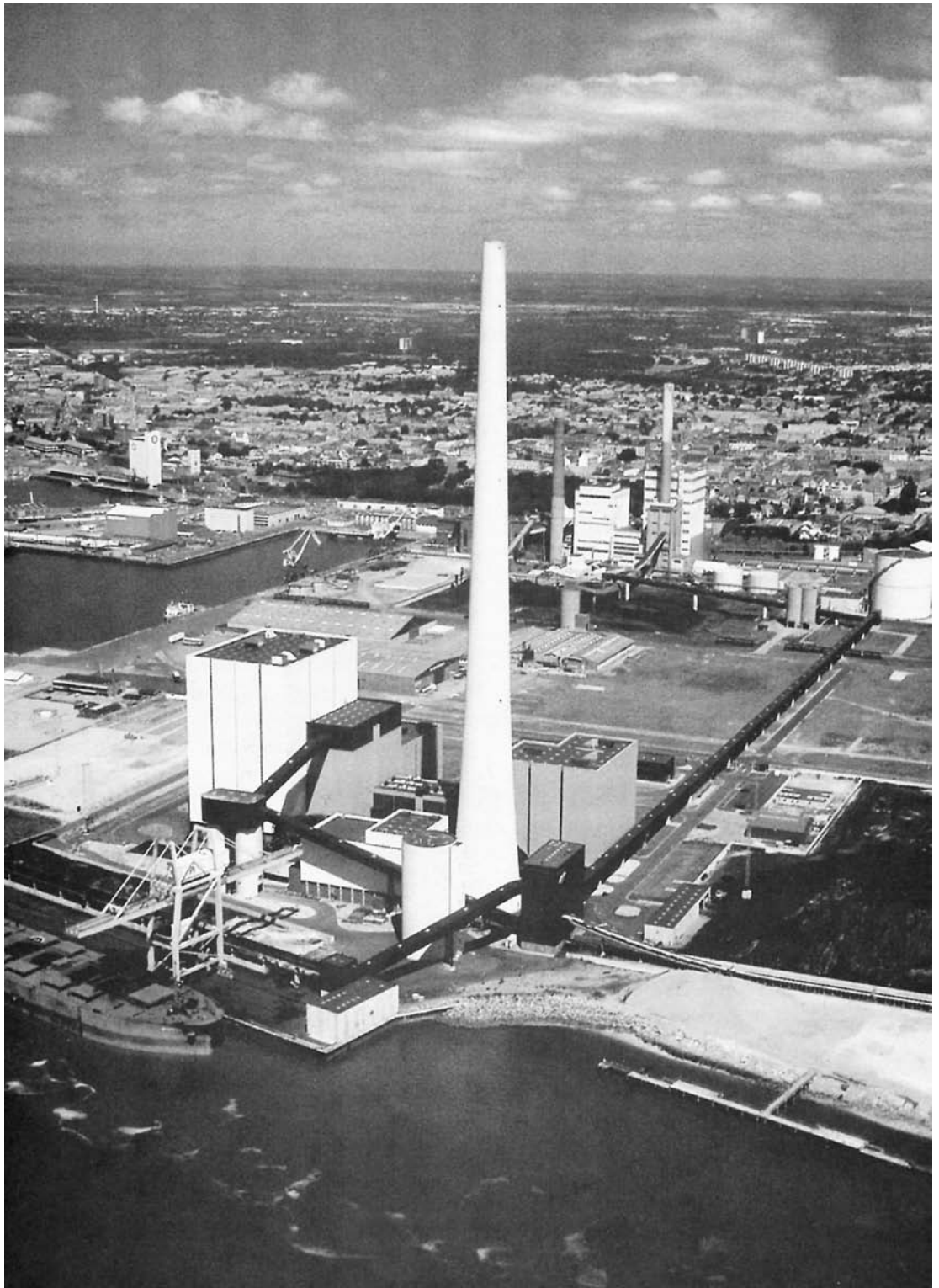
FIGURE 1.2 The Esbjerg, Denmark, power station. (Courtesy Vestkraft 1996.)
