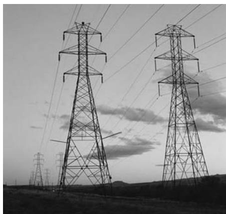
FIGURE 4.26 Electrical power transmission tower and line.
