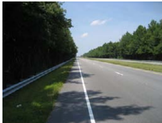
Figure 5. A Site view of NC 11 southbound
