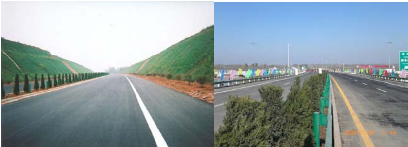
Fig. 7 The 26.78 km long Da'an to Jilao expressway long-life flexible pavement was completed and opened at the end of November 2008
