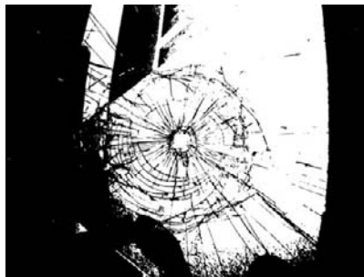
Fig. 2 The glass rupture image after processing
