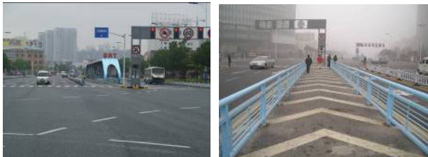
Figure 7. Passenger Access of Changzhou BRT
