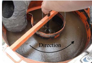
Fig. 7. Exhaust and grouting funnel
