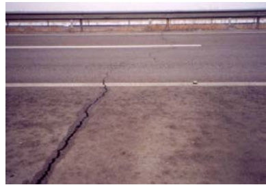
Fig. 1 Cracking of relatively new semi-rigid asphalt pavement in Hohhot, Inner Mongolia, transverse thermal crack with top down cracking in wheel path
