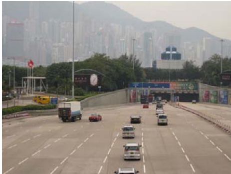
Figure 9. Enhancement of traffic control management at toll plaza and tunnel entrance
