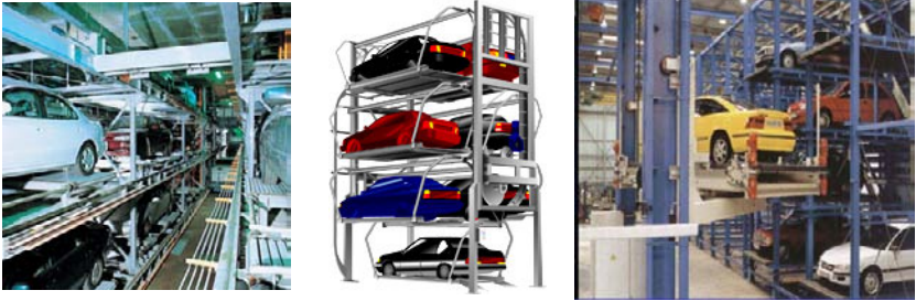
Figure 8. Mechanical parking facilities
