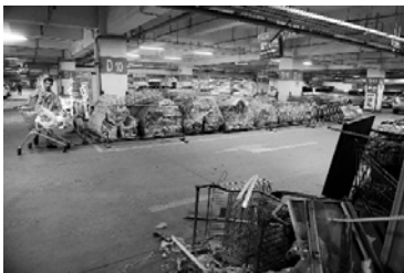
Figure 4. Abused use of parking spaces
