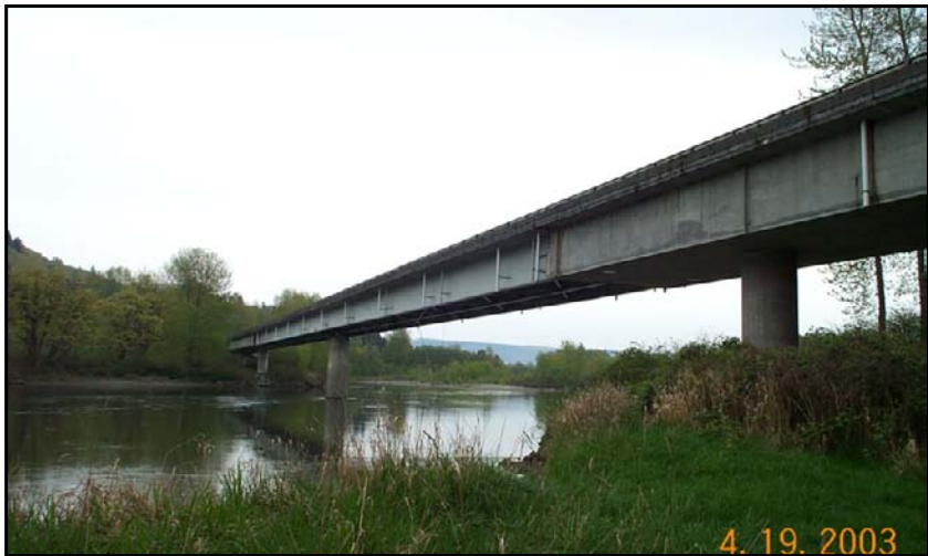
Figure 1 Existing Snohomish River Bridge
