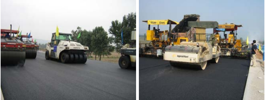
Fig. 6 Asphalt paving in summer 2008
