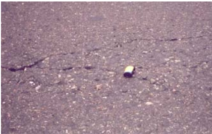
Fig. 1 Cracking of relatively new semi-rigid asphalt pavement in Hohhot, Inner Mongolia, transverse thermal crack with top down cracking in wheel path
