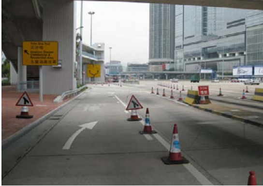
Figure 8. Erection of temporary traffic signs
