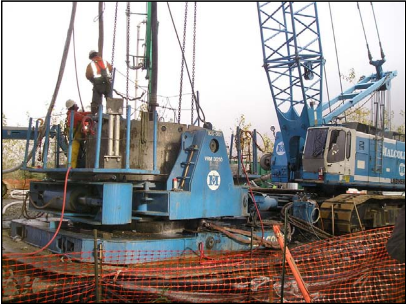
Figure 8 Oscillator was setup for the drilled shaft constructions
