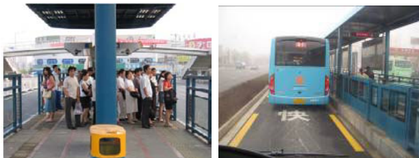
Figure 2. Automatic platform doors in Beijing and Changzhou BRT
