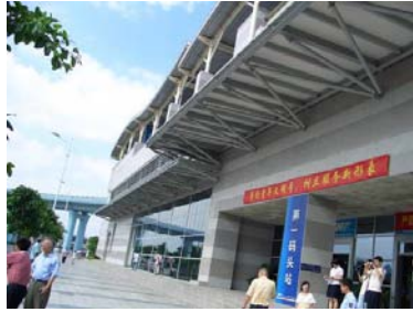
Figure 3. Xiamen BRT Station
