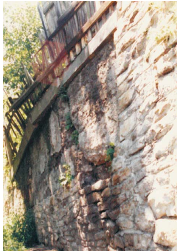
Fig. 45.4. Earth pressure on a retaining wall
