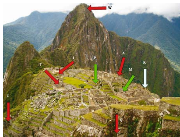
Fig. 4.1. Photo of Machu Picchu archaeological site with localization of dilatometric measurements. C: Cave (measuring site C1); T: Principal Temple (T1, T2, T3); I: Intiwatana (I1, I2, I3); P: Plaza (P1); W: Huayna Picchu (W1, W2, W3); A: Acllawasi (A1); M: Wairana o Mirador (M1, M2, M3, M4); R: Rodadero (R1, R2, R3); Q: Qhata (Q1). Qualitative evaluation of trends of movements. Red color: irreversible movements; green color: without any irreversible movements; light blue: cannot be still interpreted
