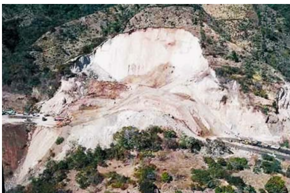
Fig. 41.3. The Pan America Highway in El Salvador was badly damaged by a landslide during the January 2001 earthquake
