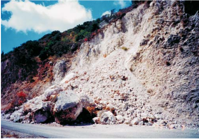
Fig. 37.5. Rock falls occurring in the highly fractured (mylonitized) and weathered zone of limestones, triggered by strong earthquake, in Lefkada Island (August 2003)
