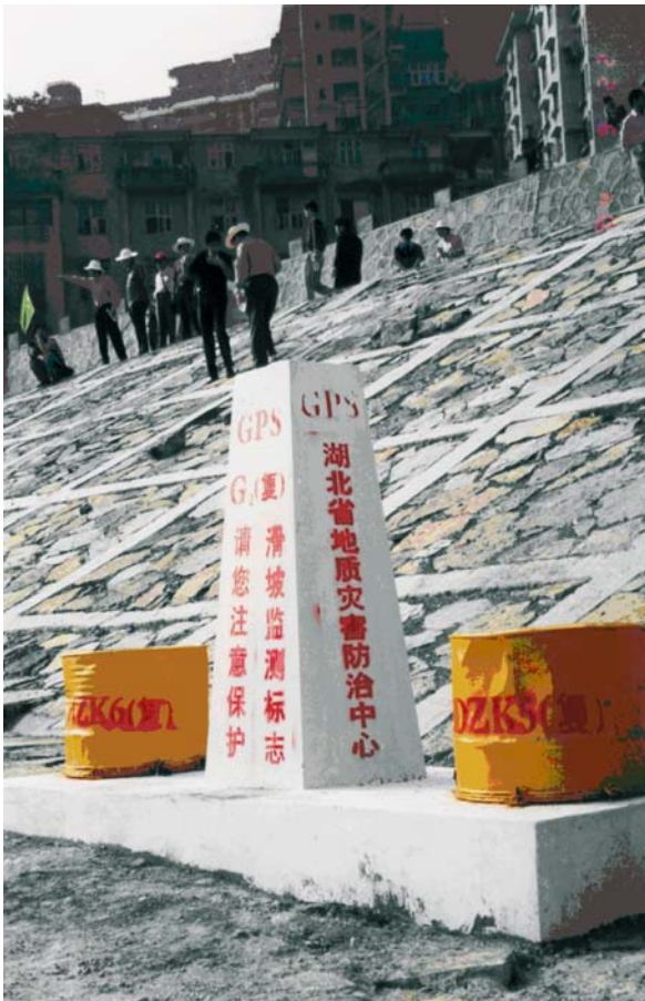
Fig. 36.9. GPS monitoring for the landslide control engineering in Three Gorges Reservoir area of China
