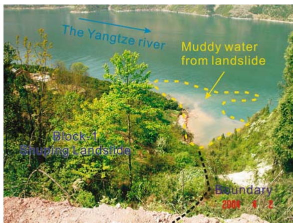
Fig. 40.5. Muddy water seeped out of the toe part of the Shuping landslide
