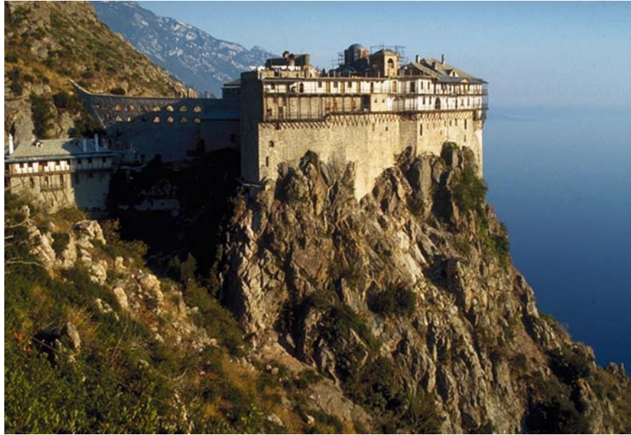
Fig. 30.2. The Simonos Petra Monastery. Important faults of E-W direction are occurred
