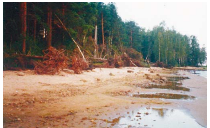
Fig. 46.9. The eastern bank of the Rybinskoe water reservoir (the village of Volkovo). The coastal destruction caused by storms
