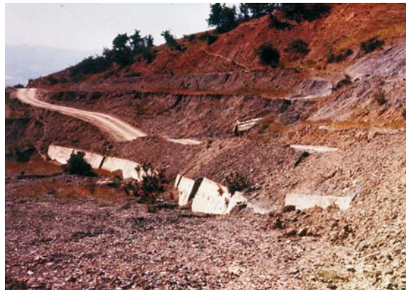
Fig. 37.7. Translational slide along the contact of sandstone and argillaceous phases of flysch
