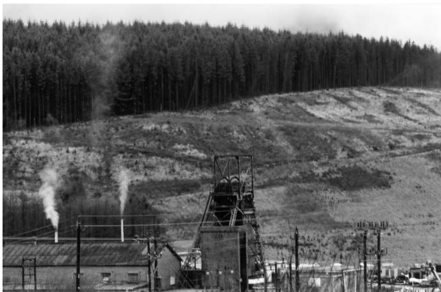
Photo 7.1: The winding gear at Tower Colliery, at the top of the Cynon Valley
