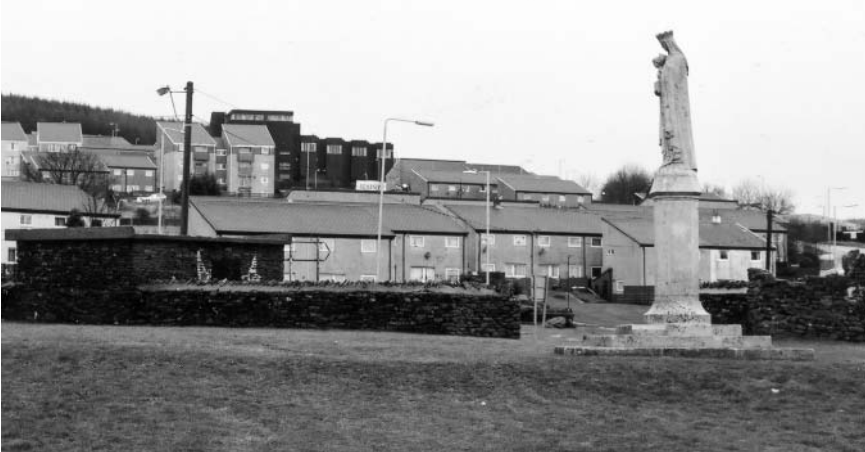
Photo 1.2: Two faces of Penrhys. On a promontory overlooking the Rhondda Fawr valley, Penrhys was visited as a pilgrimage site to the Virgin Mary until the destruction of her statue in 1536. It is now best known for the social housing estate pictured here behind the new statue.
