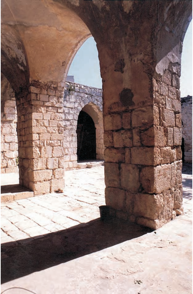
Fig. 4: Safed, The Red Mosque. The open courtyard. General view.
