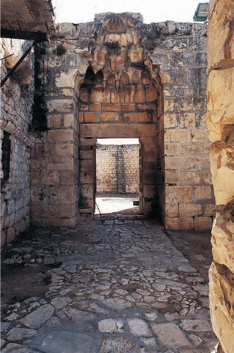
Fig. 3: Safed, The Red Mosque. Muqarnas portal. General view.
