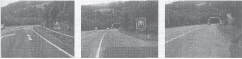
FIG. 1. The reduction of the normal four lane divided freeway cross section to one lane per direction, (Graeberntunnel on A2 in Kaernten)
