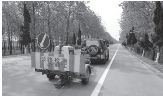
FIG.4.The testing site of the deflection test.
