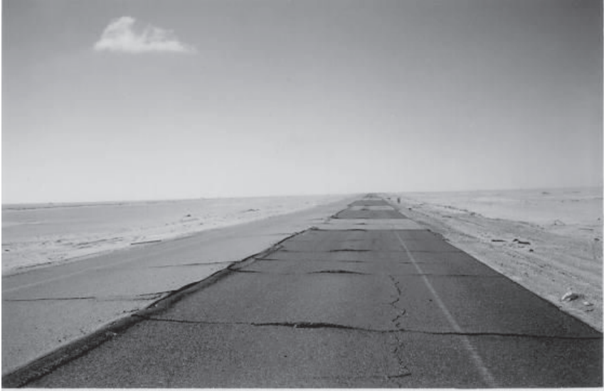
FIG.4. The Effects of temperature and solar radiation on pavement.
