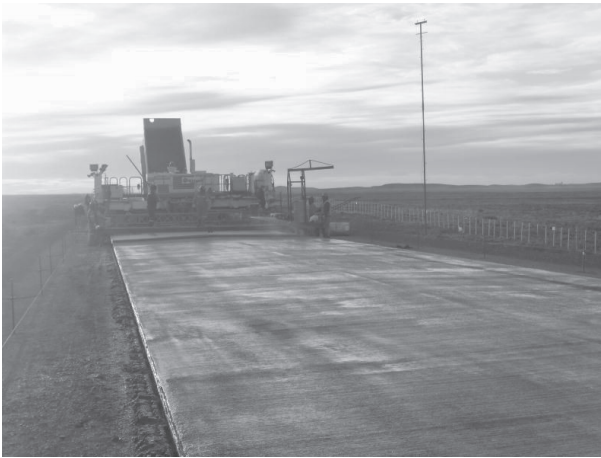
FIG. 6. Paving in one gang with slipformer in Chilean project.
