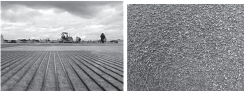
FIG. 1. Grooved runway surface (left) and antiskid runway surface (right).
