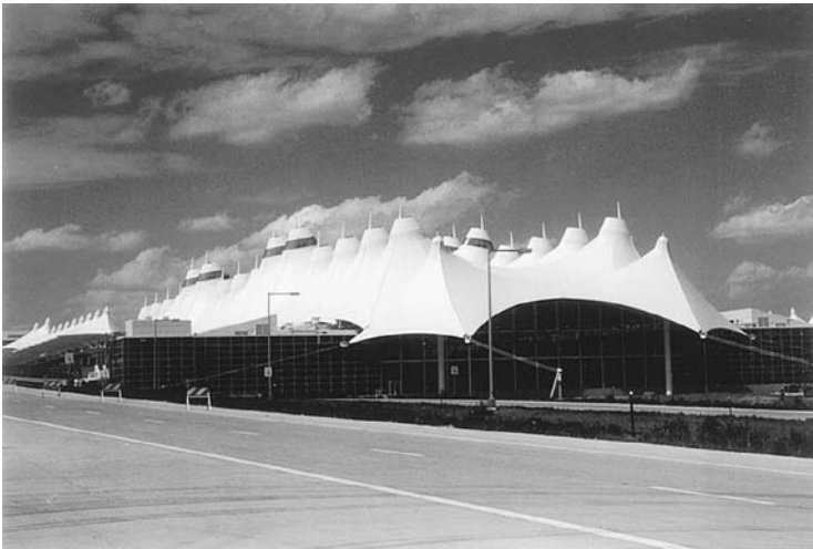
FIGURE F The form of the Denver International Airport roof combines saddle and radial shapes to echo the forms of the surrounding mountains. (Architects: C. W. Fentriss, J. H. Bradburn & Associates. Roof designer and structural engineer: Severud Associates, Horst Berger, Principal Consultant)
