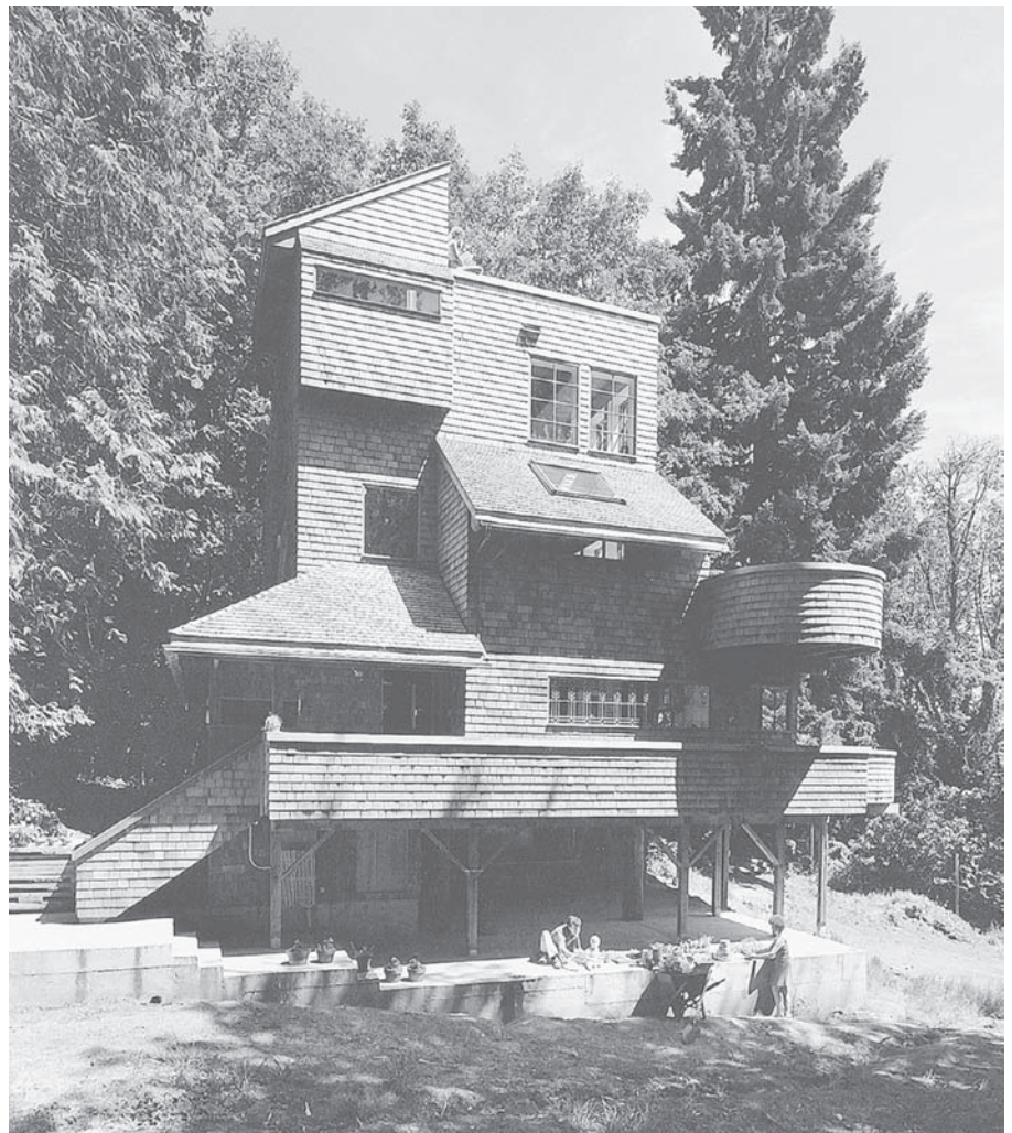
FIGURE 16.58 A house is both roofed and sided with Red cedar shingles to feature its sculptural qualities. (Architect: William Isley. Photo by Paul Harper. Courtesy of Red Cedar Shingle and Handsplit Shake Bureau)
