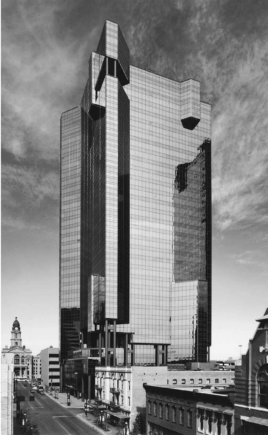
FIGURE 17.13 Reflective coated windows with subtly different reflective coated glass spandrels. (Architects: Paul Rudolph and 3D International. Photo courtesy of PPG Industries)
