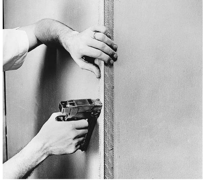
FIGURE 23.19 Stapling a corner bead to veneer plaster base to create a straight, durable corner. (Courtesy of United States Gypsum Company)
