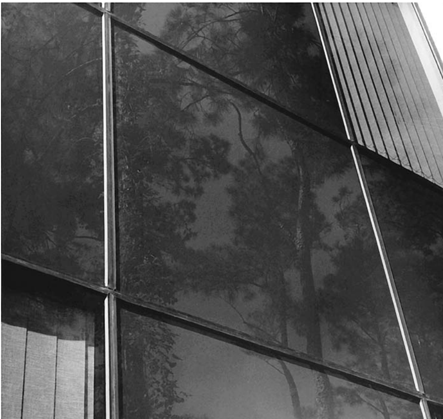
FIGURE 17.19 A finished lockstrip gasket glazing installation. (Courtesy of Standard Products Company)
