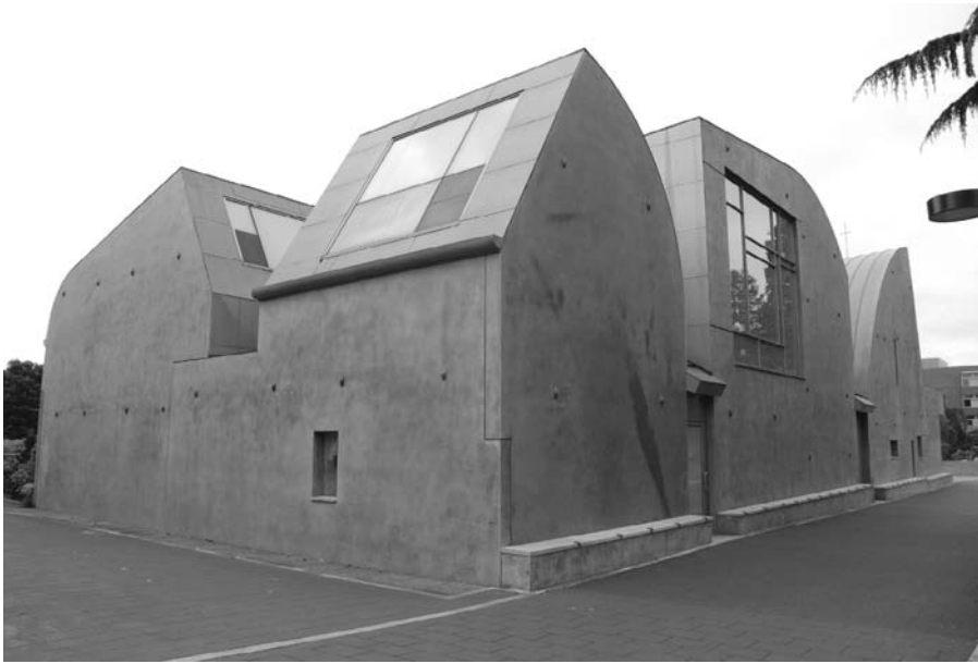
FIGURE 14.60 The Chapel of St. Ignatius, Seattle University, designed by architect Steven Holl, is a tilt-up concrete structure. (Photo by Joseph Iano)
