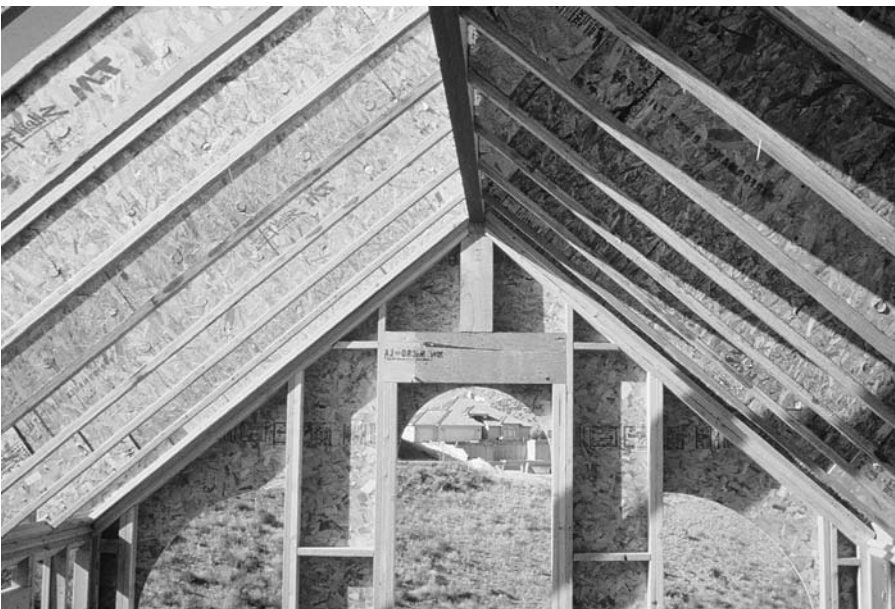
FIGURE 5.60 I-joists may be used as rafter material instead of solid lumber. (Courtesy of Trus Joist MacMillan)
