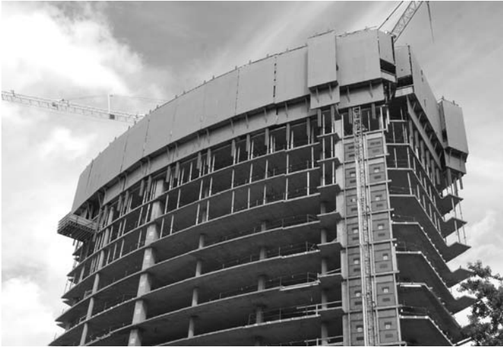
FIGURE 14.20 Banded slab construction. Compare the depth and breadth of the slab band in the center of the building to those of the conventional concrete beams around the perimeter. (Reprinted with permission of the Portland Cement Association from Design and Control of Concrete Mixtures , 12th edition; Photos: Portland Cement Association, Skokie, IL)
