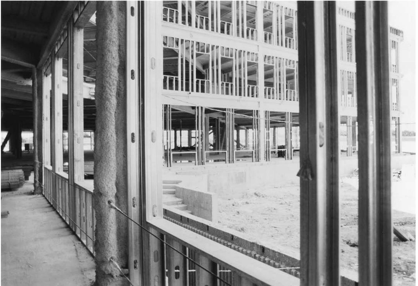
FIGURE 12.13 Light gauge steel stud walls frame the exterior walls of a building whose floors and roof are framed with structural steel. (Courtesy of Unimast Incorporated— www.unimast.com )
