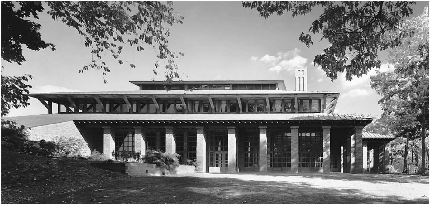
FIGURE 16.59 A standing-seam metal roof with beautifully detailed overhangs, designed by architects Kallmann and McKinnell. (Photo by Steve Rosenthal)
