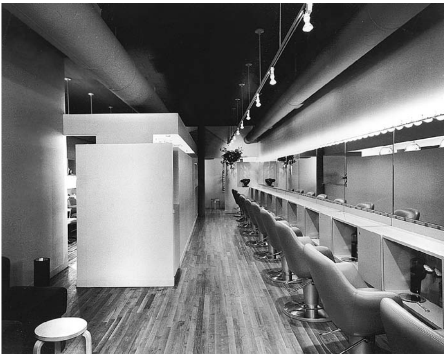
FIGURE 24.34 Oak strip flooring in a hair salon. Notice the use of exposed ducts and a lighting track at the ceiling. (Architects: Michael Rubin and Henry Smith-Miller in association with Kenneth Cohen. Courtesy of Oak Flooring Institute)
