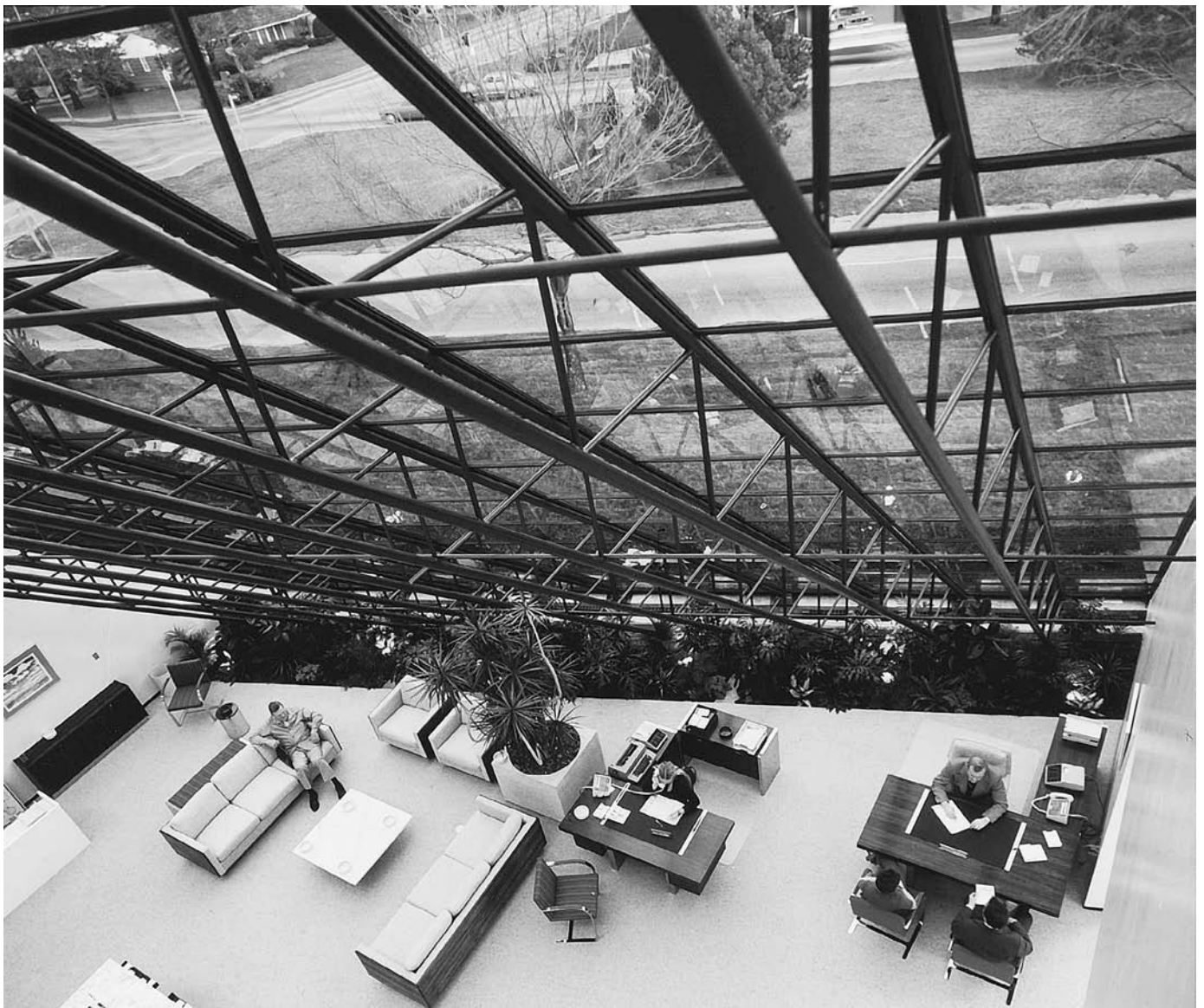
FIGURE 17.9 Laminated glass provides safety against falling shards in an overhead sloped glazing installation. (Courtesy of PPG Industries)
