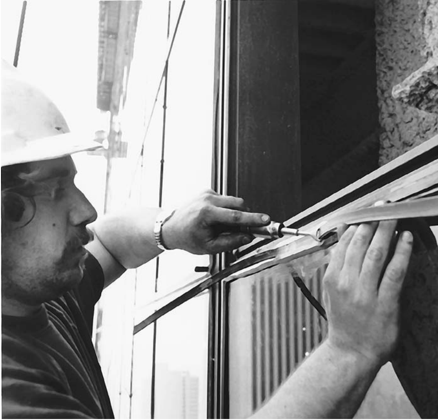
FIGURE 17.18 Inserting the lockstrip into a lockstrip gasket to expand the gasket and seal it against the glass. (Courtesy of Standard Products Company)
