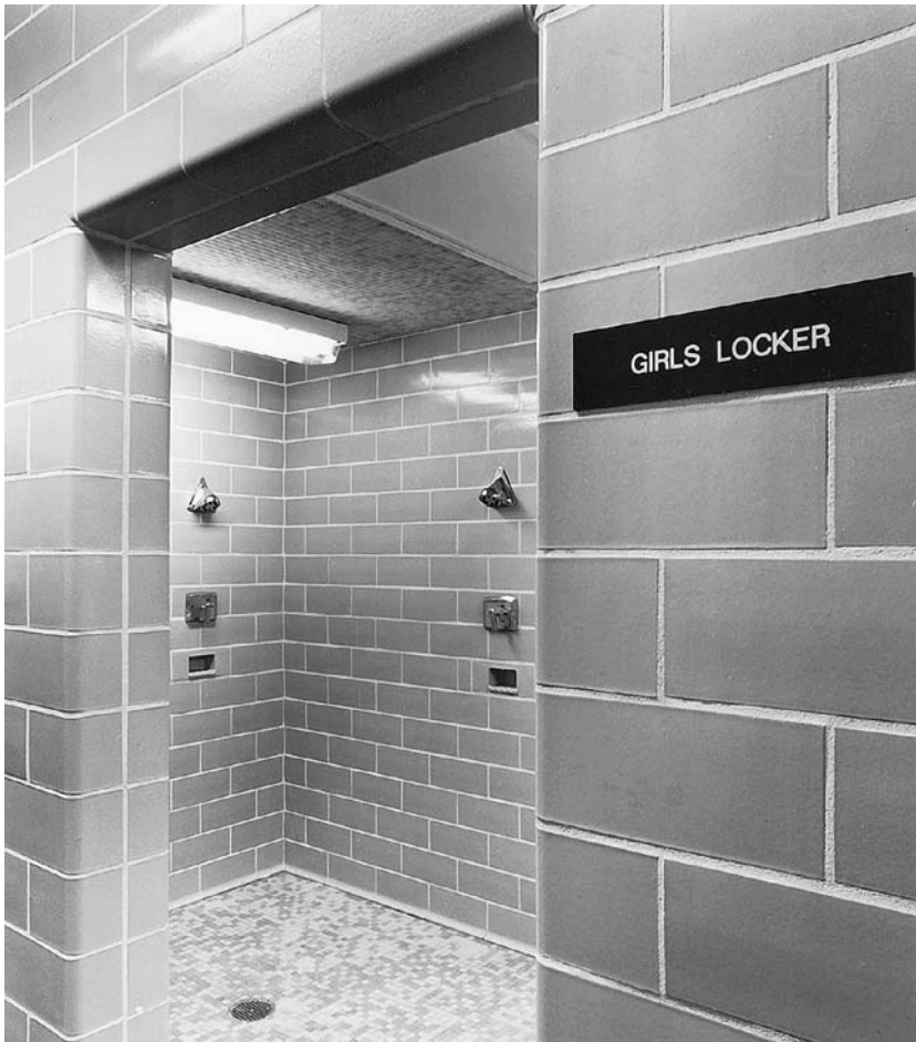
FIGURE 23.40 A glazed structural clay tile partition installation. The floor is finished with glazed ceramic tiles. (Courtesy of Stark Ceramics, Inc.)
