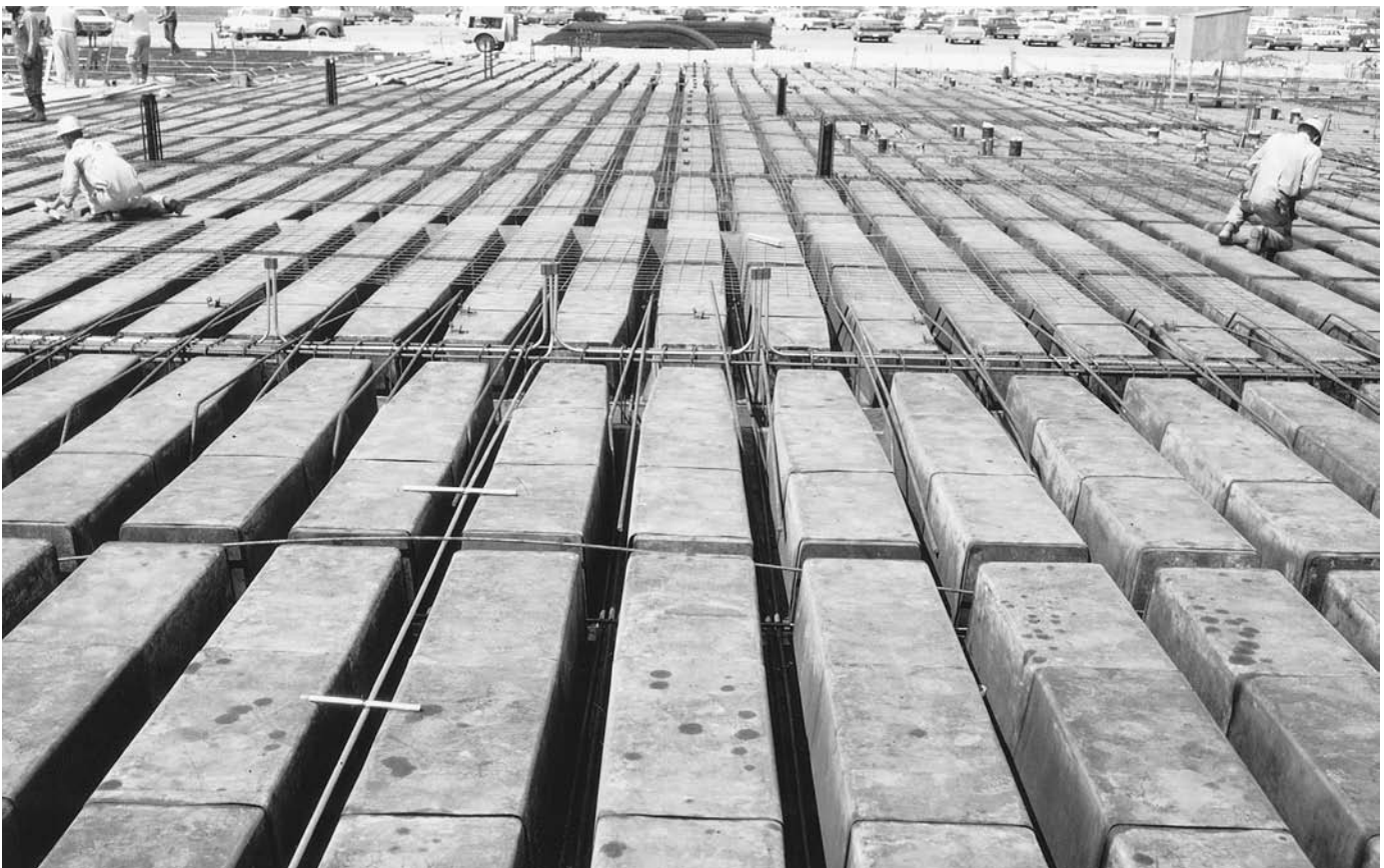
FIGURE 14.24 Reinforcing being placed for a one-way concrete joist floor. Electrical conduits and boxes have been put in place, and welded wire fabric is being installed as shrinkage-temperature reinforcing. Both the tapered end pans and the square endcaps for the midspan distribution rib are clearly visible. (Courtesy of the Ceco Corporation, Oakbrook Terrace, Illinois)
