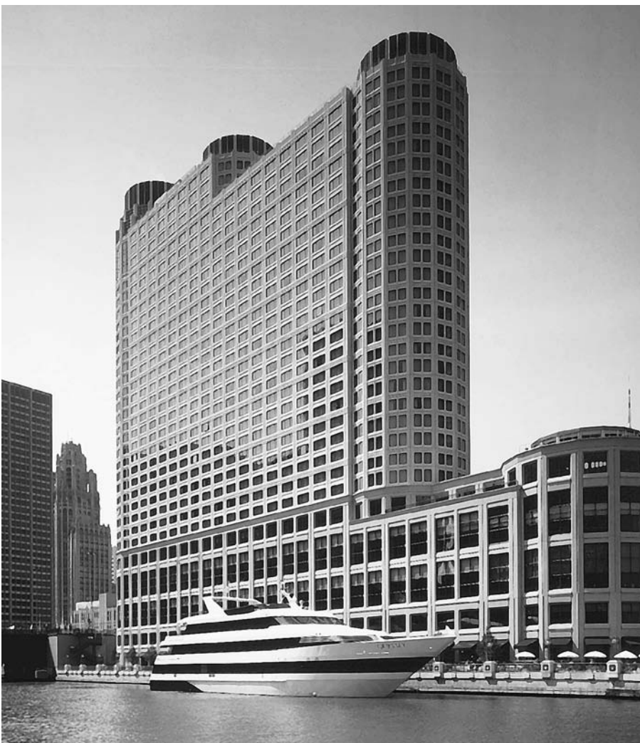
FIGURE 20.15 A Chicago hotel is clad in precast concrete panels. (Architects: Solomon Cordwell Buenz Associates. Photo by Hedrich Blessing)
