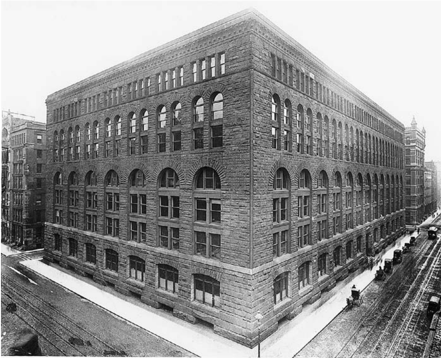
FIGURE 9.16 The Marshall Field Wholesale Store, built in 1885 in Chicago, rested on a two-story base of red granite. Its upper walls were built of red sandstone, and its interior was framed with heavy timber. (Architect: H. H. Richardson. Courtesy of Chicago Historical Society, IChi-01688)
