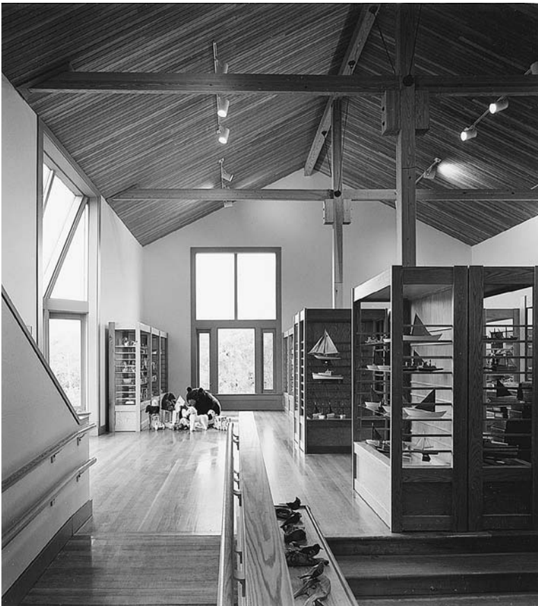
FIGURE 7.41 Varnished oak flooring, millwork, and casework. (Woo & Williams, Architects. Photographer: Richard Bonarrigo)
