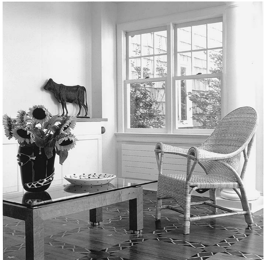
FIGURE 18.6 A pair of double-hung wood-framed windows in a dwelling. (Photo courtesy of Marvin Windows and Doors)
