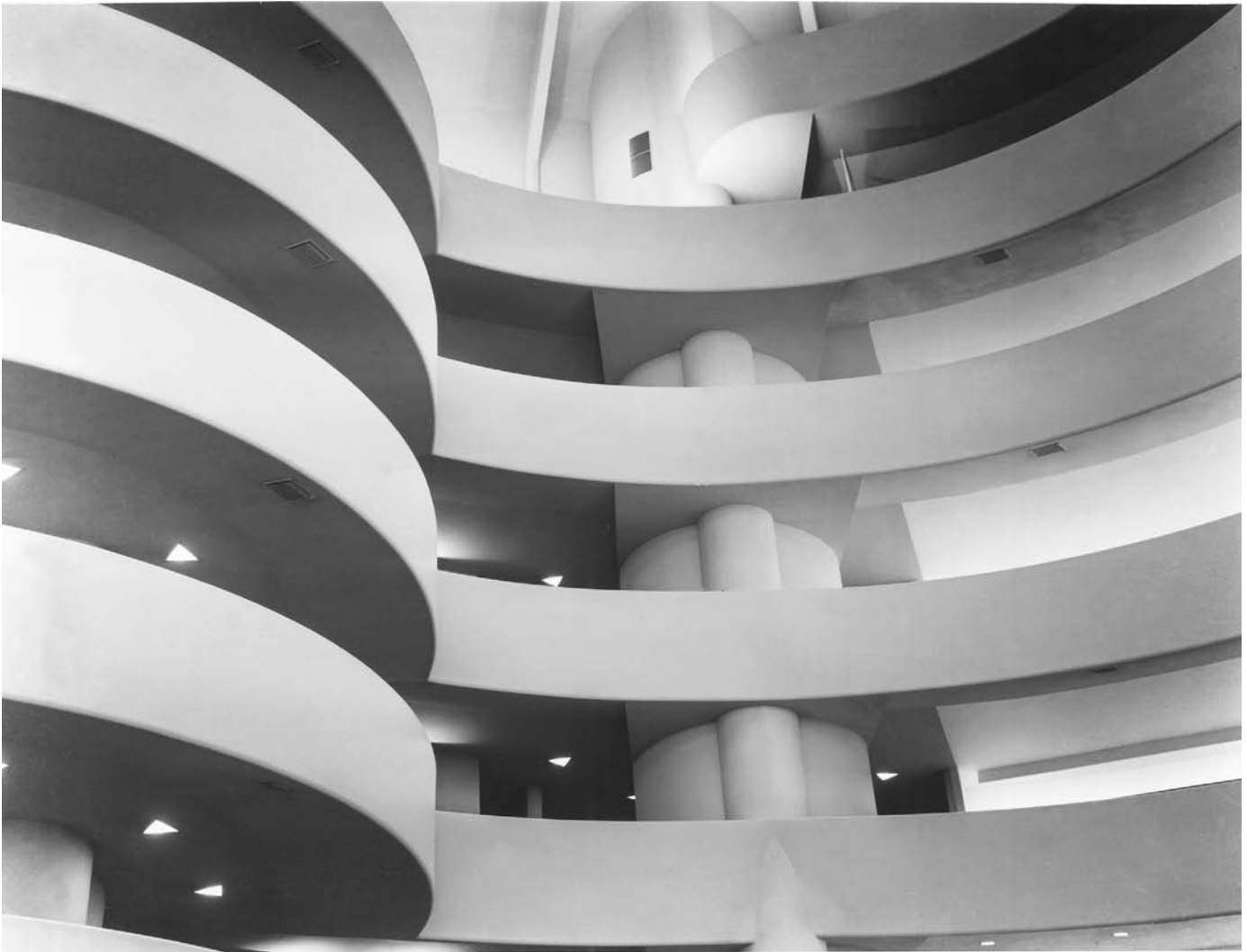
FIGURE 14.59 The plastered surfaces of Frank Lloyd Wright's Guggenheim Museum (1943–1956) cover a helical ramp of cast-in-place concrete. (Photo by Wayne Andrews)
