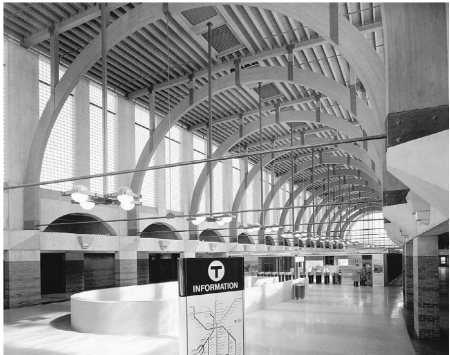
FIGURE 4.29 Semicircular laminated wood arches support the timber roof of the Back Bay Station in Boston. Notice the use of horizontal steel tie rods to resist the thrust of the arches at the base. (Architects: Kallmann, McKinnell & Wood. Photo © Steve Rosenthal)
