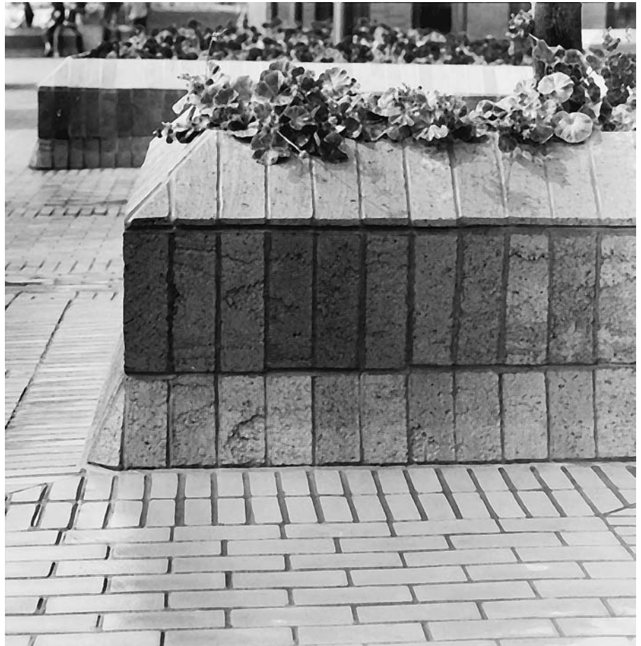
FIGURE 24.26 A floor of glazed brick pavers meets a planter bed constructed of brick masonry. (Courtesy of Stark Ceramics, Inc.)
