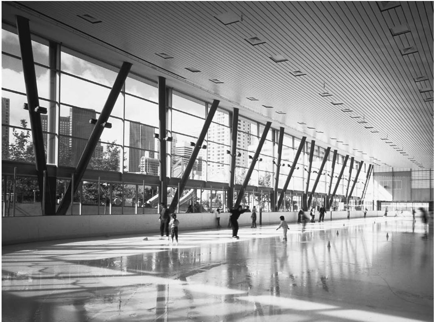
Figure E Interior View.
