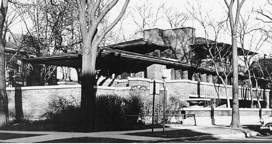
FIGURE 8.45 Frank Lloyd Wright used long, flat Roman bricks and cut limestone wall copings to emphasize the horizontality of the Robie House, built in Chicago in 1906. (Photo by Mildred Mead. Courtesy of Chicago Historical Society, IChi-14191)
