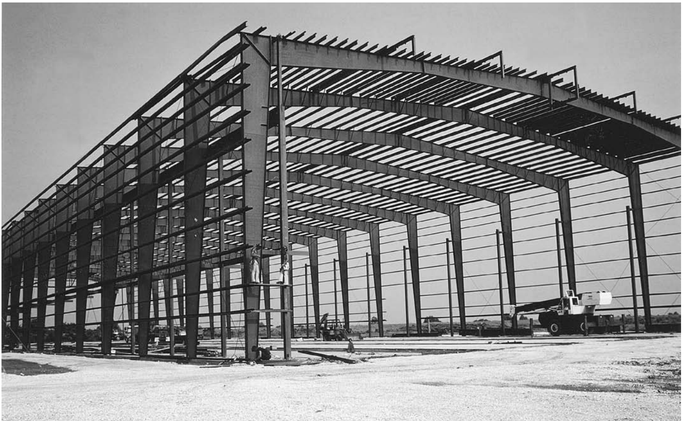
FIGURE 11.80 The steel rigid frames of this industrial building carry steel purlins that will support the roof deck and girts to support the wall cladding. The depth of each frame varies with the magnitude of the bending forces and is greatest at the eave connections, where these forces are at a maximum. (Courtesy of Metal Building Manufacturers Association)
