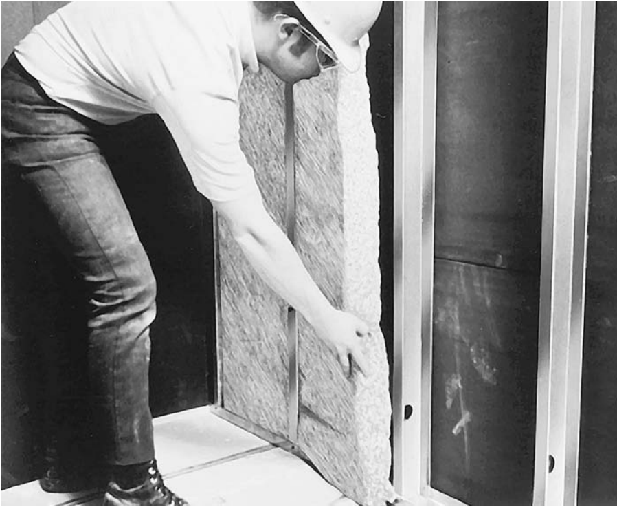
FIGURE 23.36 Installing a sound attenuation blanket. (Courtesy of United States Gypsum Company)
