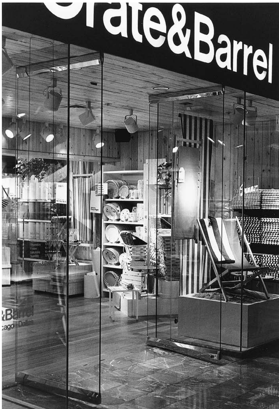
FIGURE 17.7 Tempered glass is used for strength and breakage safety in both the doors and windows of this store in a downtown shopping mall. (Photo by Edward Allen)
