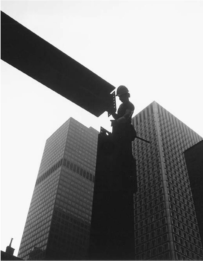
FIGURE 11.52 Connecting a beam to a column. (Courtesy of Bethlehem Steel Corporation)
