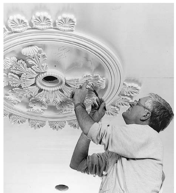
FIGURE D A close-up of Flaharty's blade and template. The template rides on the sledlike runner of the portion under his hand, which is called the "slipper." The long portion of the template, called the "stock," is a radius guide that is fastened to a pin at the end to create the circular form of the medallion. (© Brian McNeill)
