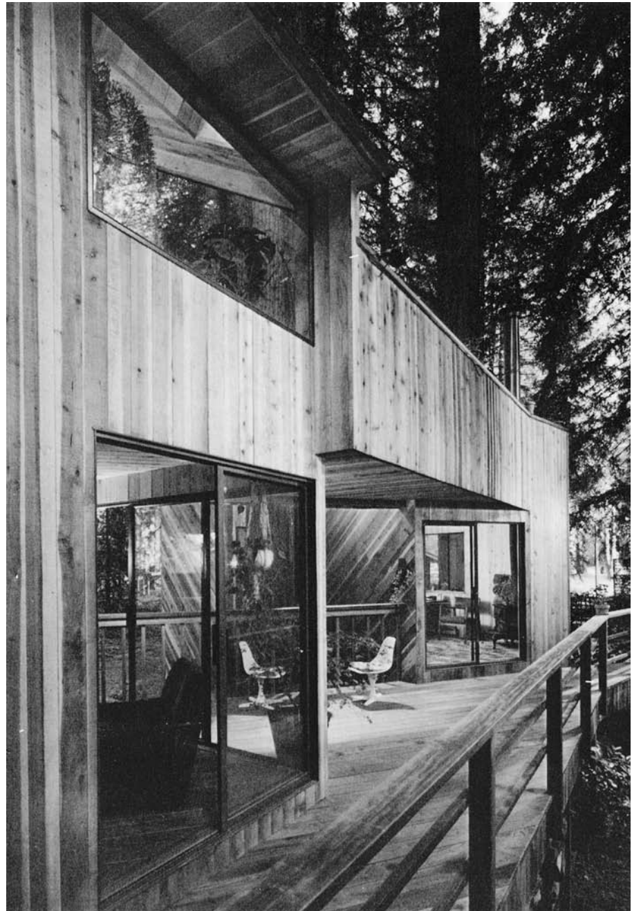
FIGURE 6.19 A completed installation of tongue-and-groove siding, vertically applied in the foreground of the picture and diagonally in the area seen behind the chairs. The lighter-colored streaks are sapwood in this mixed heartwood/sapwood grade of redwood. The windows are framed in dark-colored aluminum. (Architect: Zinkhan/Tobey. Photo by Barbeau Engh. Courtesy of California Redwood Association)
