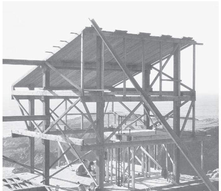
FIGURE 4.34 Each of the attached dwellings in Sea Ranch Condominium #1 at Sea Ranch, in northern California, built in 1965, is framed with a simple cage of unplanned timbers sawn from trees taken from another portion of the site. The diagonal members are wind braces. (Architects: Moore, Lyndon, Turnbull, and Whitaker. Photo by Edward Allen)
