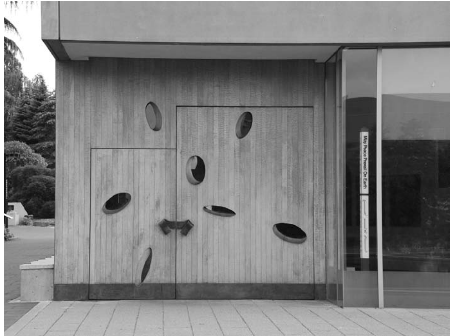
FIGURE 18.29 Custom wood doors on architect Steven Holl's The Chapel of St. Ignatius. (Photo by Joseph Iano)
