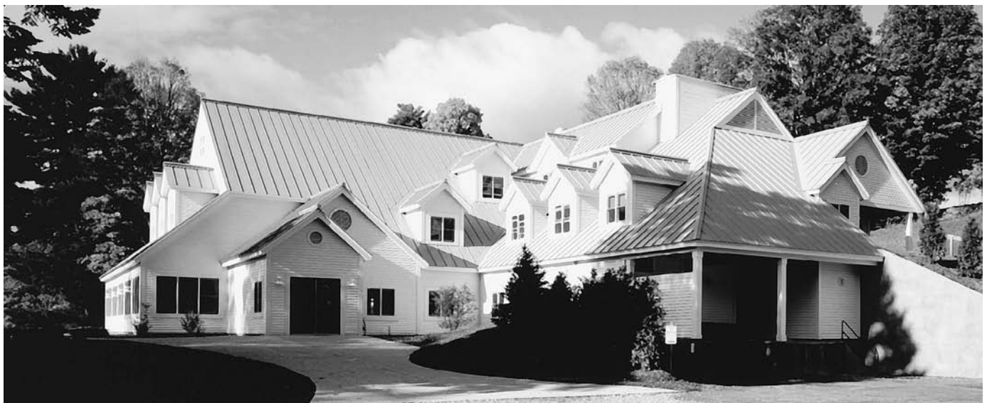
FIGURE 16.54 The raised seams in the architectural panel metal roof accentuate the complex roof geometries of the International Center in Brattleboro, Vermont. (Architect: William A. Hall Partnership. Photo by Stanley Jesudowich)
