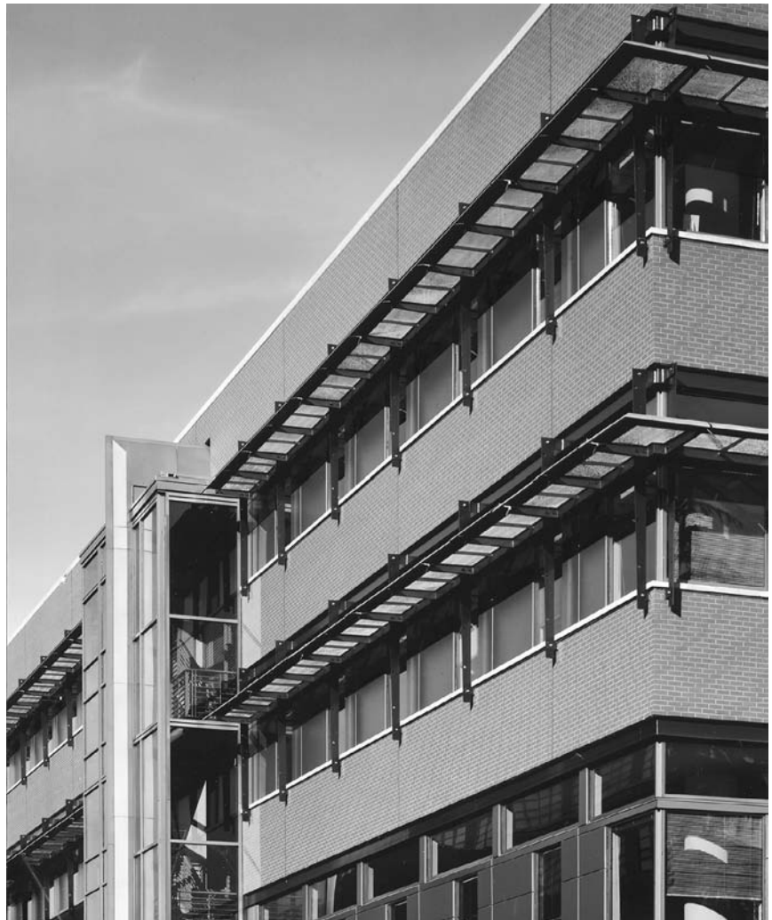
Figure D Photo detail of veneer and channel support.
