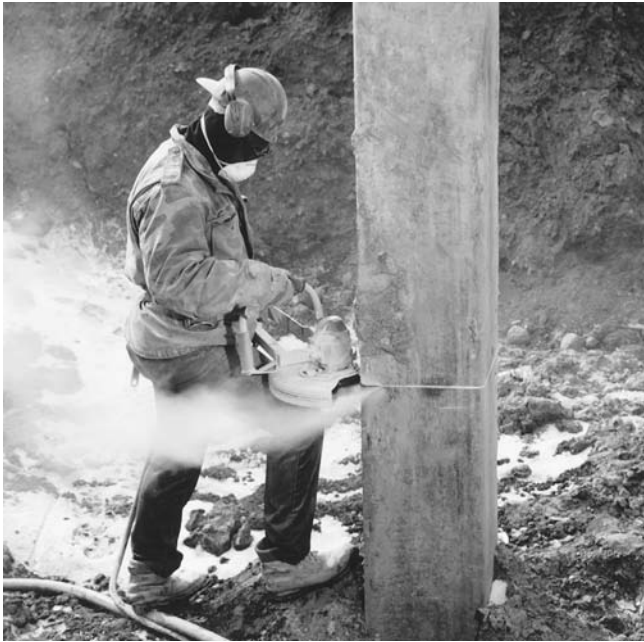
FIGURE B A hand-held pneumatically powered diamond circular saw cuts excess length from a concrete pile. (Courtesy of Sinco Products, Inc.)
