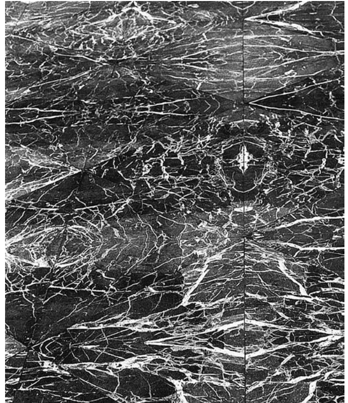
FIGURE 24.24 Flooring of matched, polished triangles of white-veined red marble gives a kaleidoscopic effect. (Architect: The Architects Collaborative. Photo by Edward Allen)
