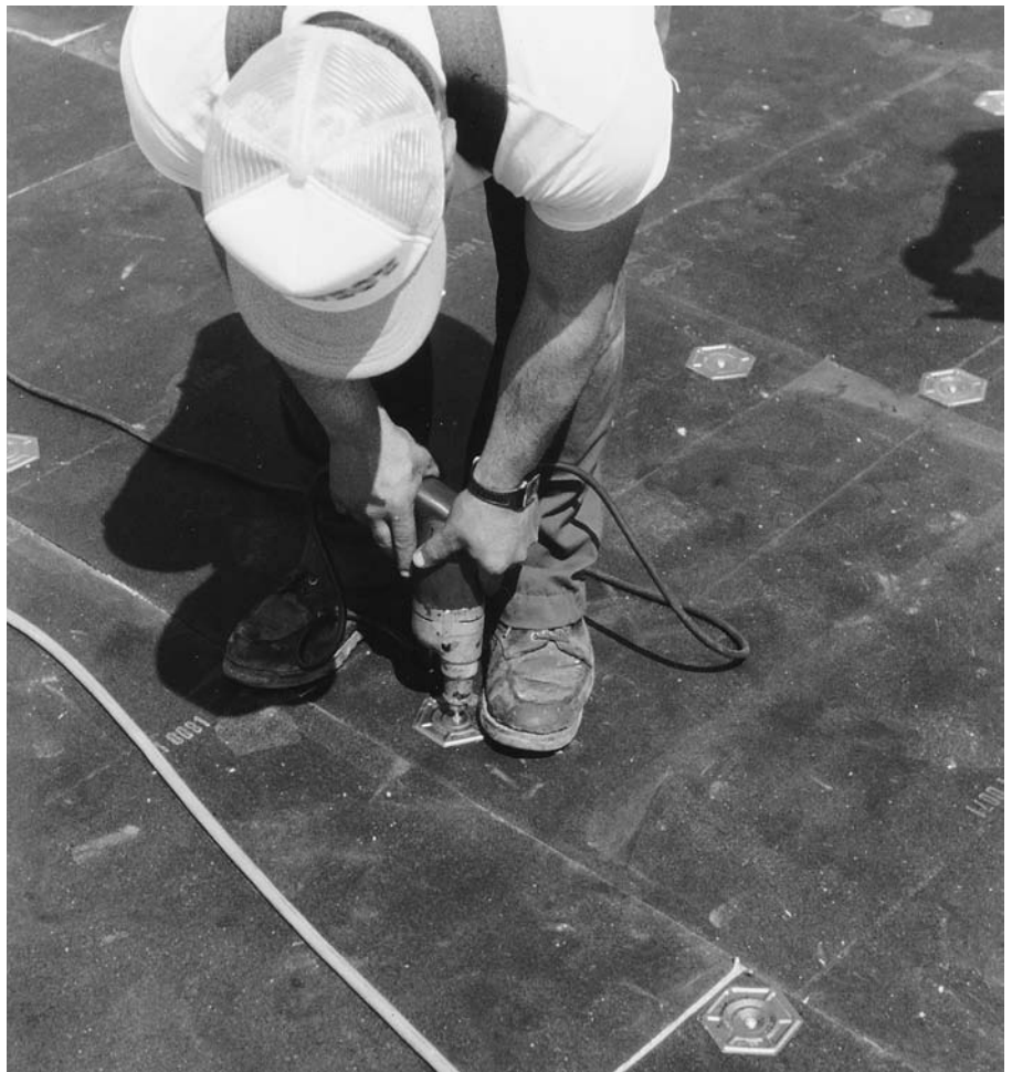
FIGURE 16.12 Screws and large sheet metal washers attach insulation more securely to a metal deck than can hot asphalt. (Courtesy of GAF Corporation)
