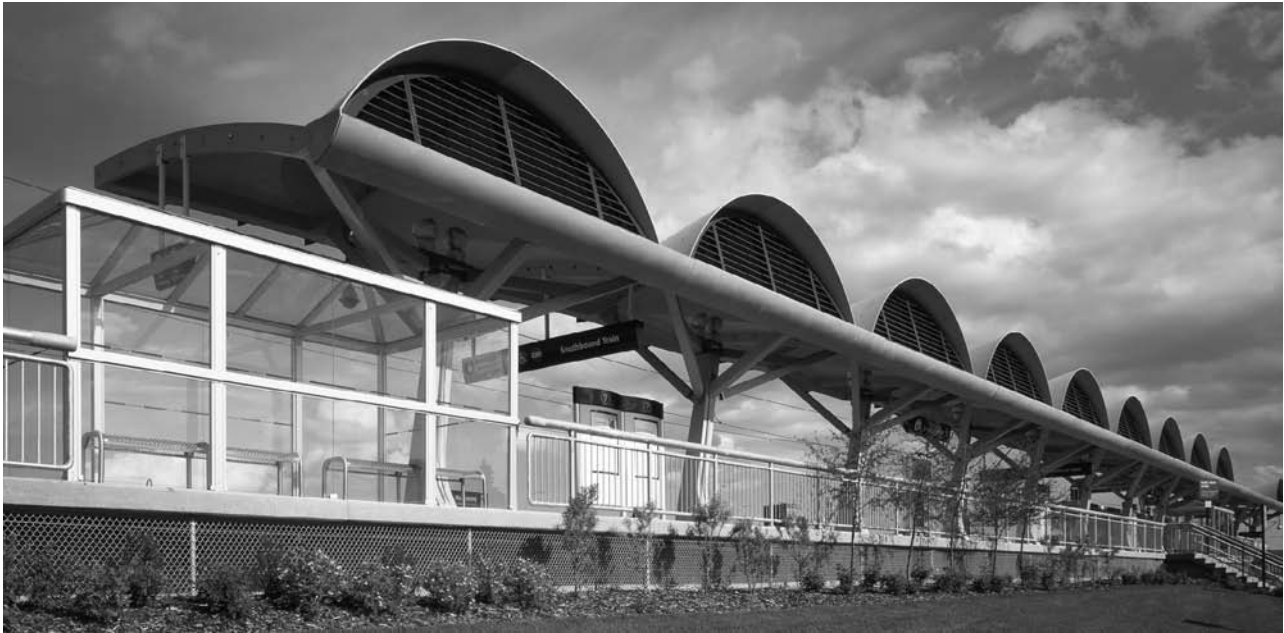
FIGURE 13-43 The Shawnessy LRT Station in Calgary, Alberta, designed by Stantec Architecture, Ltd. The canopy shells were cast from ultra-high-performance concrete and are only \frac{3}{4} inch (19 mm) thick. (Courtesy of Lafarge North America, Inc. Photography by Tucker Photography)
