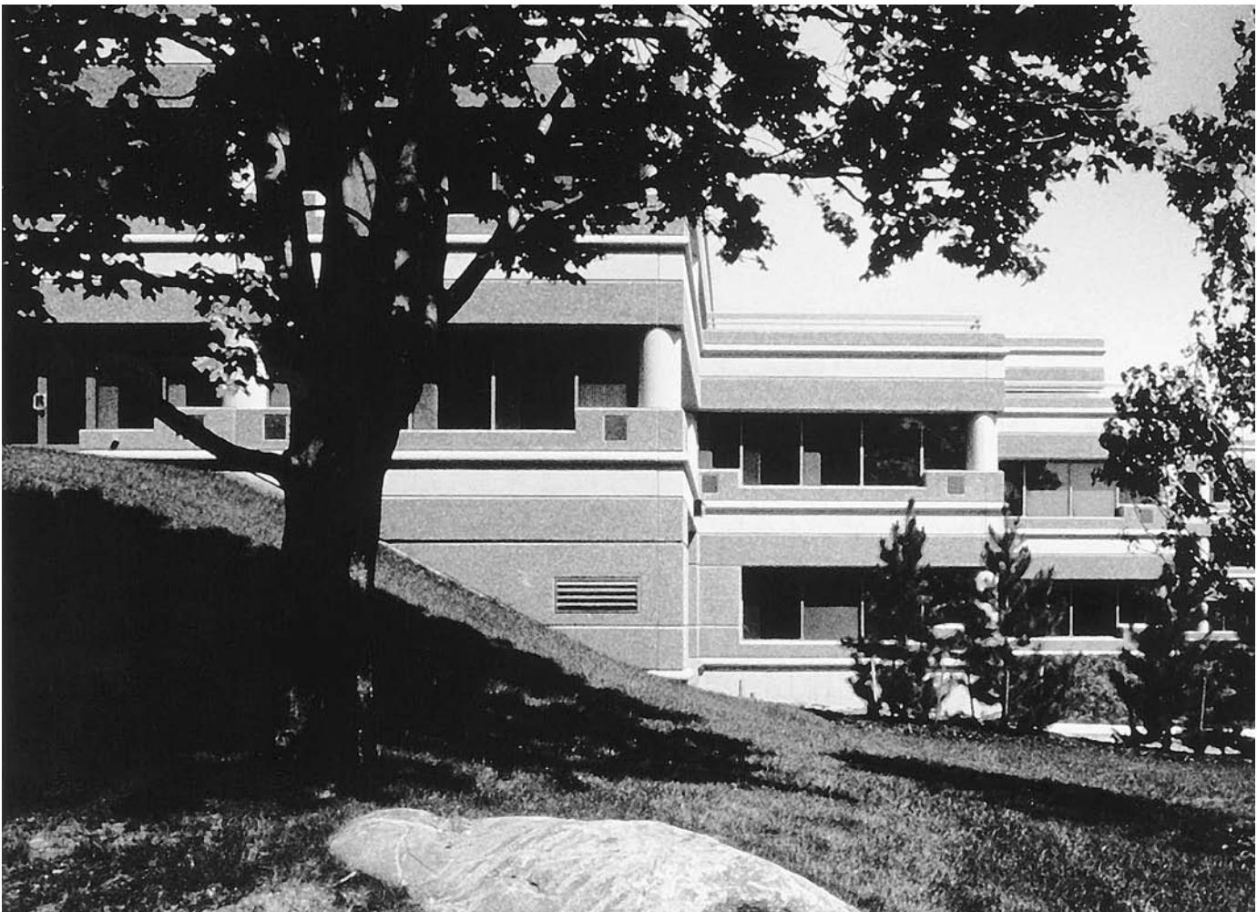
FIGURE 20.16 Horizontal bands of smooth and textured precast concrete create the facade pattern of this suburban office building. (Architect: ADD, Inc. Courtesy of Precast/Prestressed Concrete Institute)
