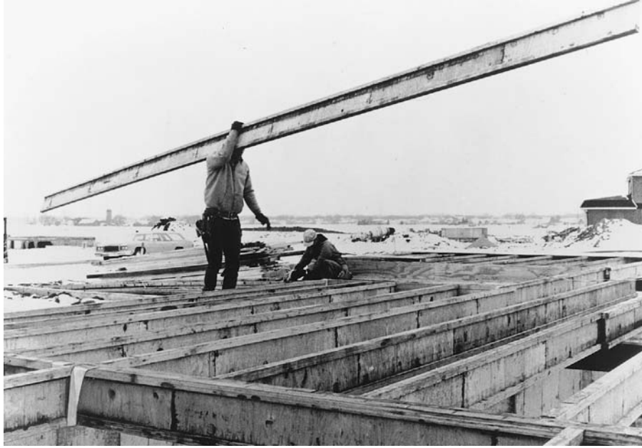
FIGURE 5.24 Various types of manufactured joists and floor trusses are often used instead of dimension lumber. This I-joist has laminated veneer lumber (LVL) flanges and a plywood web. I-joists are manufactured in very long pieces and tend to be straighter, stronger, stiffer, and lighter in weight than sawn joists. (Courtesy of Trus Joist MacMillan)
