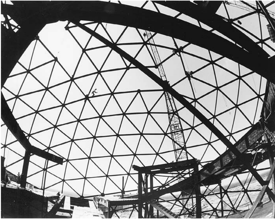
FIGURE 11.87 Erecting the steel dome at Disney World. (© Walt Disney Productions. Permission of American Institute of Steel Construction)
