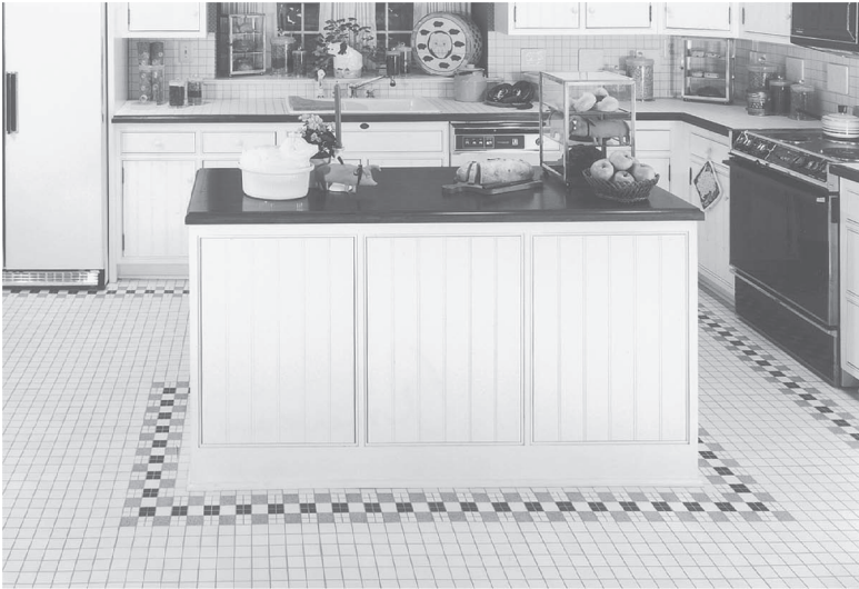
FIGURE 7.40 Ceramic tile is used for the floor, countertops, and backsplash in this kitchen. The border was made by selectively substituting tiles of four different colors for the white tiles used for the field of the floor. (Designer: Kevin Cordes. Courtesy of American Olean Tile)
