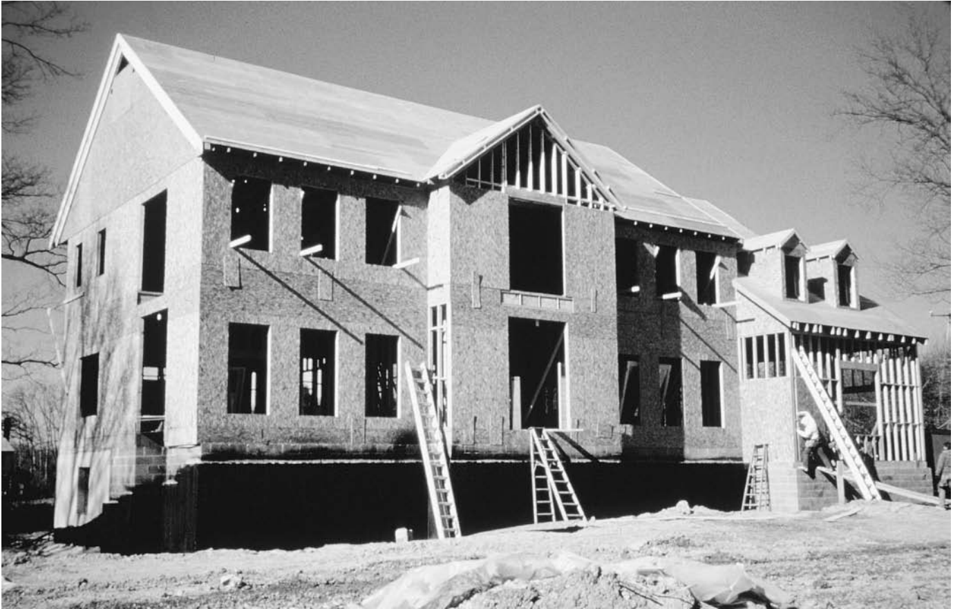
FIGURE 5.63 A light wood frame structure fully sheathed with OSB structural panels.
