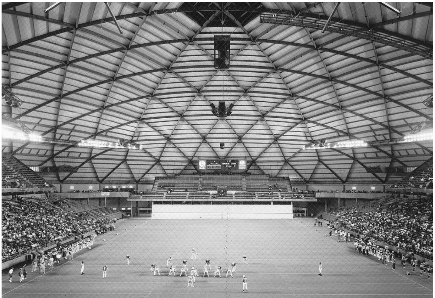
FIGURE 4.31 This laminated wood dome spans 530 feet (161.5 m) to cover a 25,000-seat stadium and convention center in Tacoma, Washington. (Architects: McGranahan, Messenger Associates. Structural engineers: Chalker Engineers, Inc. Photo by Gary Vannest. Courtesy of American Wood Council)
