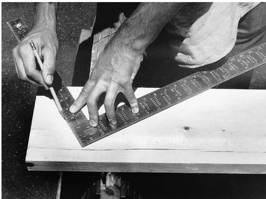
FIGURE 5.58 A framing square being used to mark rafter cuts. The run of the roof, 12 inches, is aligned with the edge of the rafter on the blade (the wider leg) of a square, and the rise, 7 inches in this case, is aligned on the tongue (the narrower leg) of the square. A pencil line along the tongue will be perfectly vertical ( a plumb cut ) when the rafter is installed in the roof, and one along the blade will be horizontal ( a level cut ). True horizontal and vertical distances can be measured on the blade and tongue, respectively. The layout of these types of cuts can also be seen in Figures 5.52 and 5.56. (Photo by Edward Allen)
