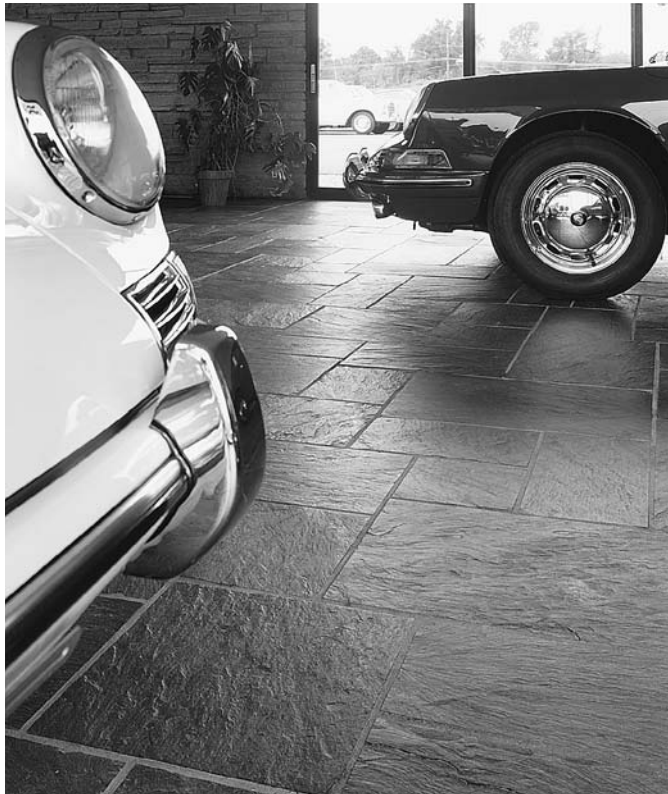
FIGURE 24.23 A slate floor in an automobile showroom. (Photo by Bill Engdahl, Hedrich Blessing. Courtesy of Buckingham-Virginia Slate Company)
