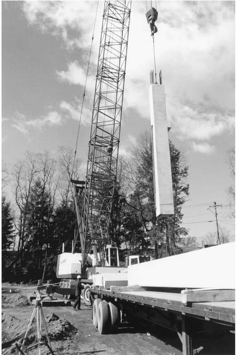
FIGURE 15.34 (a) A crane lifts a column section from a flatbed truck to begin erection of a tennis stadium in New Haven, Connecticut.
