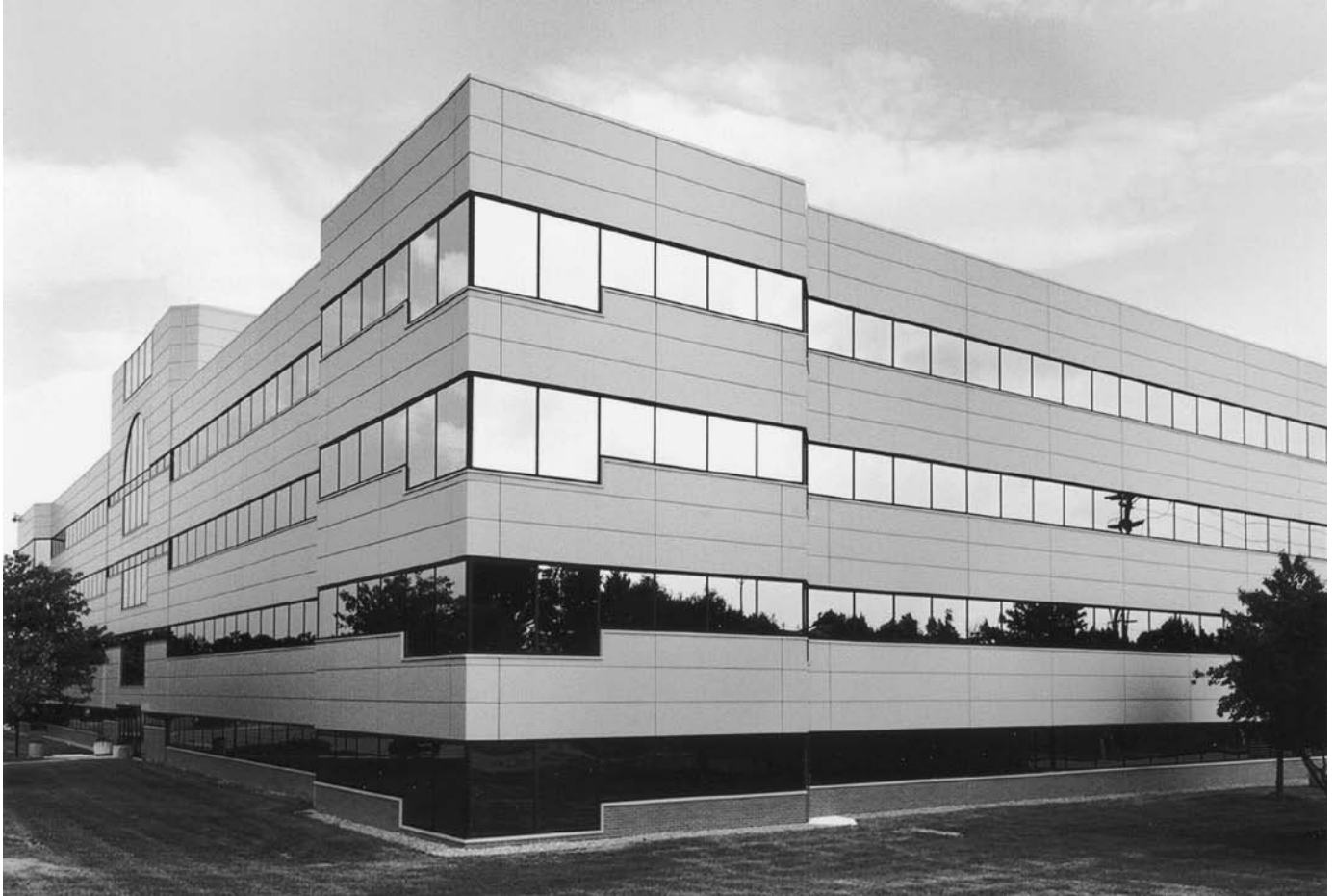
FIGURE 21.25 CENTRIA Form-A-Wall panels present a neat appearance that features the pattern of the open joints. Notice that special panels are used for corners; there is no seam at the corner itself. (Courtesy of CENTRIA)
