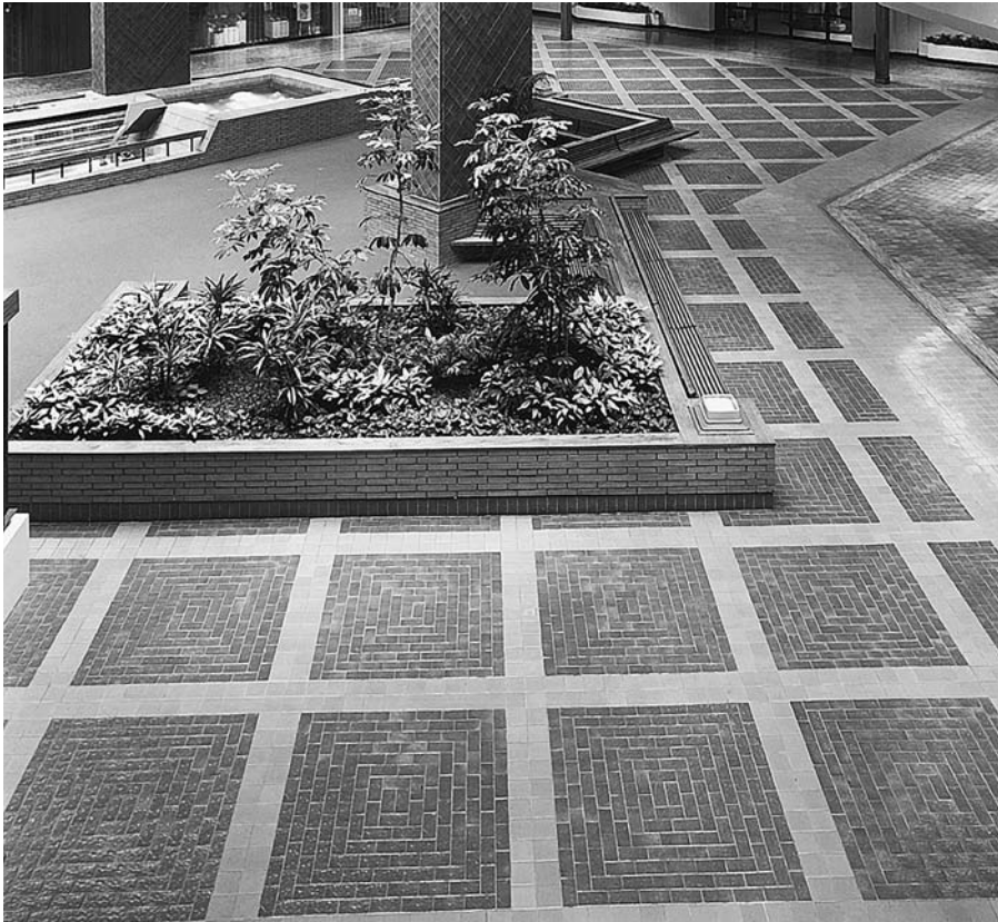
FIGURE 24.28 Square and rectangular quarry tiles in contrasting colors create a pattern on the floor of a retail mall. (Architect: Edward J. DeBartolo Corp. Courtesy of American Olean Tile Company)
