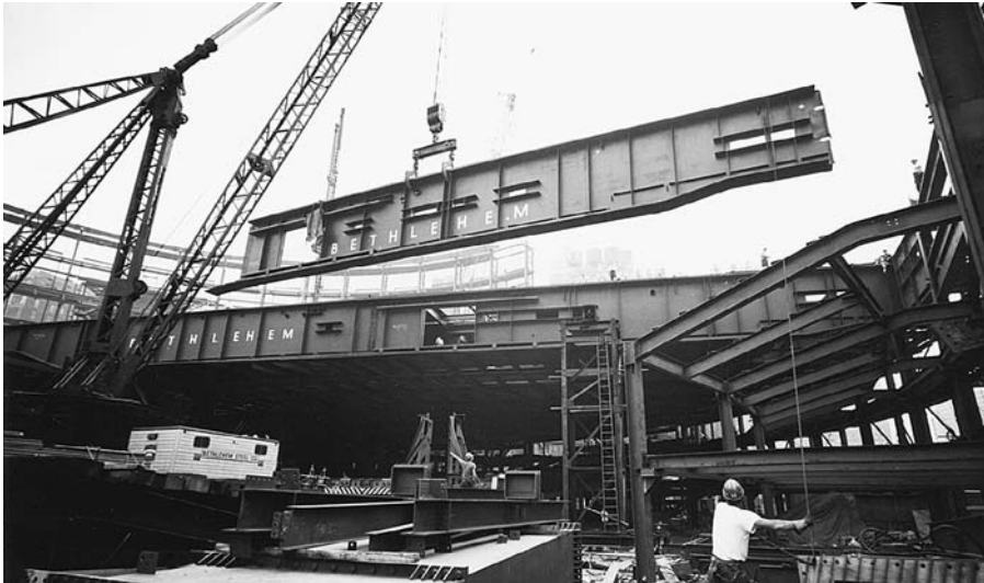
FIGURE 11.79 Erecting a welded steel plate girder. Notice how the girder is custom made with cutouts for the passage of pipes and ductwork. The section being erected is 115 feet (35 m) long, 13 feet (4 m) deep, and weighs 192,000 pounds (87,000 kg). (Courtesy of Bethlehem Steel Corporation)
