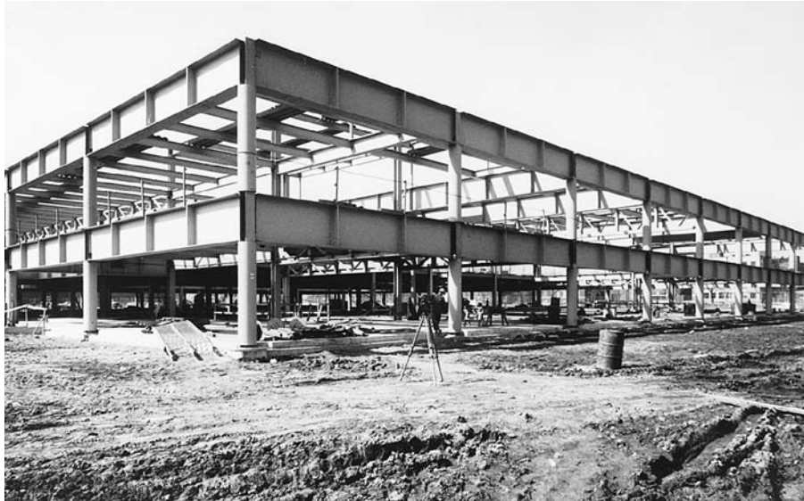
FIGURE 11.94 The Chicago Police Training Center expresses elegantly the logic and simplicity of a straightforward steel frame. (Architect: Jerome R. Butler, Jr. Engineer: Louis Koncza. Permission of American Institute of Steel Construction)
