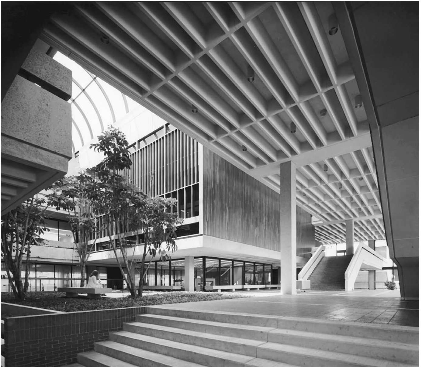
FIGURE 15.38 Highly customized precast concrete framing is used in this courthouse by architect Eduardo Catalano. (Photo by Gordon H. Schenk, Jr. Courtesy of the architect)
