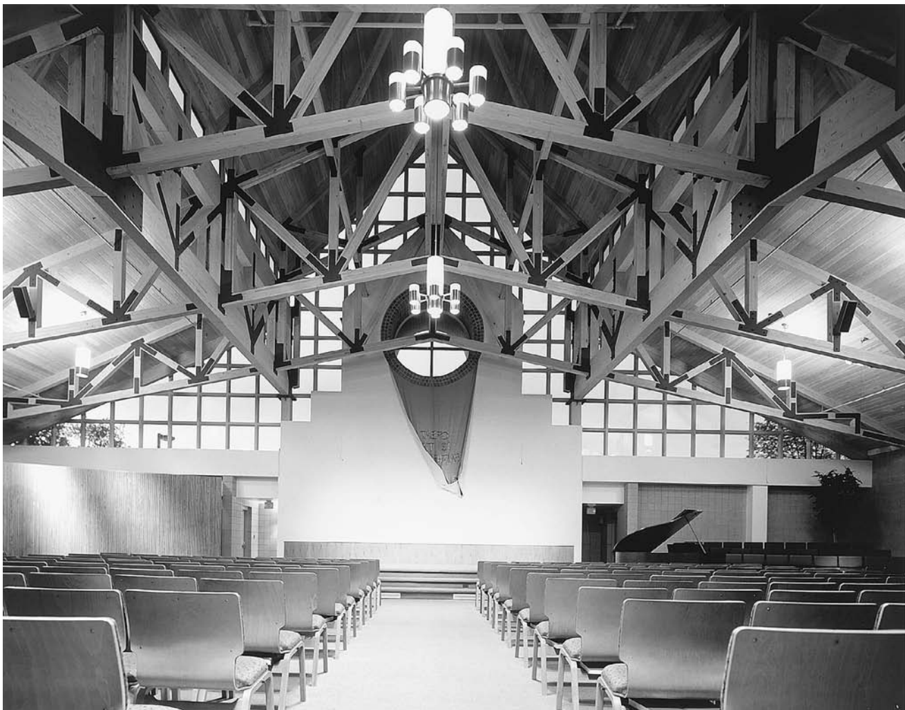
FIGURE 18.30 The Blanchard Road Alliance Church in Wheaton, Illinois, silhouettes laminated wood trusses against a wall of vinyl-clad wood frame fixed windows. (Architect: Walter C. Carlson Associates. Photo courtesy Andersen Windows, Inc. Andersen is a registered trademark of Andersen Corporation, copyright 1997. All rights reserved)
