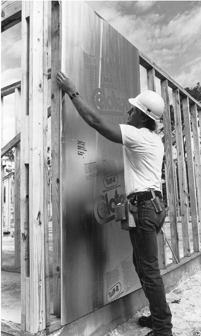
FIGURE 5.42 Applying a panel of insulating foam sheathing. Because this type of sheathing is too soft and weak to brace the frame, diagonal bracing is inserted into the outside faces of the studs at the corners of the building. Steel bracing, nailed at each stud, is used in this frame and is visible just to the right of the carpenter's leg. (Courtesy of The Celotex Corporation)
