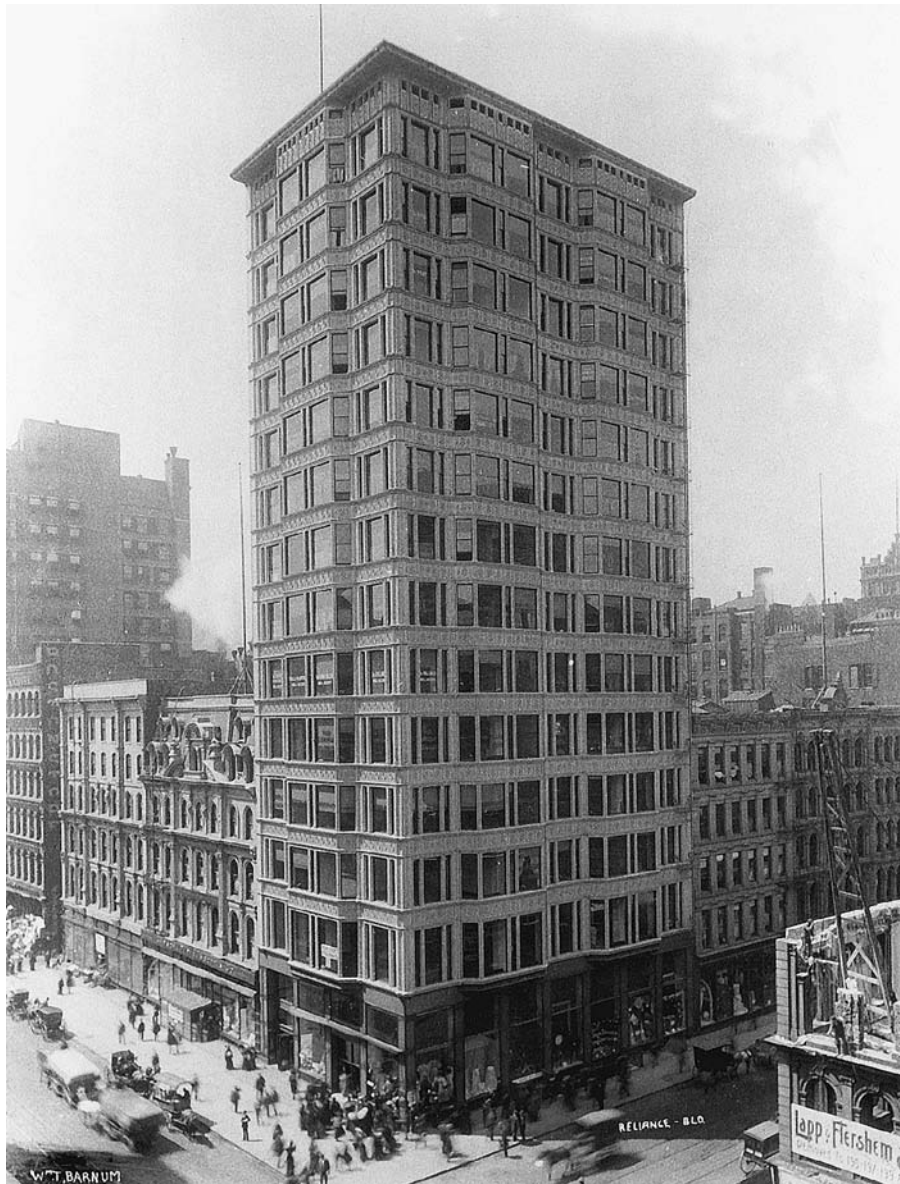
FIGURE 19.2 The curtain wall of Chicago's Reliance Building, built in 1894–1895, has spandrels constructed of white terra-cotta tiles. (Architect: Charles Atwood, of Daniel H. Burnham and Company. Photo by Wm. T. Barnum. Courtesy of Chicago Historical Society ICHi-18294)
