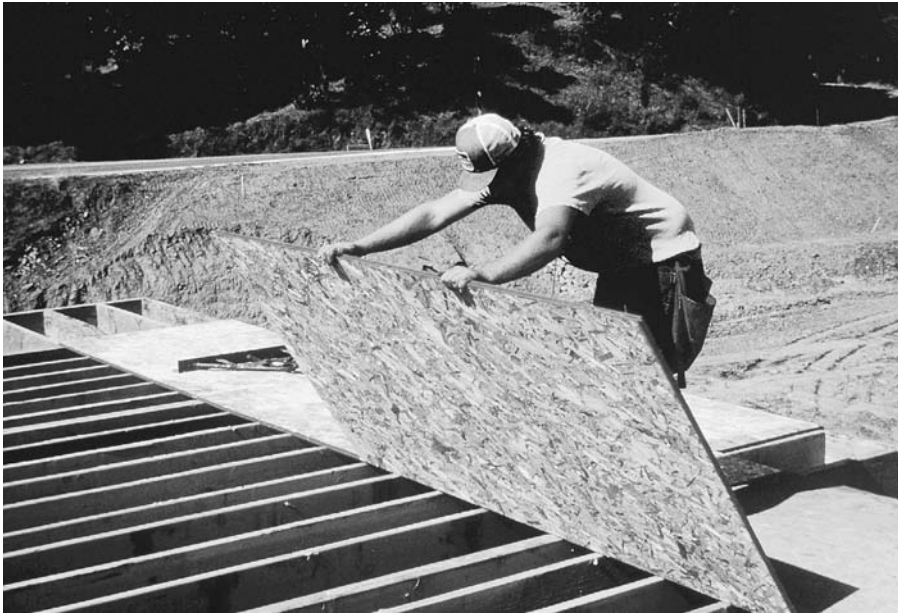
FIGURE 5.26 Applying OSB subflooring. Note that the longer dimension of the panel runs perpendicular to the joist framing. (Courtesy of APA—The Engineered Wood Association)
