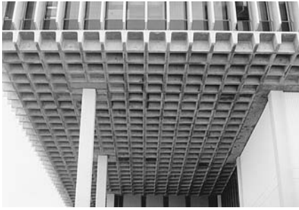
FIGURE 14.39 The underside of a two-way concrete joist floor. Notice how the joists are cantilevered beyond the column line for maximum structural efficiency. (Courtesy of the Ceco Corporation, Oakbrook Terrace, Illinois)
