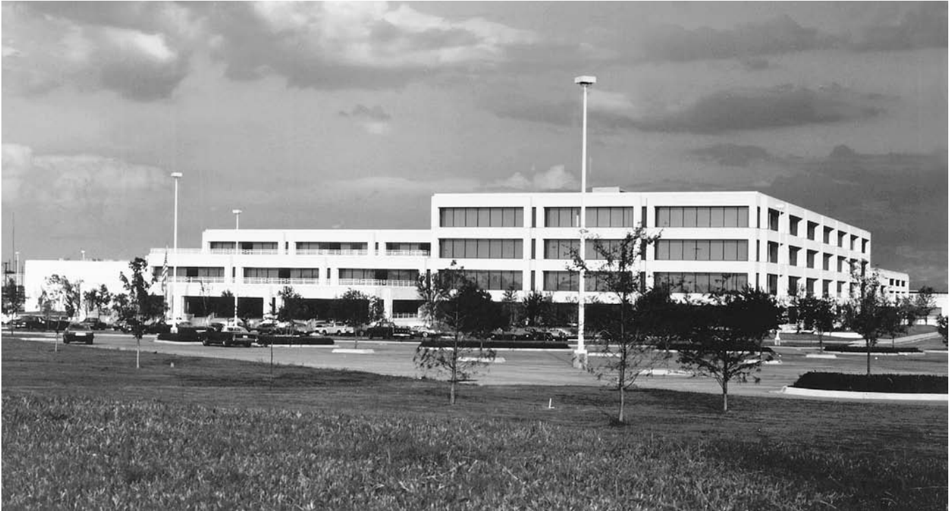
FIGURE 15.35 A low-rise office building in Texas shows a carefully detailed frame of precast concrete. (Architects: Omniplan Architects. Courtesy of Precast/Prestressed Concrete Institute)
