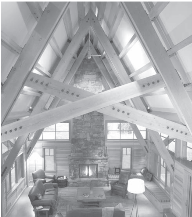
FIGURE 4.33 Dramatic exposed timber scissor trusses support a steeply sloping roof structure in this vacation cabin designed by Nils Finne in the North Cascade Mountains of Washington State. (Architect: FINNE Architects www.FINNE.com ; photograph by Art Grice)
