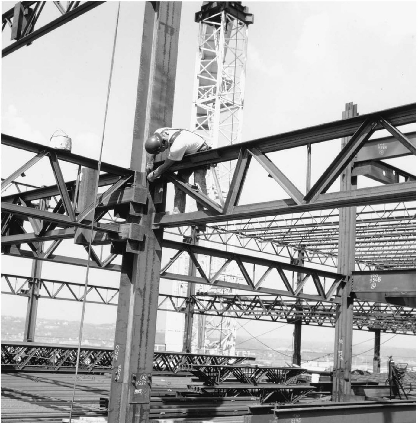
FIGURE 11.54 Bolting joist girders to a column. (Courtesy Vulcraft Division of Nucor)
