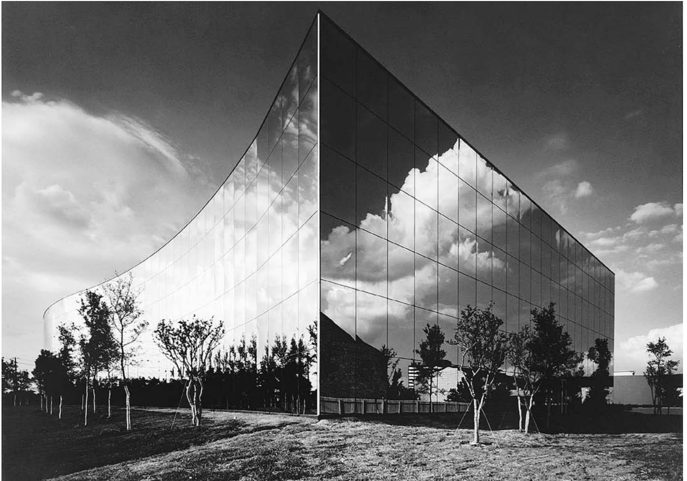
FIGURE 17.25 Reflective glass mounted with a four-side structural silicone glazing system shows no metal on the exterior of this Texas office building, only thin lines of sealant. (Architects: Haldeman, Miller, Bregman & Haman. Photo courtesy of PPG Industries)
