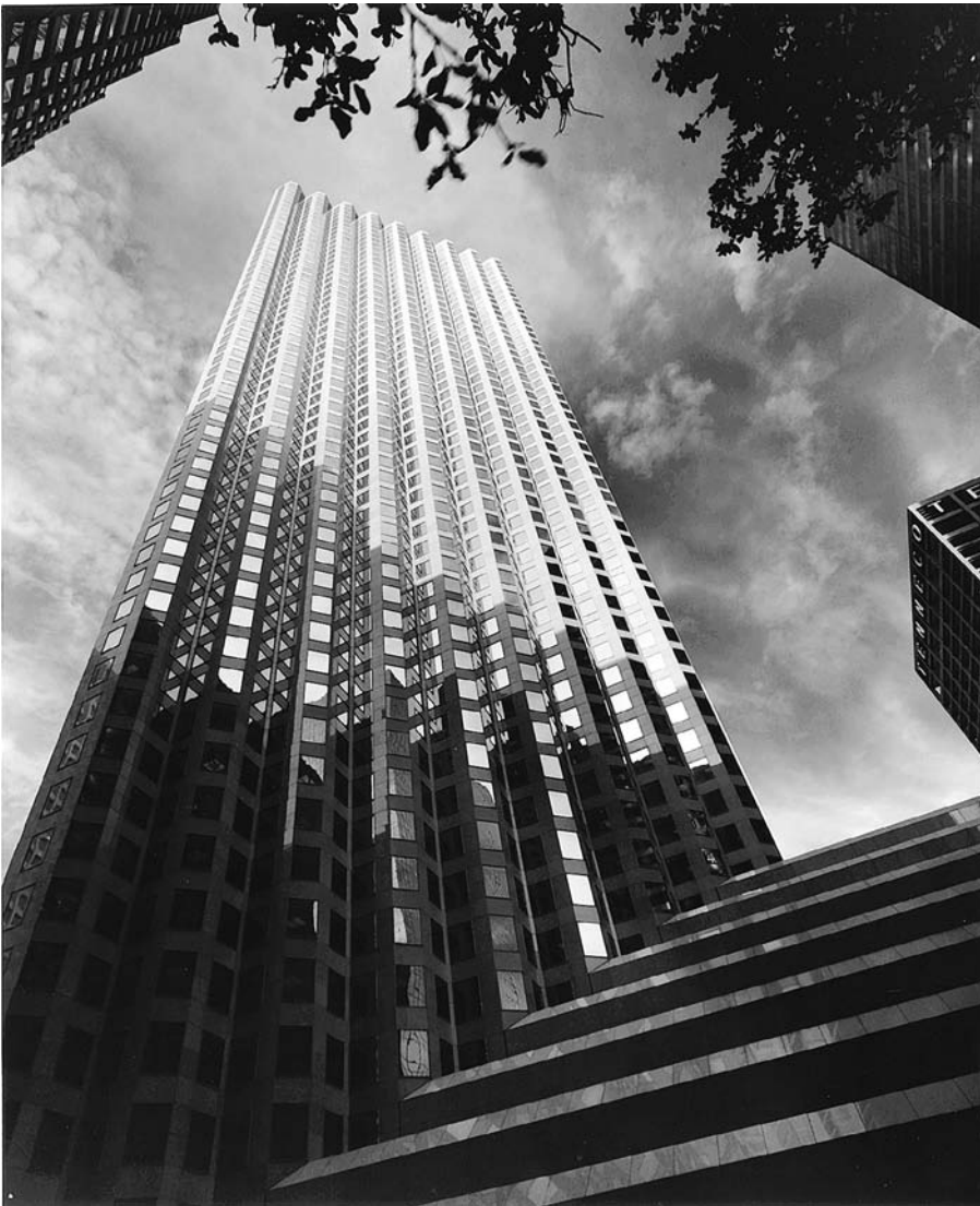
FIGURE 17.32 Discrete windows in an office building. (Architects: Skidmore, Owings and Merrill. Photo courtesy of PPG Industries)
