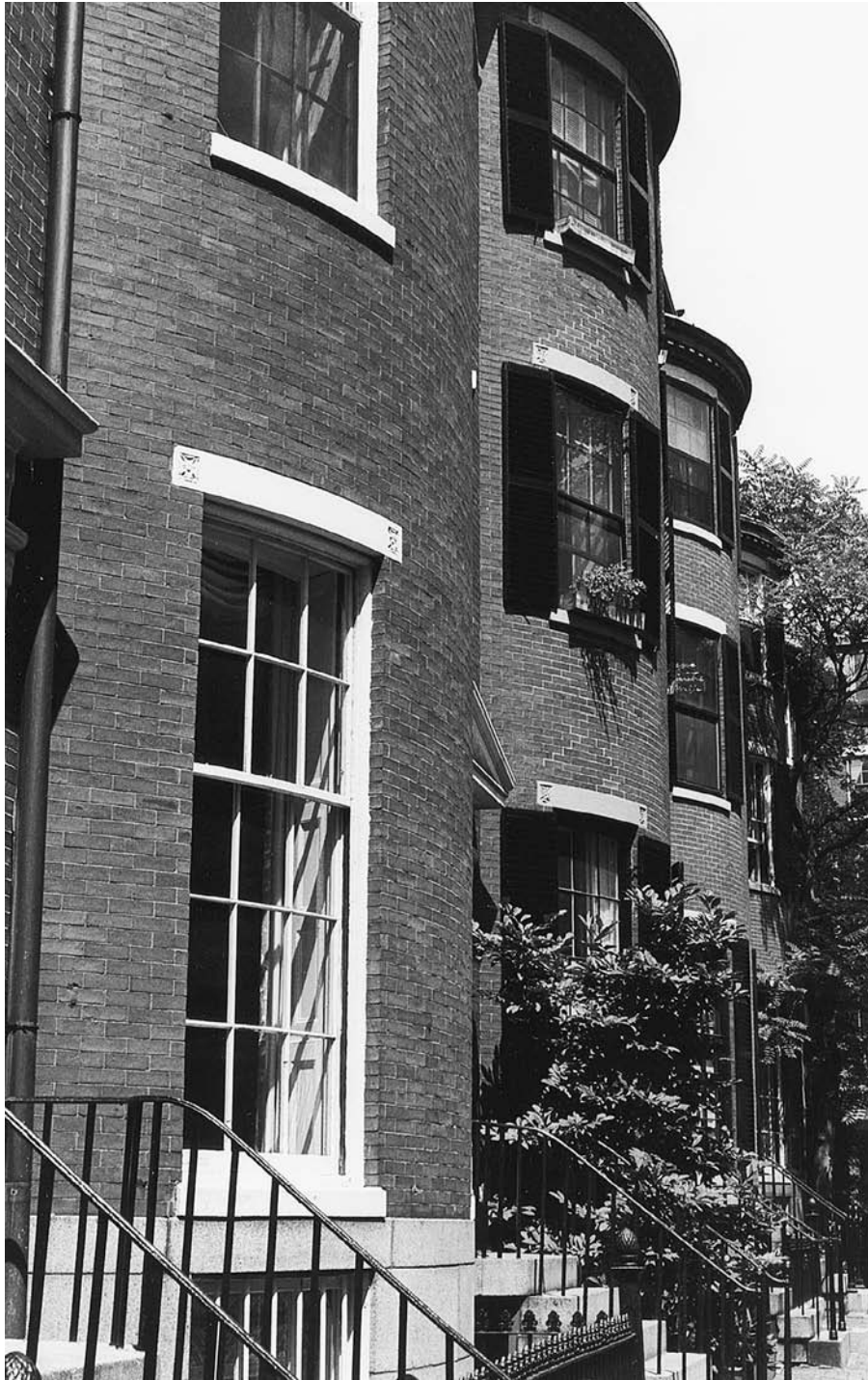
FIGURE 8.40 Cylindrical bays of brick with stone lintels front these Boston rowhouses. (Photo by the Edward Allen)
