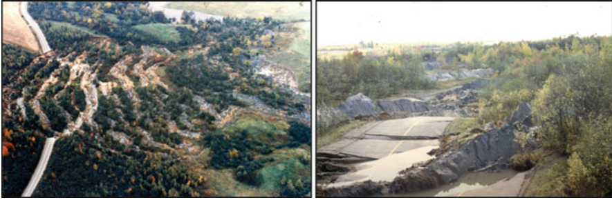
Fig. 7.8 Spread in St-Luc-de-Vincennes in 1986. Note that the plant cover and the roadway remain practically intact on top of the grabens (Source: MTQ)
