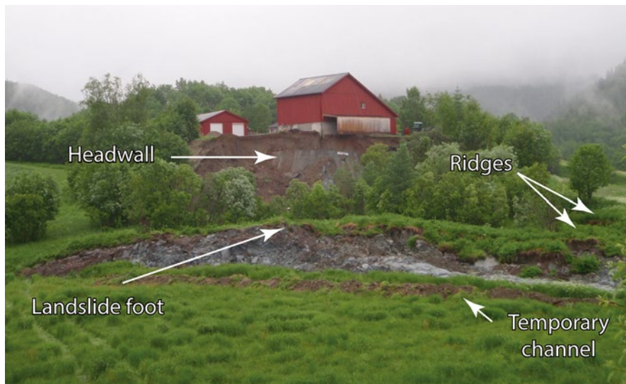
Fig. 12.2 Landslide seen from the northwest (Photo R. Moholdt)
