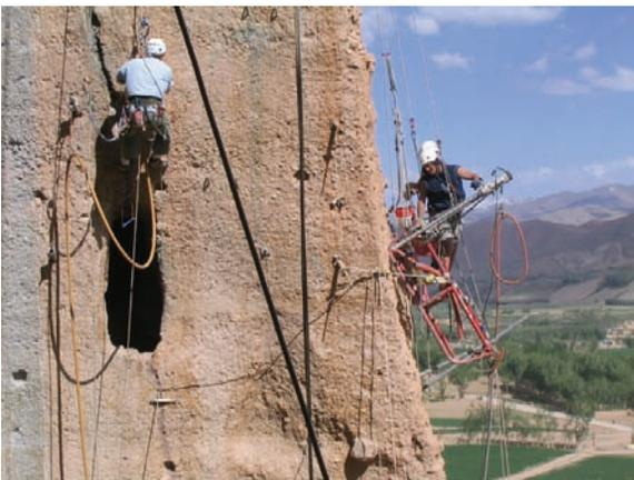
**Fig. 10.18** Execution of nails for the stabilisation of unstable blocks
