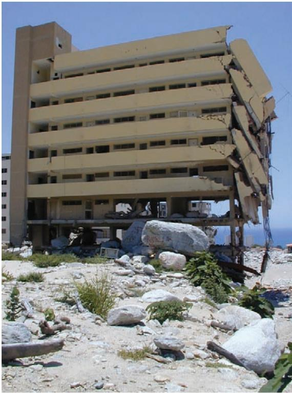
**Fig. 24.2** Apartment building in Caraballeda extensively damaged by passage of debris-flow front at least 3.5 m in height, depositing boulders (>1 m long) on second floor of structure. Note apartment building in background similarly damaged by debris flow. (Photograph by Matthew C. Larsen, USGS)
