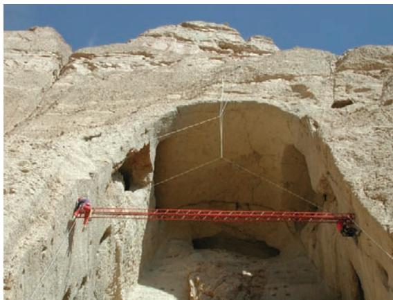
**Fig. 10.16** Installation of temporary struts. Note that, during the installation, the strut is fixed on top of the cliff, in the safe zone
