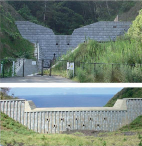
**Fig. 32.5** Concrete Check Dam (*upper*): concrete panels are pitched in the front of the dam body in order to harmonize with the surrounding landscape. Check Dam Filled with Local Sediment (*lower*): steel panels cover the dam body consisting of sediment
