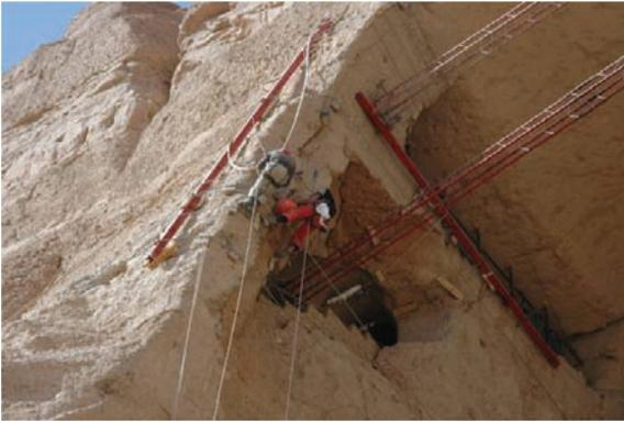
**Fig. 10.27** The temporary support necessary for a secure execution of the work in the western wall: two long iron beam replaced in the upper part of the niche, the short iron/wood struts for local support and the steel ropes
