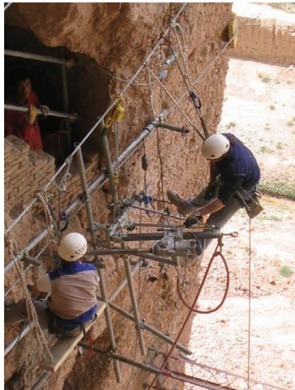
**Fig. 10.20** Execution of nails with rotary machine and diamond head, at the inner side of the niche
