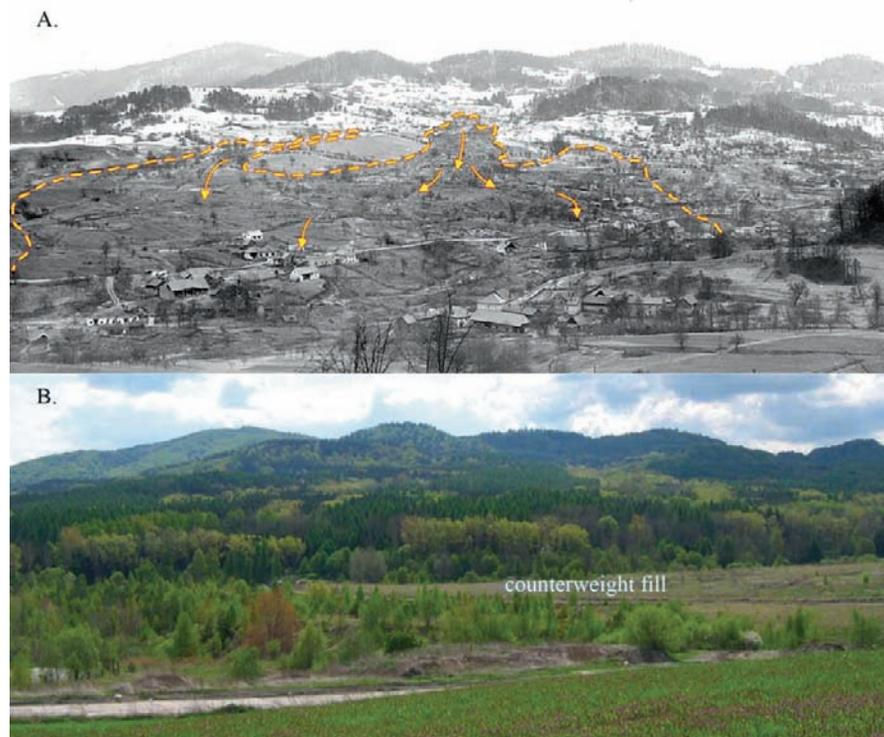
**Fig. 25.7** A view at landslide area in Handlova. A – active slide in 1961 (photo by Nemcok and Malgot), B – present state of slope with counterweight fill at the toe (April 2008)
