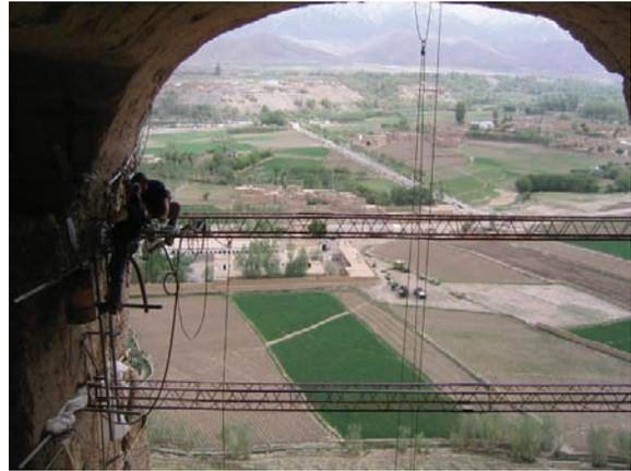
**Fig. 10.19** Execution of nails on the roof of the niche
