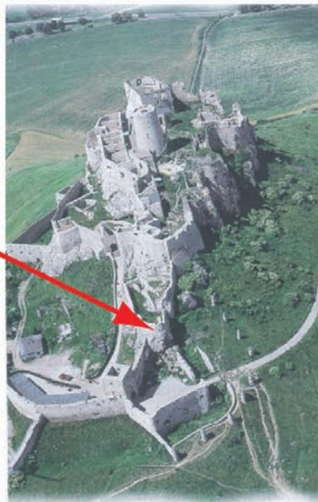
**Fig. 22.9** Spis castle with the location of the Perun's rock exhibiting displacements due to the lateral spreading of the travertine rock mass
