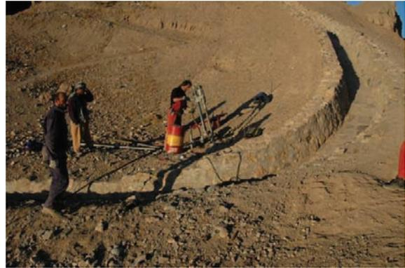
**Fig. 10.35** Detail of the grouting from the top of cliff
