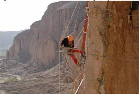
**Fig. 10.29** Drilling for nails
