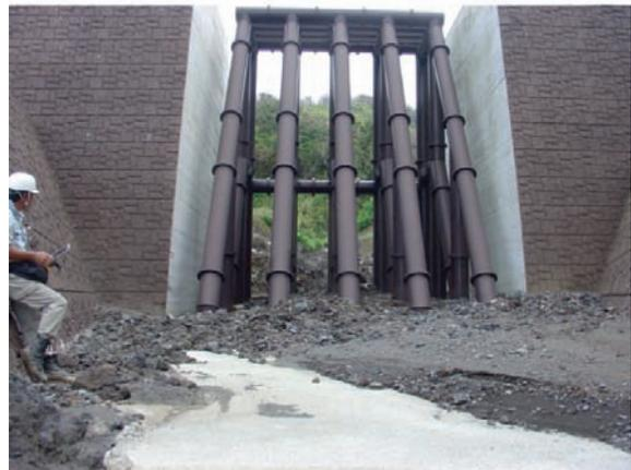
**Fig. 32.10** Open-type Check Dam: The Concrete Slit Dam (upper) is expected to have both sediment capture and retrieval functions as well as sediment discharge control function. The Steel Pipe Grid Dam is expected to catch the debris flow and discharge the captured sediment after the debris flow
