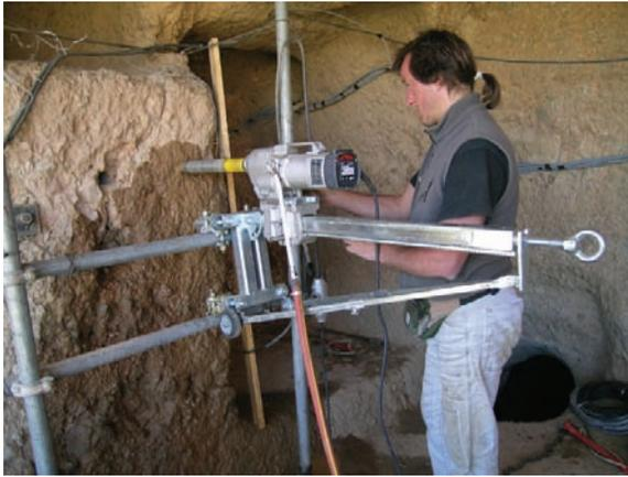
**Fig. 10.21** Detail of execution of nails from inside the caves by means of small rotary machine and diamond head
