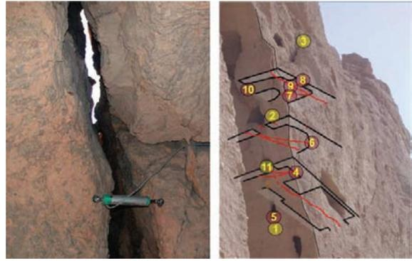
**Fig. 10.12** Distribution of the 11 sensors monitoring the cracks underlining of the most unstable block. On the right a detail of such sensors
