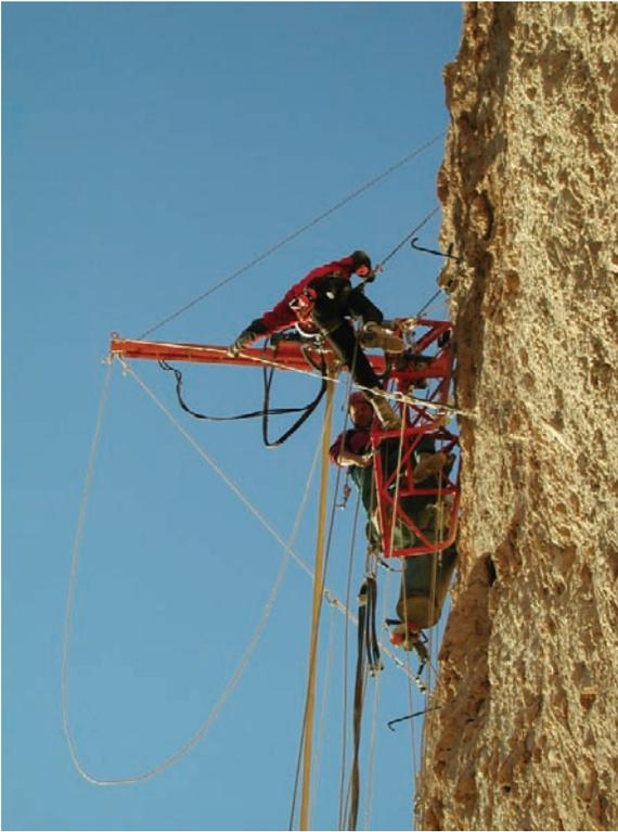
**Fig. 10.17** Final consolidation with the use of professional climbers and large rotary machine
