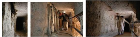
**Fig. 10.34** The large crack in the corridor on the back side of the niche before, during and after the grouting
