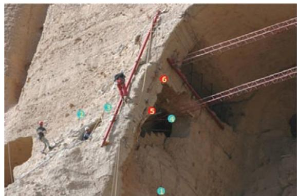
**Fig. 10.26** The location of potentiometric crack gauges for discontinuity monitoring and alarm; in green are external sensors and red are internal to the cave
