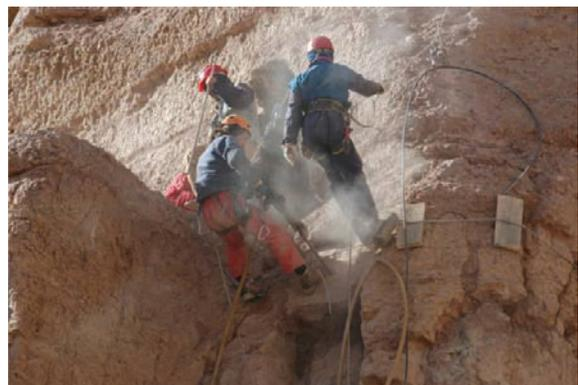
**Fig. 10.36** Drilling in the lower part of the niche
