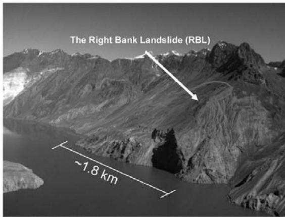
**Fig. 3.13** Active landslide on the right bank of Lake Sarez (Photo SECO, State Secr. for Economic Affairs, Switzerland)
