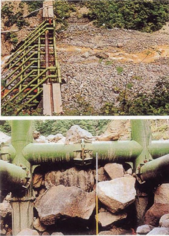
**Fig. 5.8** An example of a grid-type sabo dam, and the clogging situation at front-row of the dam
