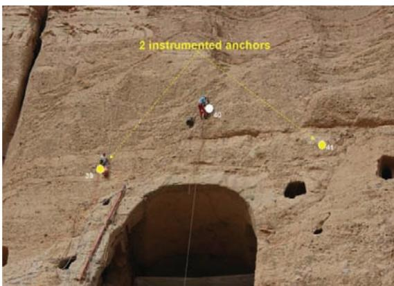
**Fig. 10.30** Position of anchors on the *top* of niche. The *yellow* ones are monitored with 10 strain gauges
