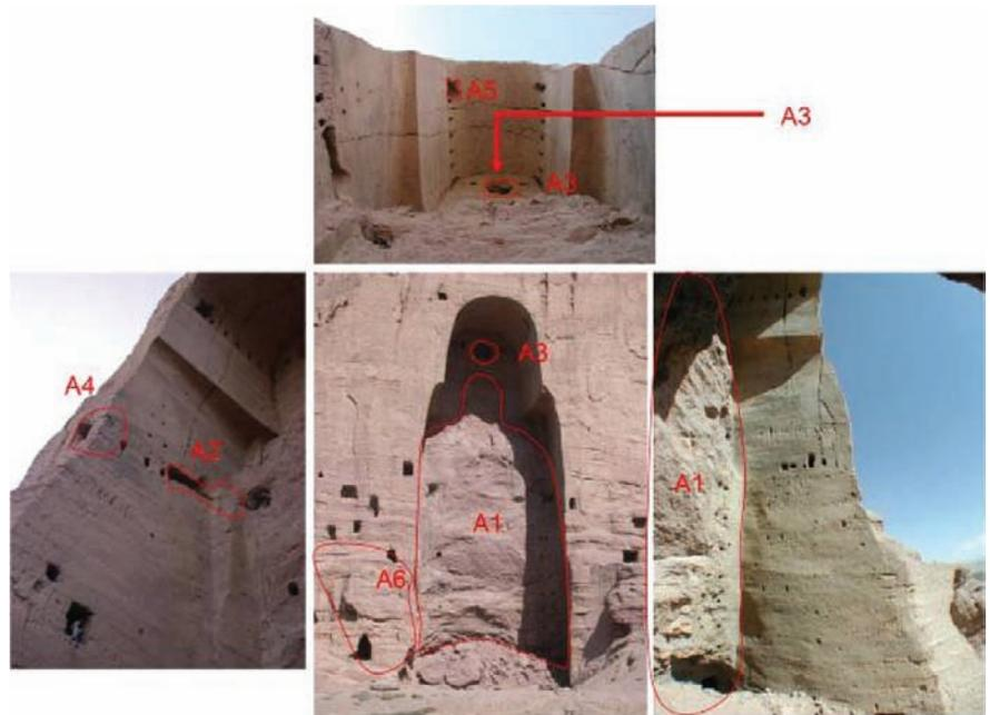
**Fig. 10.9** Identification of most critical instability areas in the West Giant Buddha niche. The *arrow* points to a serious problem inside the niche. Other important areas to secure are A4 and the *top* of A6
