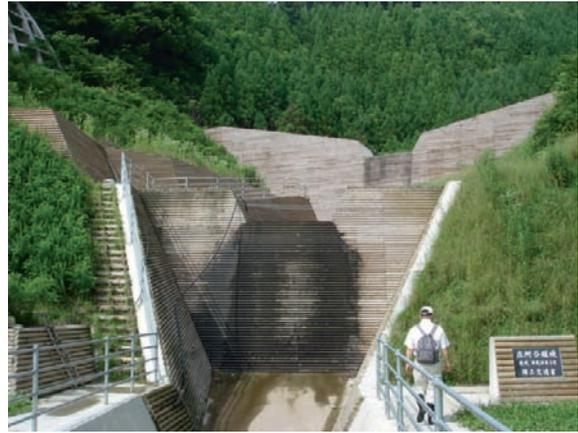
**Fig. 32.6** Check Dam with Pitching Logs: pitching logs in front of the dam body harmonize with the surrounding forest landscape
