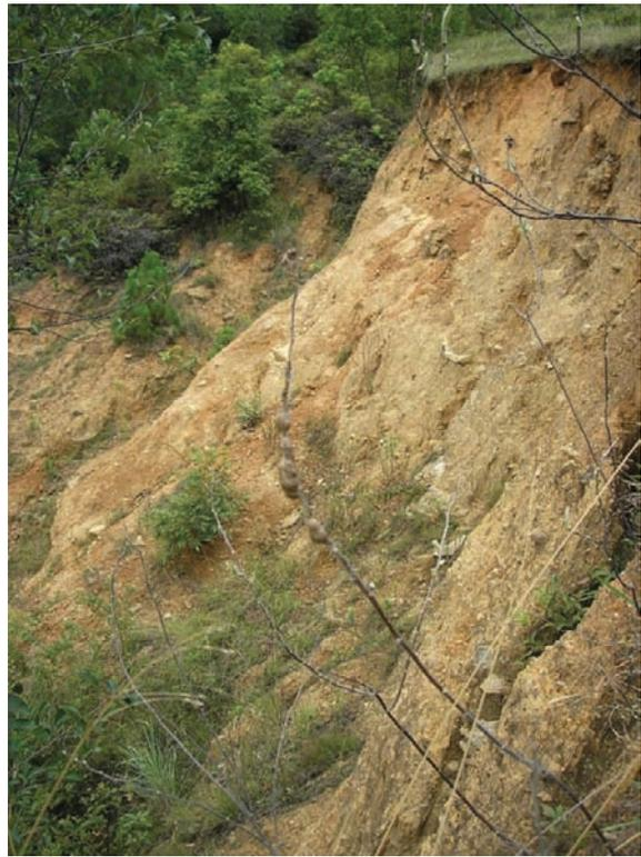
**Fig. 33.4** An example of man-made landslide process. Starting from a badly located drainage channel which has been eroded to form a gully, recurrent landsliding from the sides of the gully led to 10,000 m<sup>3</sup> soil losses within 30 years on a 0.3 ha big area of this hill of the Kathmandu valley, Nepal (picture N. Dolidon, FAO)
