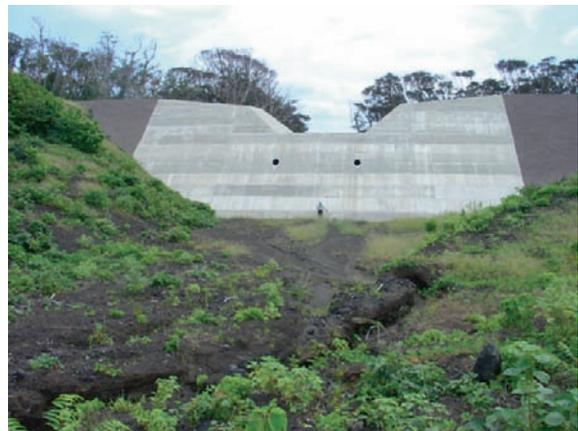
**Fig. 32.7** Check Dam Made of Soil Cement: the wings are made of soil cement and the spillway is made of concrete
