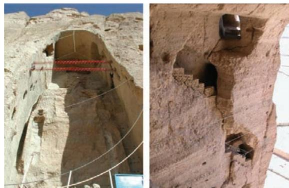
**Fig. 10.13** The temporary beam (*left*) and steel rope (*right*) for the temporary support of upper Eastern part of small Buddha
