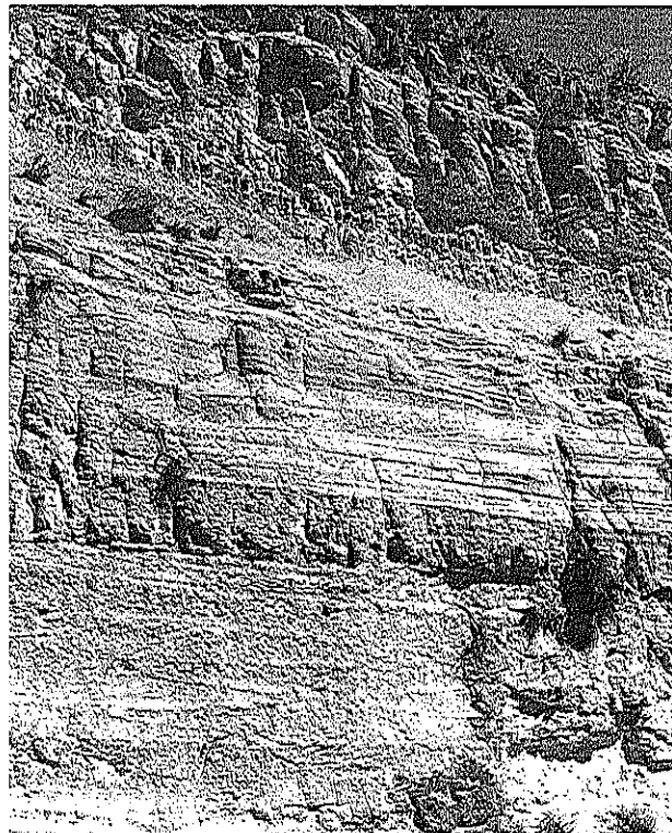
Figure CH-5.6 Pelton Park Slide. Exposure of tuffaceous soils in a road cut near the slide site. Upper beds: silty fine sandstone; lower beds: sandy, clayey silt (Photo: 1990).
