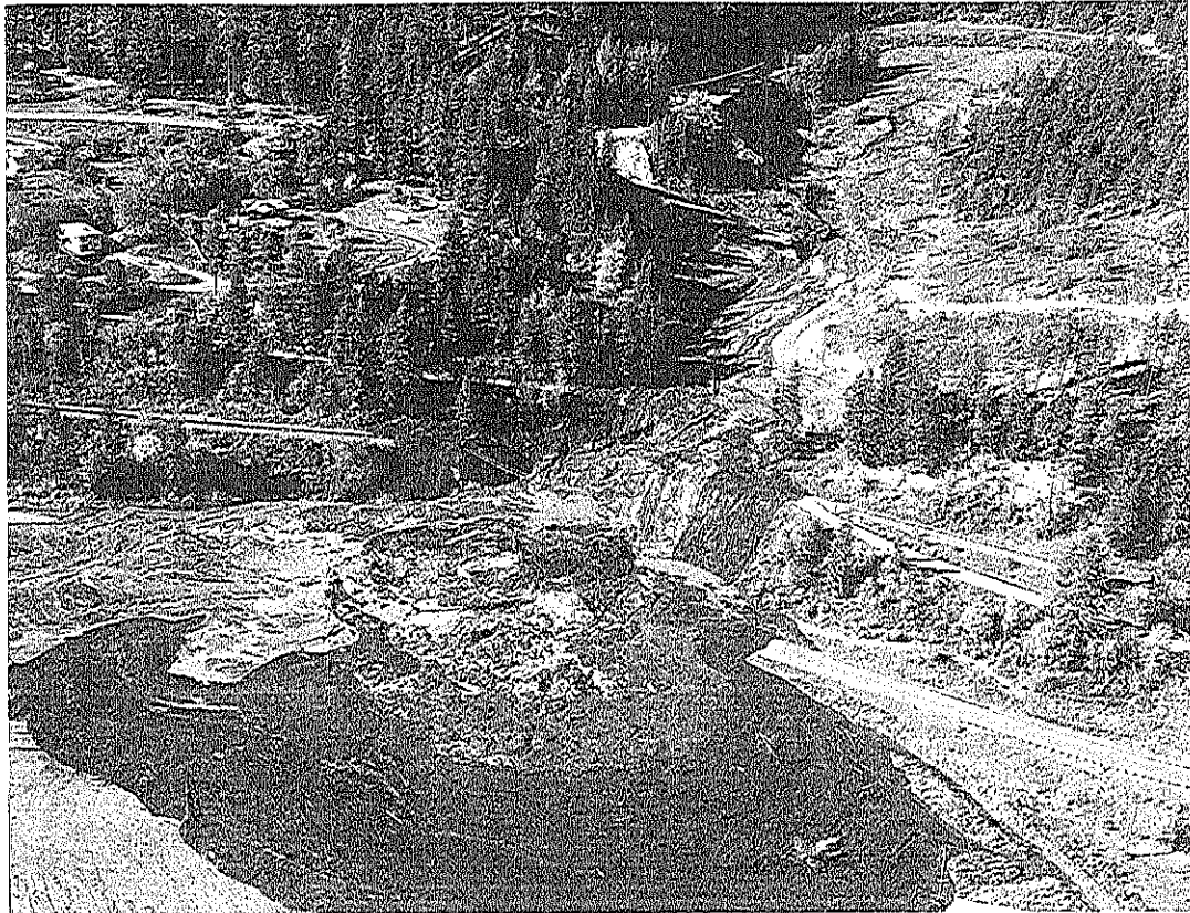
Figure CH-3.1 Bonners Ferry Slide. Oblique aerial photograph of the major flow slide aftermath, showing rupture of the railroad embankment adjacent to the flood plain (in foreground) (Photo: David Kramer).
