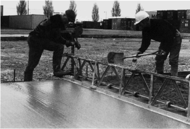
Fig. 5.53. The twin beam compactor is winched along progressively. The winch is attached to a heavy item of plant at each side of the twin beam compactor
