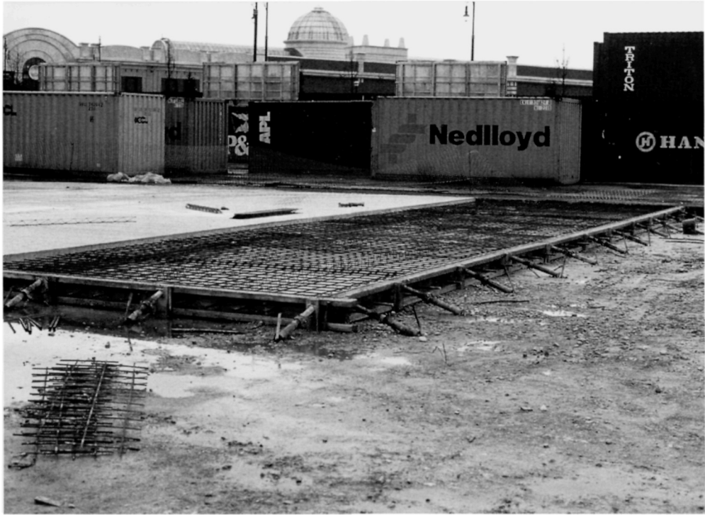
Fig. 5.43. This bay is ready for concreting
