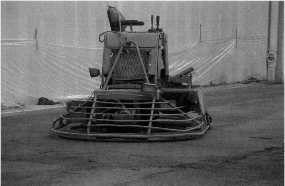
Fig. 5.19. Ride-on power trowelling machines allow greater areas to be finished and are commonly used on floors of area exceeding 500 m 2
