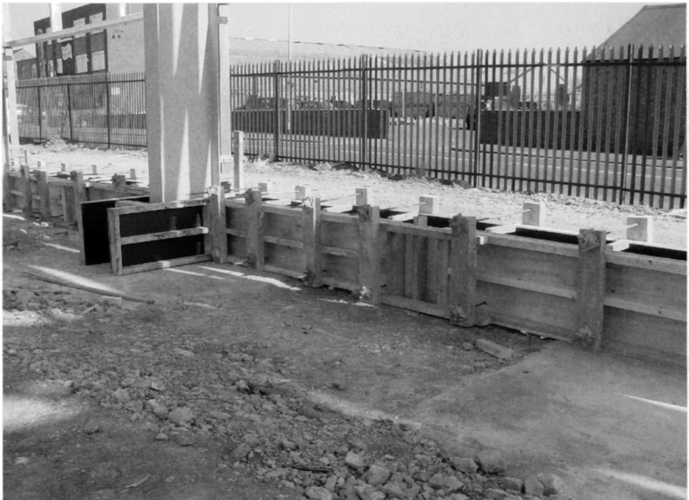
Fig. 5.92. Perimeter beam formwork positioned at the inner face of a column
