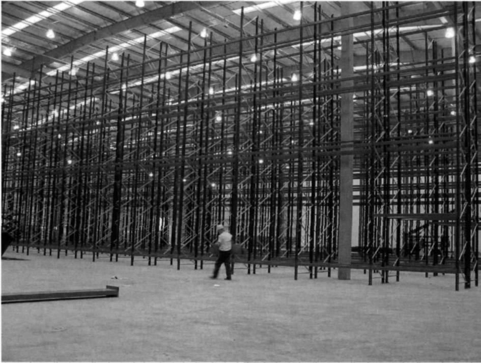
Fig. 3.35. This back-to-back high bay racking system occupies the full height of the building. It was installed in Scotland in 2002 in a distribution warehouse. Note how the system is built around the building's portal prop column. Although a loading bay is lost, the reduction in the cost of the structural steelwork makes this solution cost effective. Stability is provided by moment connections between the horizontal beams and the uprights
