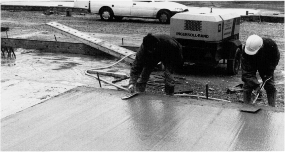
Fig. 5.45. Making good the concrete surface prior to applying the brushed finish
