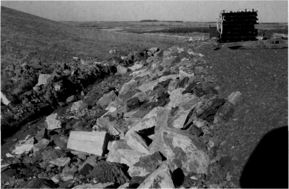
Fig. 5.62. Here the road runs over an embankment. Large mudstone boulders are used to stabilise the sides of the embankment
