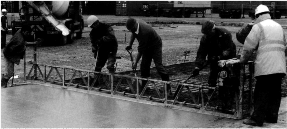
Fig. 2.1. Use of 'Razorback' enables greater widths of concrete to be placed
