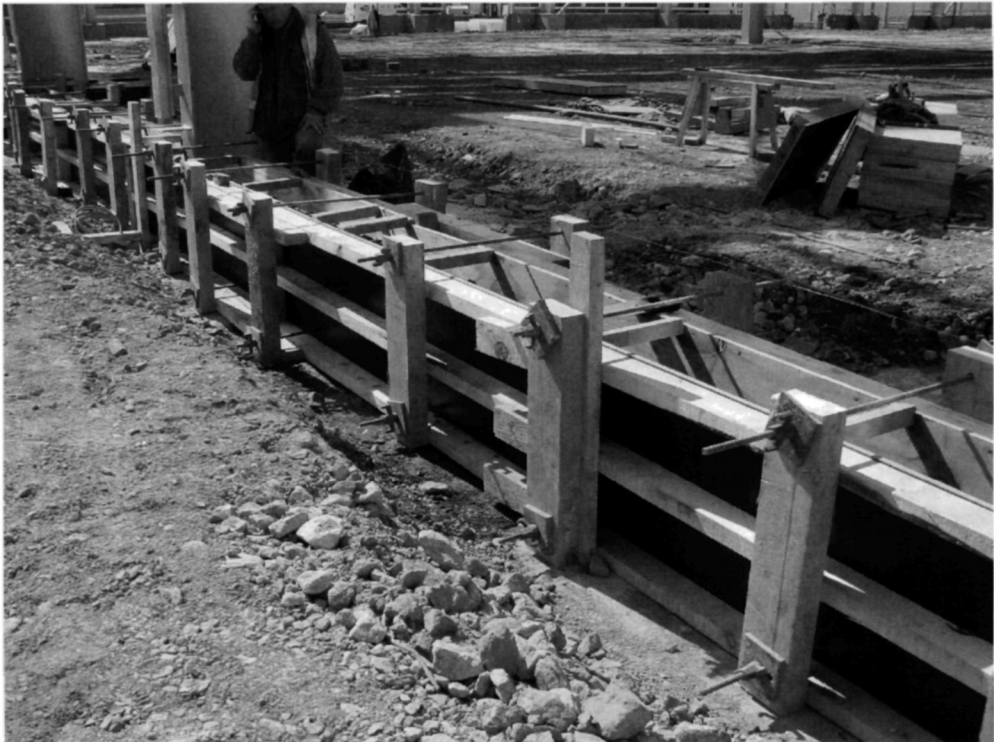
Fig. 5.88. Perimeter beam formwork in place awaiting concrete to be placed
