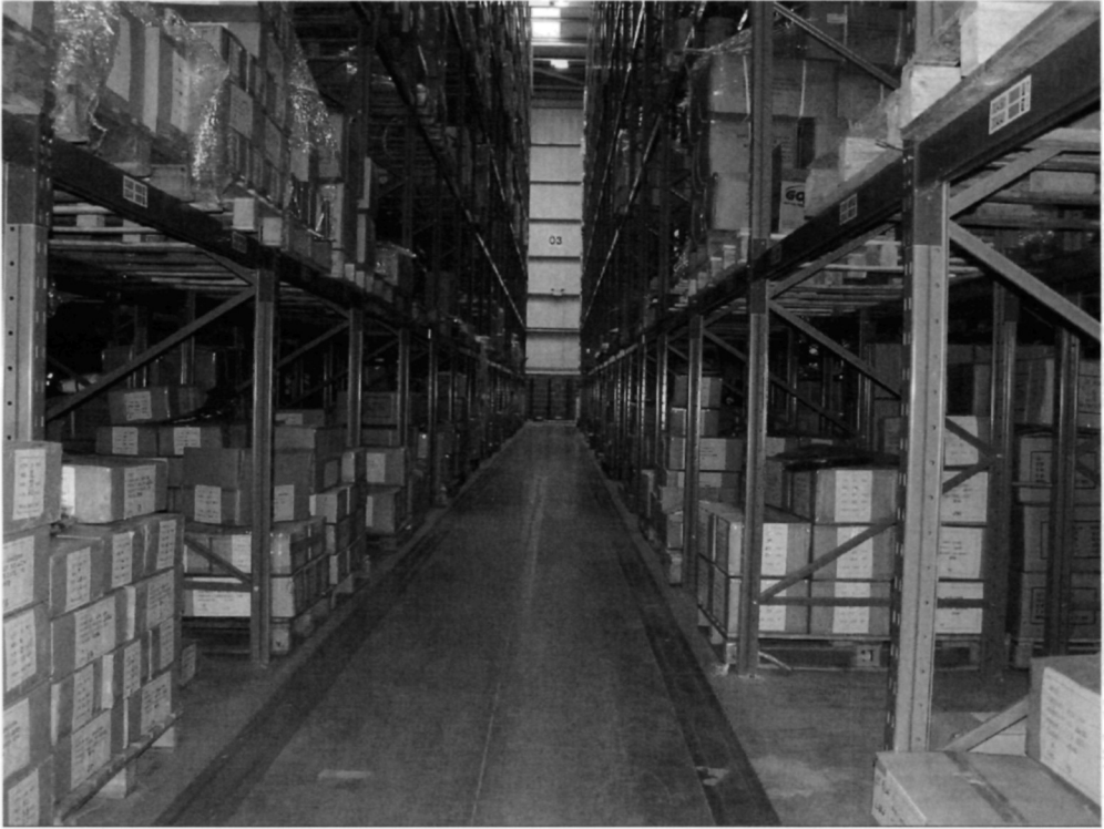
Fig. 3.41. The darker tyre tracks show how little clearance is required by a VNA truck. The line running along the centre of the aisle is where the guide wire is located. In this system, the lower pallets are stored directly on the floor, so introducing a distributed load in addition to the rack leg loads
