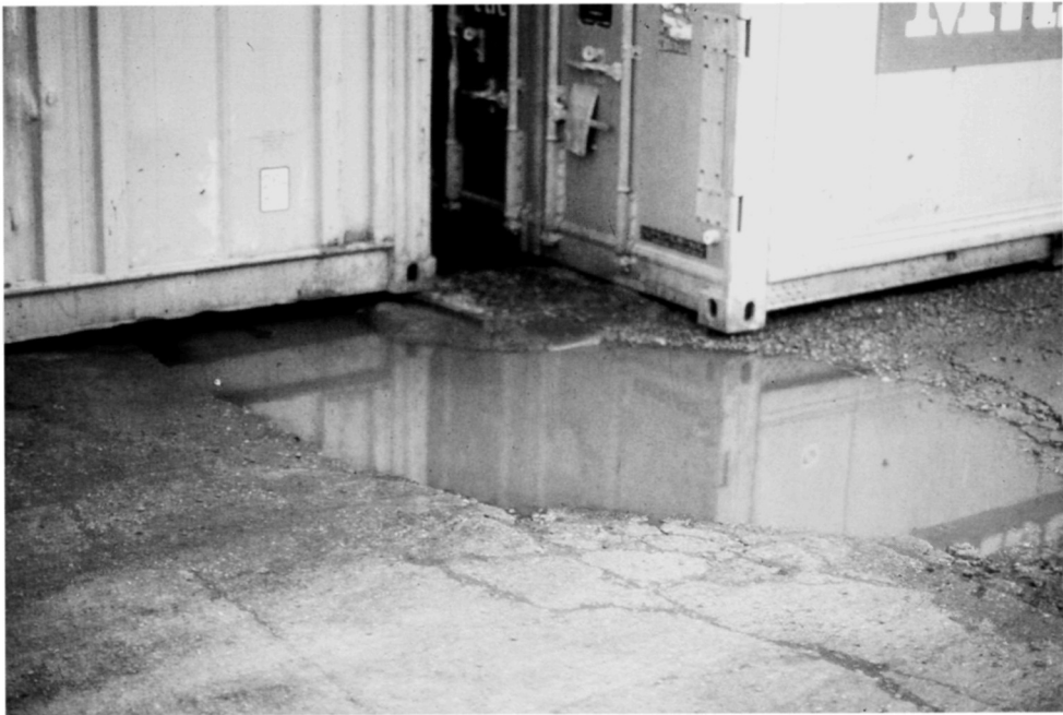
Fig. 3.7. Failure of concrete slab in vicinity of container corner castings. When the deformation exceeds 12 mm, the containers rest on their underside and the slab load becomes small. This is unacceptable from the structural capacity of the containers
