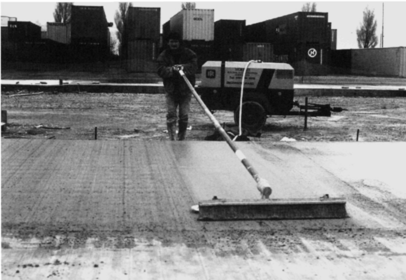
Fig. 5.52. A brushed finish is achieved by this combination float/brush device
