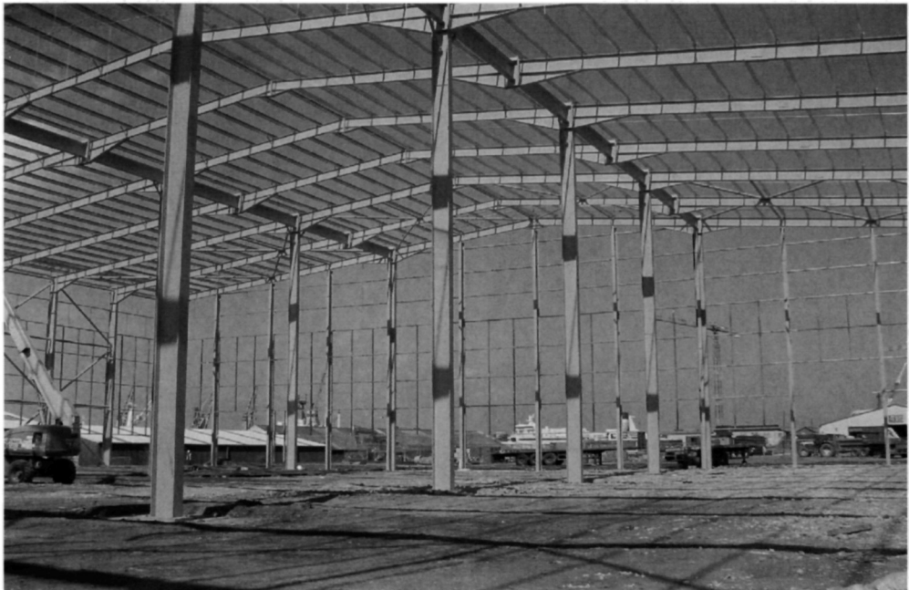
Fig. 5.86. This building at Port of Tyne's Tyne Dock is designed to accommodate a high bay racking storage system. Each portal has two props at third points and each prop has a pad foundation beneath the floor
