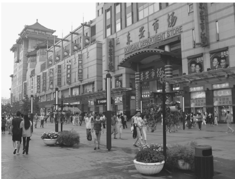
Photo 10.7. The Wang Fu Jing Shopping Center in downtown Beijing (Youqin Huang)
