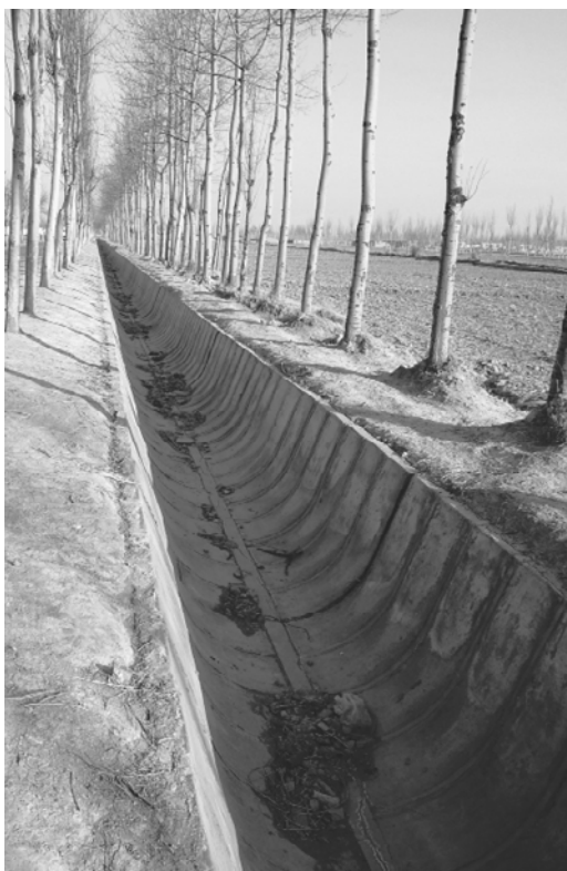
Photo 8.1. CAD-funded program in northern Ningxia Hui Autonomous Region in Northwest China that provides funds to line irrigation ditches with concrete to conserve irrigation water (2010) (Gregory Veeck)
