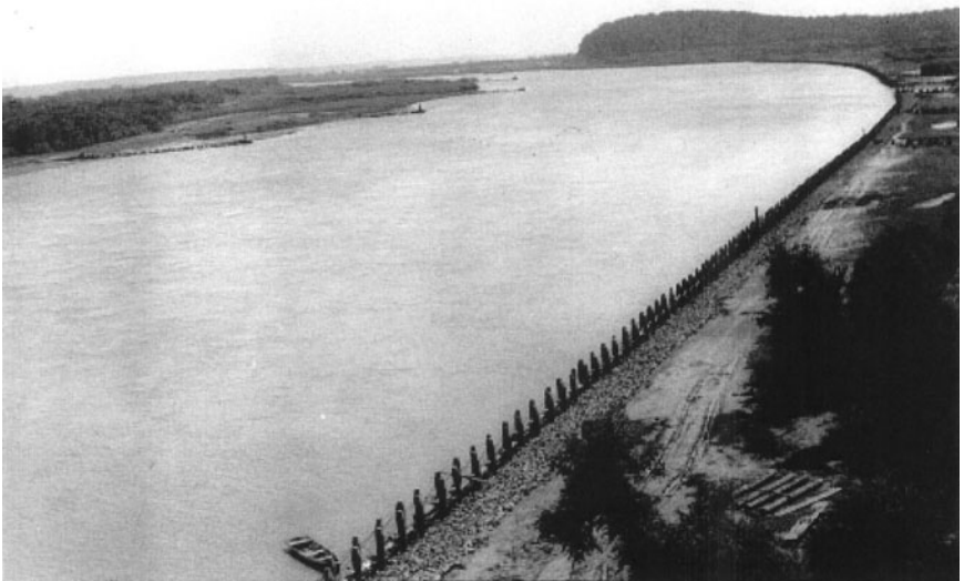
Fig. 5-22. Rock Bluff Bend, Missouri River, longitudinal stone-filled timber-pile dike added and timber-pile dikes on opposite point bar, September 1942
