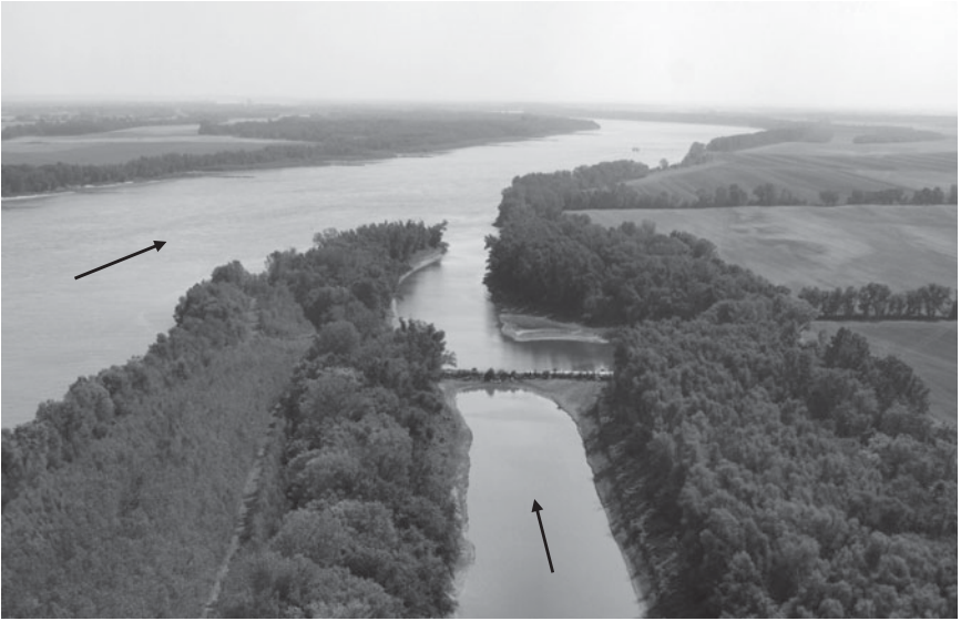
Fig. 5-13. Looking downstream at a closure dike on a secondary channel on the Mississippi River. Note the widened bankline just below the dike caused by the plunge pool when the dike is overtopped Source: USACE St. Louis District
