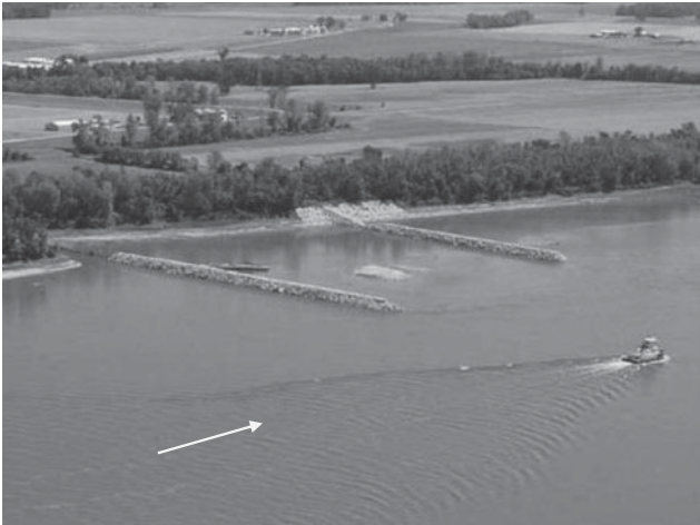
Fig. 5-7. Dike bank paving on the upper Mississippi River Source: USACE St. Louis District
