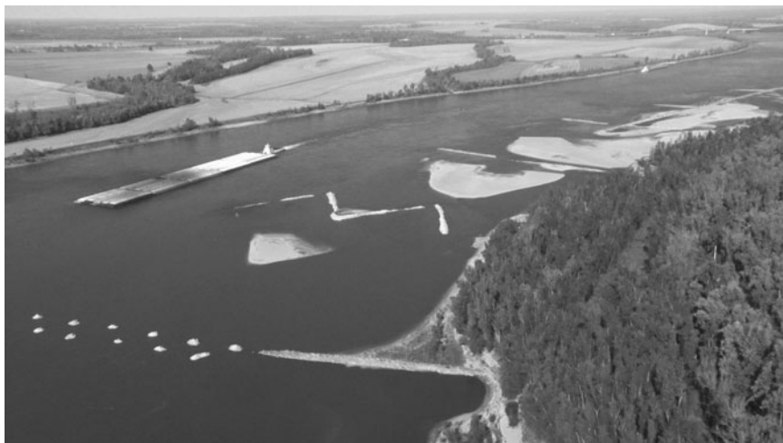
Fig. 1-1. Dikes and revetments on the Mississippi River
