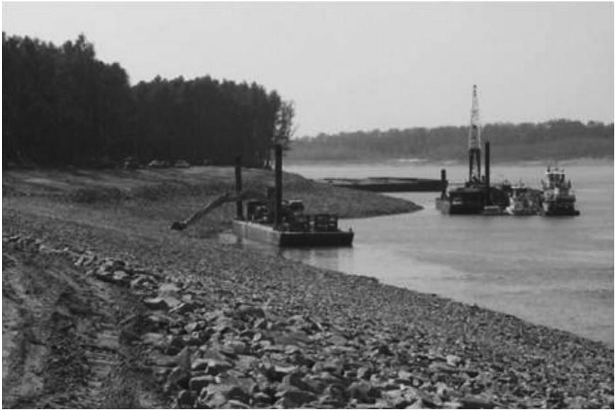
Fig. 4-2. Stone revetment protecting a Mississippi River bankline Source: USACE Vicksburg District
