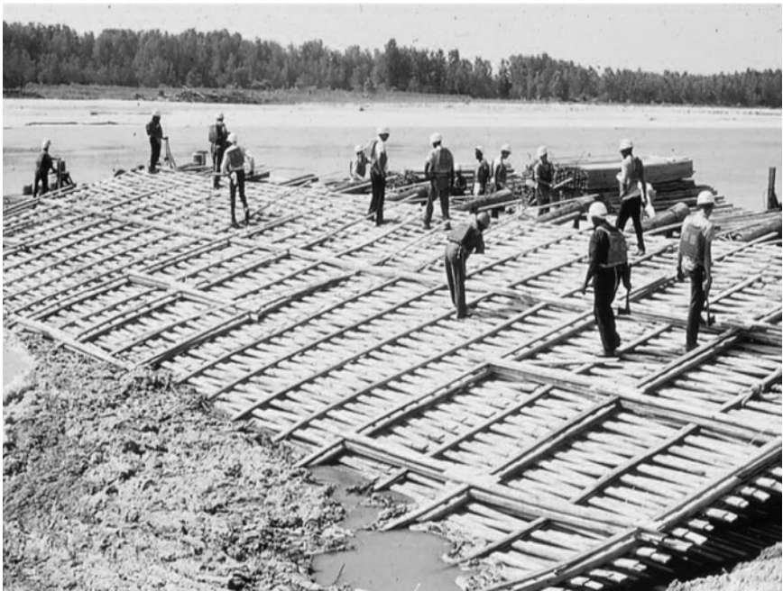
Fig. 6-3. Section of board mattress revetment under construction Source: USACE Vicksburg District
