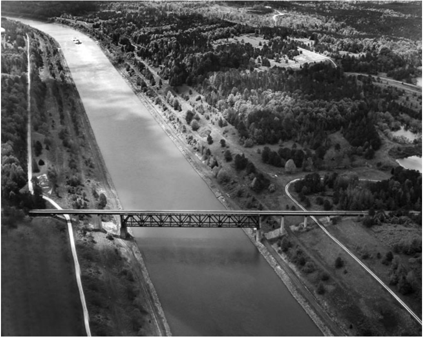
Fig. 8-1. Tennessee-Tombigbee Divide Cut Source: USACE Mobile District
