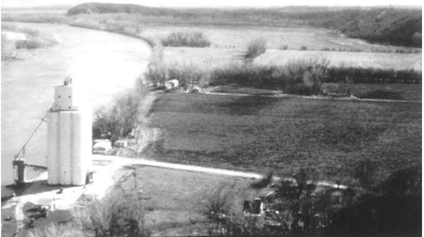
Fig. 5-24. Conditions at Rock Bluff Bend, Missouri River, March 1983 Source: USACE Omaha District
