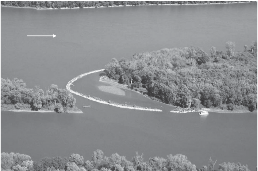
Fig. 7-4. Bullnose structure on the Mississippi River
