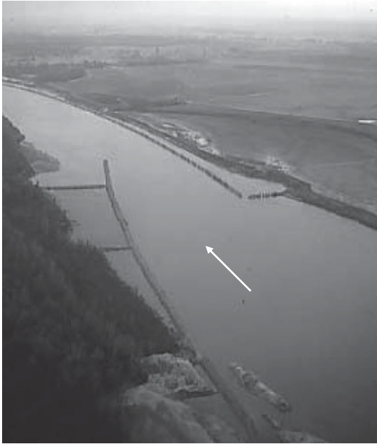
Fig. 5-14. Crain revetment kicker dike, Red River, Louisiana Source: USACE Vicksburg District
