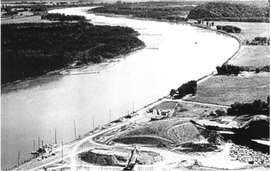
Fig. 5-23. Rock Bluff Bend, Missouri River, 1956 Source: USACE Omaha District
