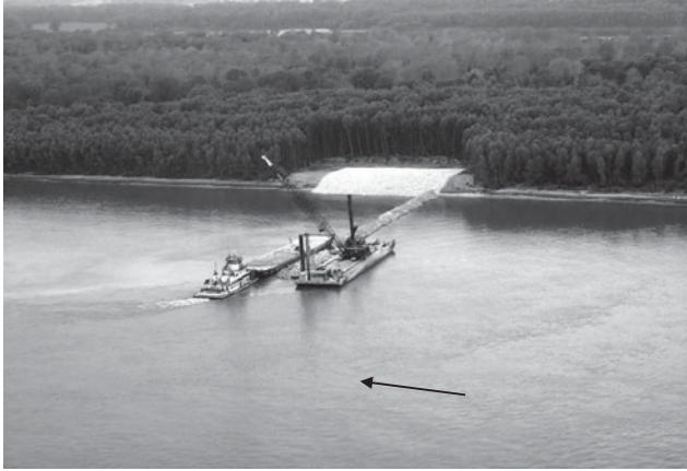
Fig. 5-8. Dike bank paving on the lower Mississippi River
