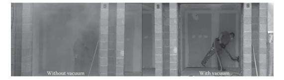
Figure 45.6 Drywall finishing without and with ventilated tool.
