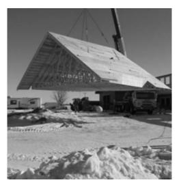
*Figure 45.2* Example of "elimination" control: roof being placed on structure, after being constructed at ground level.
