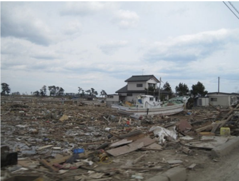
Fig. 7 Tsunami damaged area in Sendai Alluvial Flats
