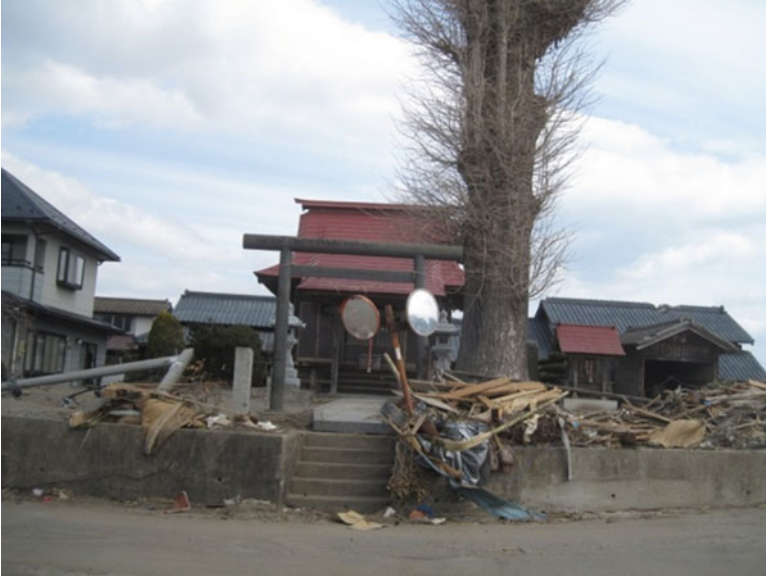
Fig. 24 Shinmei shrine survived the tsunami
