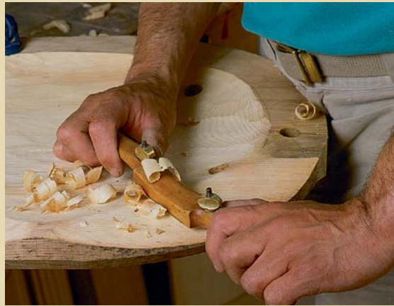
STEP 4: Remove gouges and ridges with spokeshaves.
