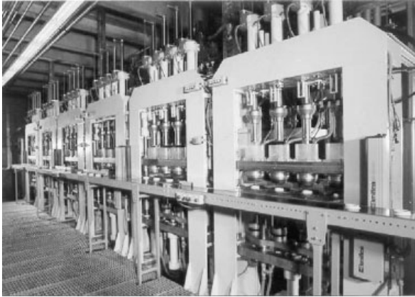
Fig. 3.11 Preform series production equipment, press side.
