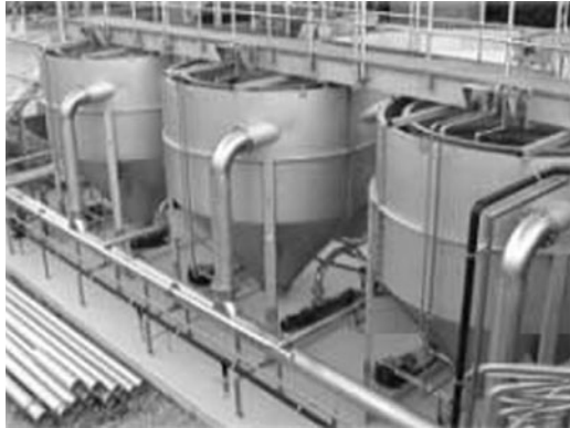
FIGURE 9.5 An example of vortex grit chambers (courtesy of Hans Huber AG).
