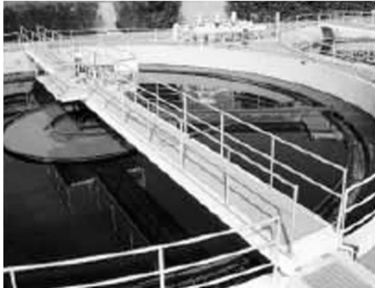
FIGURE 9.6 An example of a circular sedimentation tank (courtesy of Walker Process Equipment).
