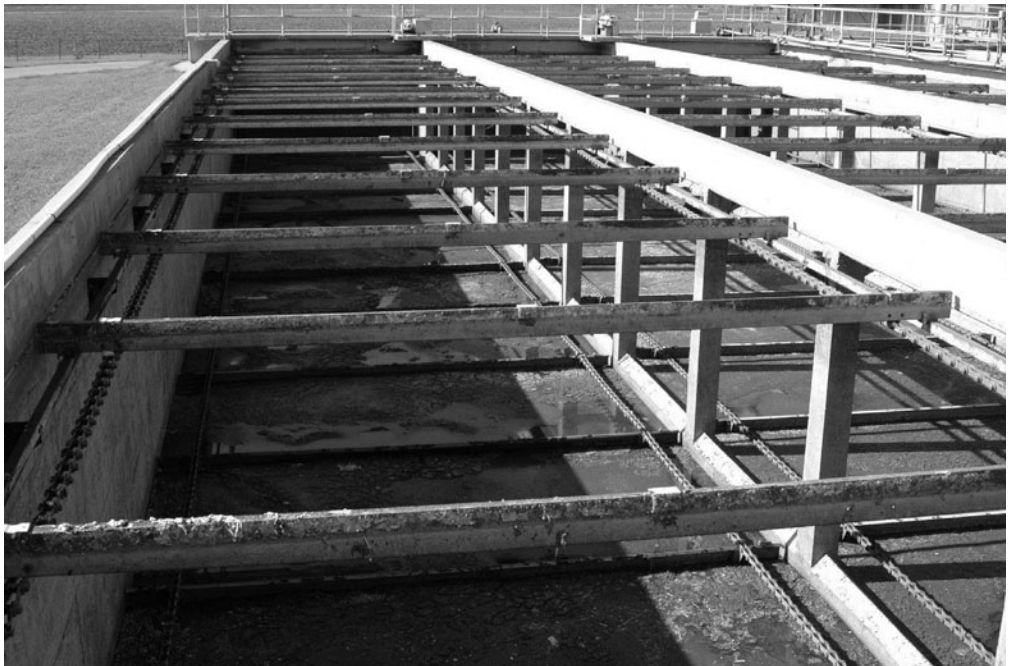
FIGURE 9.7 An example of a rectangular sedimentation tank.
