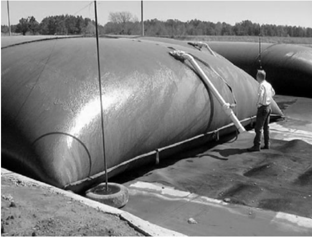
FIGURE 9.26 An example of a typical geotextile system (Geotube ® ) (courtesy of TenCate ™ Geosynthetics North).
