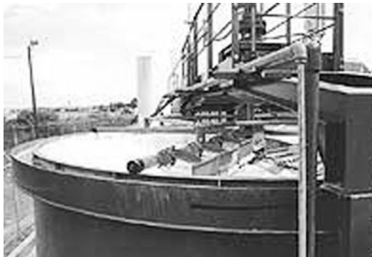
FIGURE 9.18 An example of a dissolved air flotation thickener (courtesy of Hoffland Environmental, Inc.).
