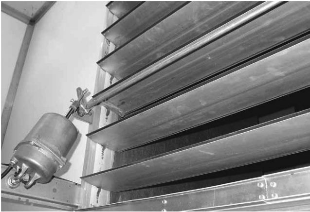
FIGURE 11.18 Pneumatic actuator on tight-seal outdoor air dampers.
