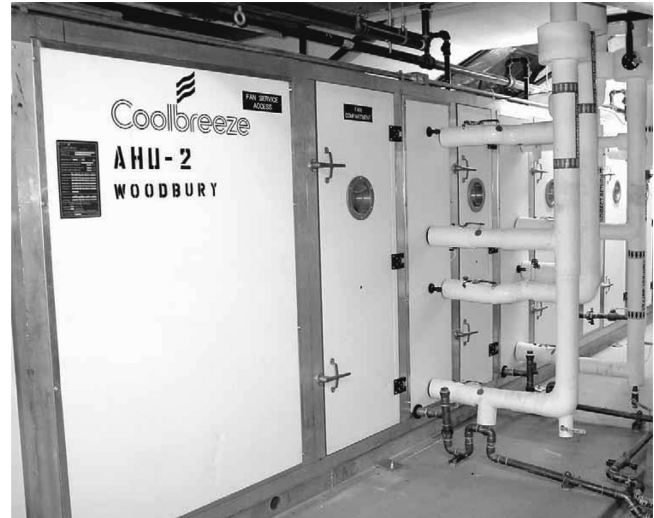
FIGURE 11.20 Large air-handler unit showing access door. (From Curtiss, P. and Breth, N., HVAC Instant Answers , McGraw-Hill, New York, 2002.)
