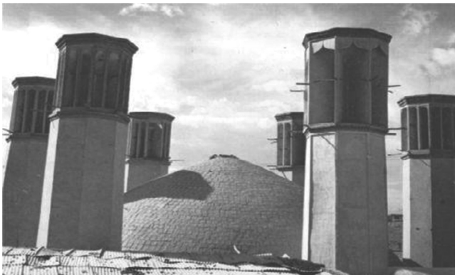
FIGURE 24.14 Photograph of downdraft wind towers.
