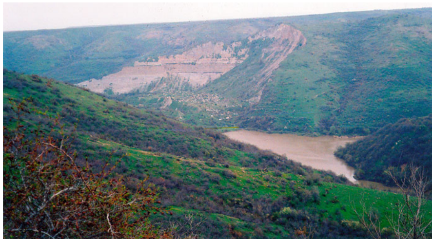
Fig. 17.2 Scar of the Gradot landslide with impounded river (Photo by B. Markoski)
