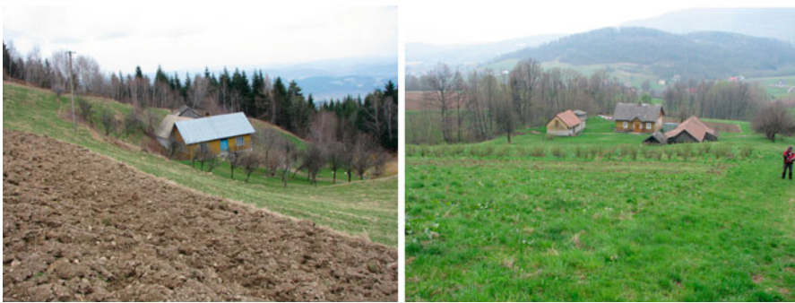
Fig. 15.5 Examples of houses located in landslide niches
