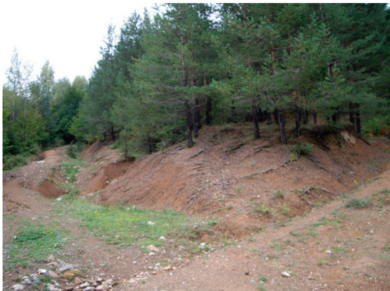
Fig. 12.2 Erosion in the basin of the Ravnitsa Stream
