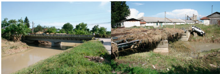
Fig. 7.13 Barriers (railway and road bridges) at Dorohoi town
