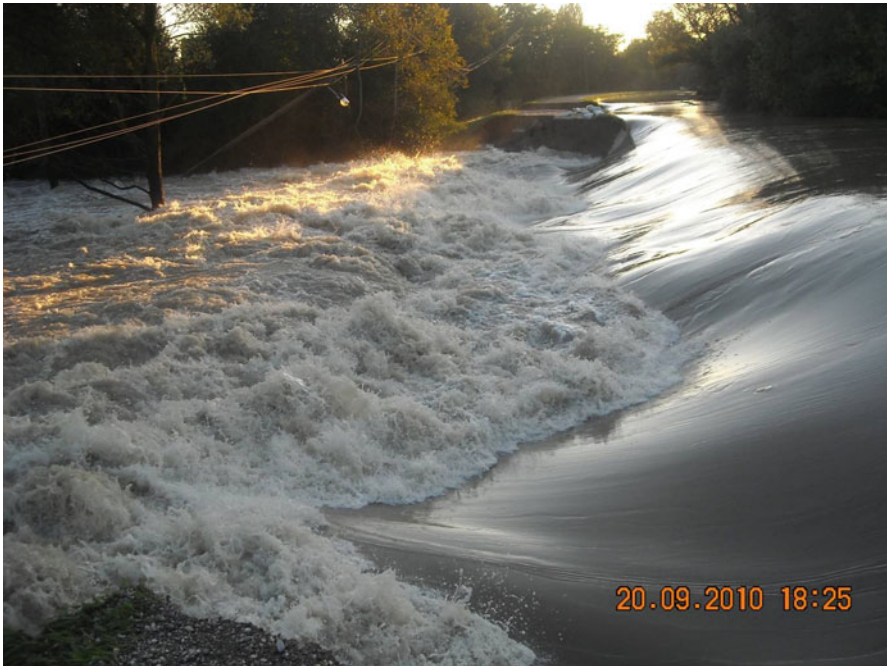
Fig. 9.3 Overflow of the right-bank Sava embankment downstream of Zagreb, 20 September 2010 ( Source: Hrvatske vode)
