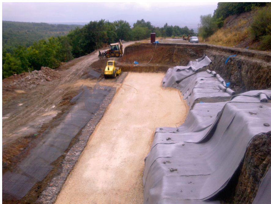
Fig. 17.7 Repairing the national road M5 between Resen and Bitola (south-western Macedonia): unloading the slided mass, stabilization with gabions, and reinforced soil surface (Photo by A. Strašeski)
