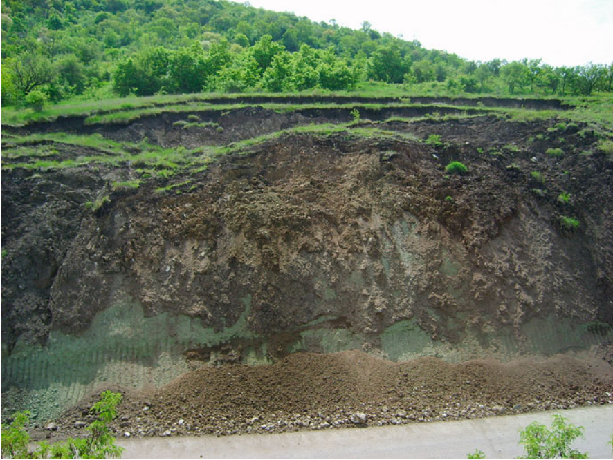
Fig. 17.9 The Stracin landslide on the international road Corridor 8, highly active in early 2010 (Photo by I. Milevski)
