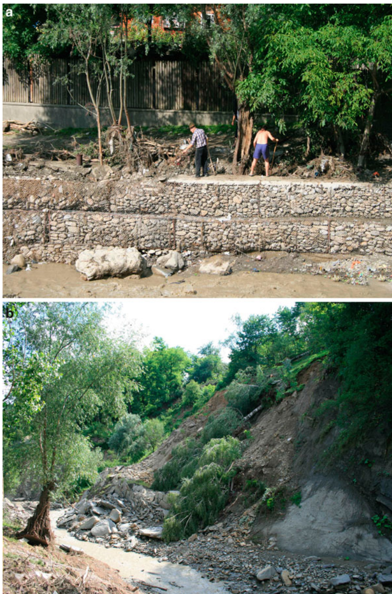
Fig. 16.5 The flash flood of July 2010 on the Drajna catchment (Cerașu, Prahova County) overpassed bank protections by 2 m (a), damaging 18 households and causing numerous riparian landslides (b) through lateral erosion (Photo by M. Micu)
