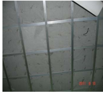
Figure 5 (c). Under deck retrofitting
