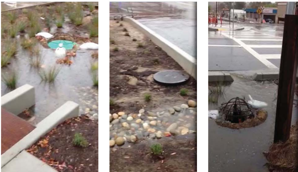
Figure 6. Three Examples of Urban First Flush Drainage into Bioretention Swale – 21 st Street, Paso Robles, California.
