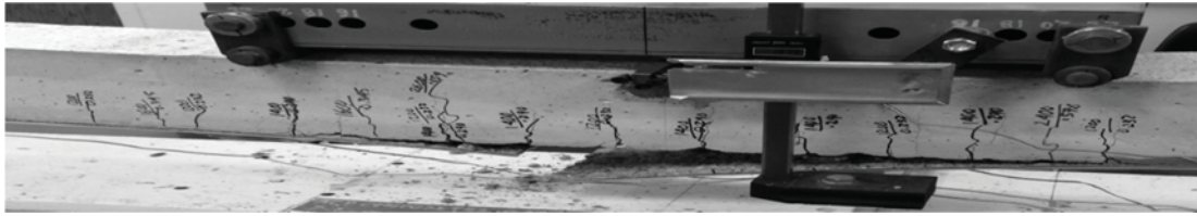
Figure 3. Observed experimental plate rupture failure of GFRP reinforced beam.
