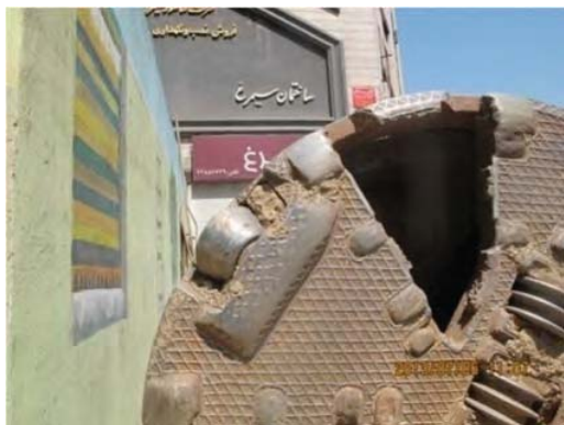
Figure 17-a- Damage of Cutter head in facing boulders
