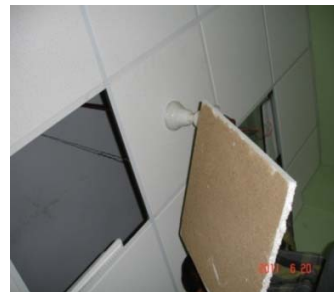
Figure 6 (c). Under deck retrofitting
