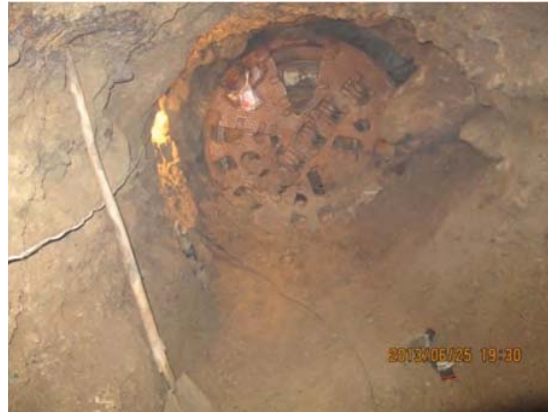
Figure 15-crossing machine through handmade tunnel
