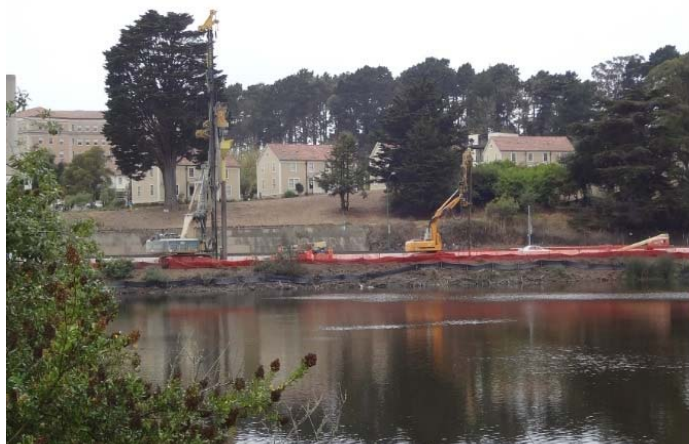
Figure 6. General view of construction site.
