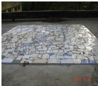
Figure 6 (b). Over deck retrofitting
