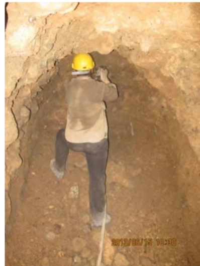
Figure 12-b-Excavation by hand through huge boulders
