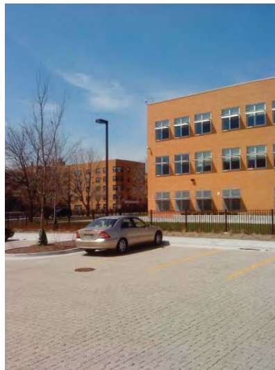
Figure 4: Permeable Paver Parking Lot at Powell Elementary School
