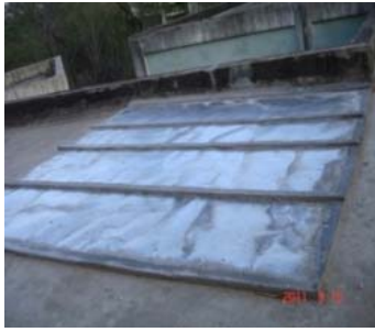
Figure 5 (b). Over deck retrofitting
