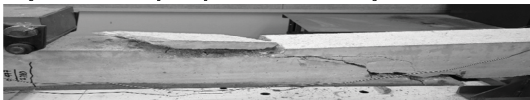
Figure 2. Main shear-flexure crack and RC cover failure for CFRP beams.
