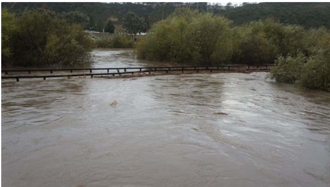
Figure 3: Bridge 248.7 over Las Penasquitos Creek, December 2010 (Photo credit: NCTD MOW)
