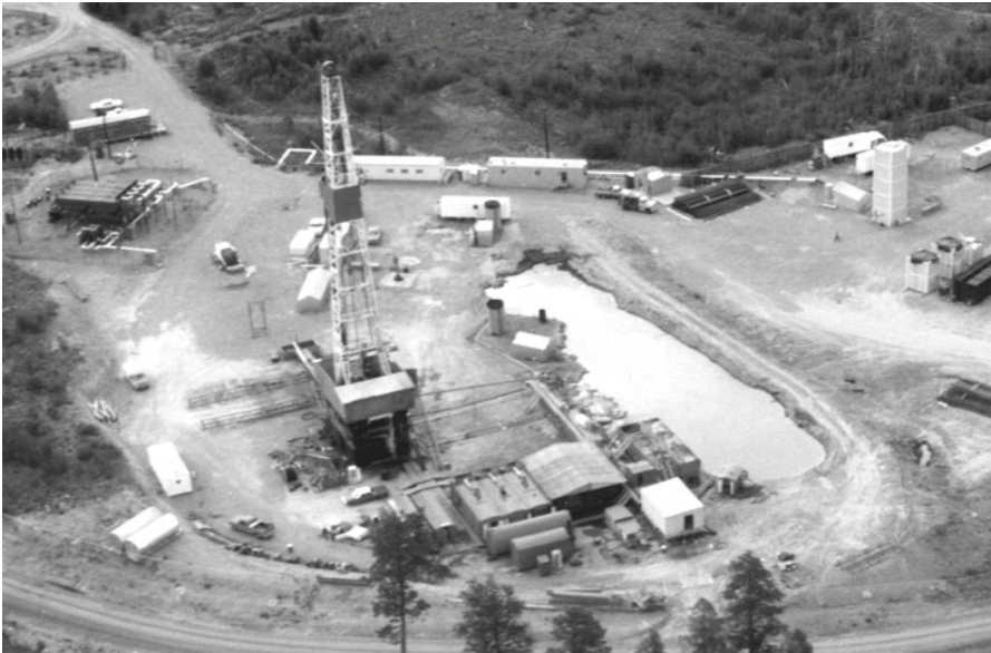
Fig. 5-3. The EE-2 drilling location, viewed to the east, in the spring of 1979. The heat exchanger, the tower over GT-2, and the numerous trailers, tanks, and pipelines associated with the first two flow tests of the Phase I reservoir are visible behind and to the right of EE-2.
