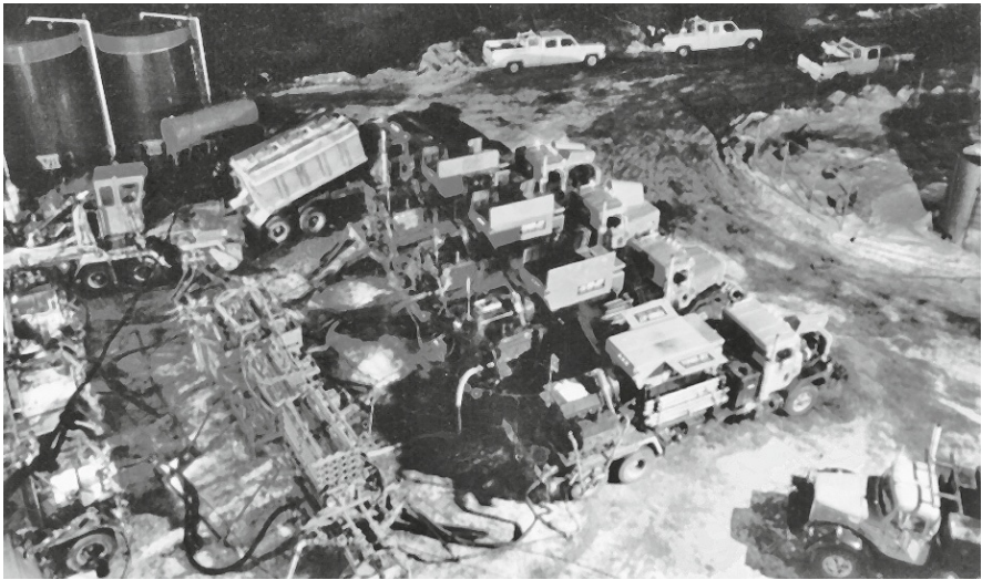
Fig. 6-19. Dowell equipment deployed around EE-2 for the MHF Test. Source: HDR Project photo archives
