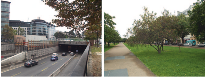
Fig. 10 Coverage of A1 highway and its transformation in Boulevard Wilson, with a large median green space; photograph Mihaela Negulescu
