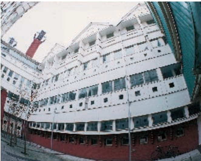
Figure 1.13 De Montfort Engineering Building, Leicester, maximises daylight by incorporating high windows; light shelves reduce glare. Smaller windows provide a view for individuals sitting at the workstations
