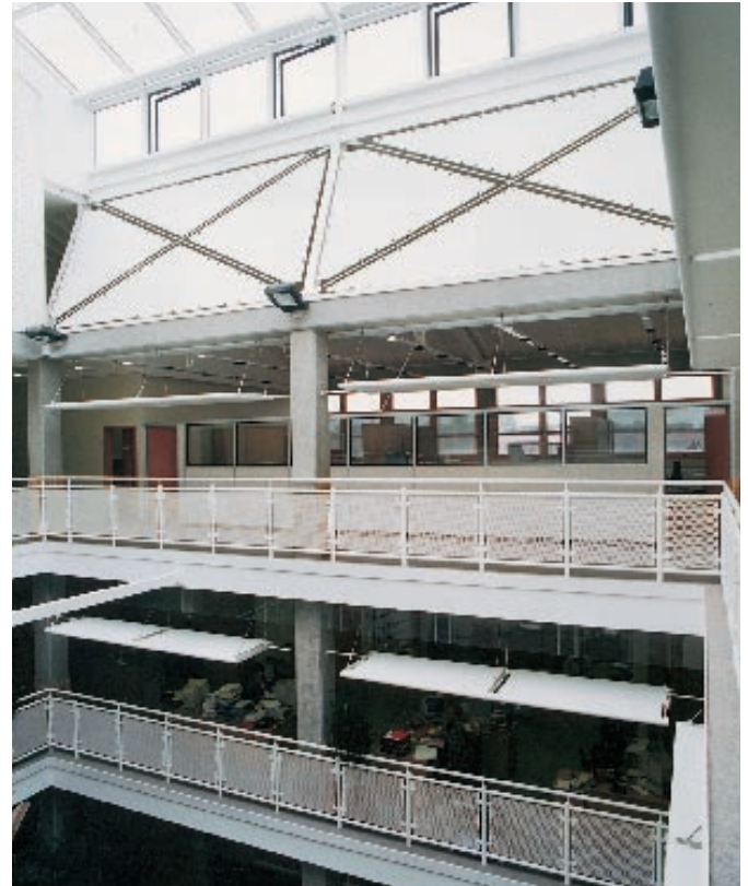
Figure 1.15 The Queens Building, Anglia Polytechnic, has light shelves on the outside façade and inside the atrium
