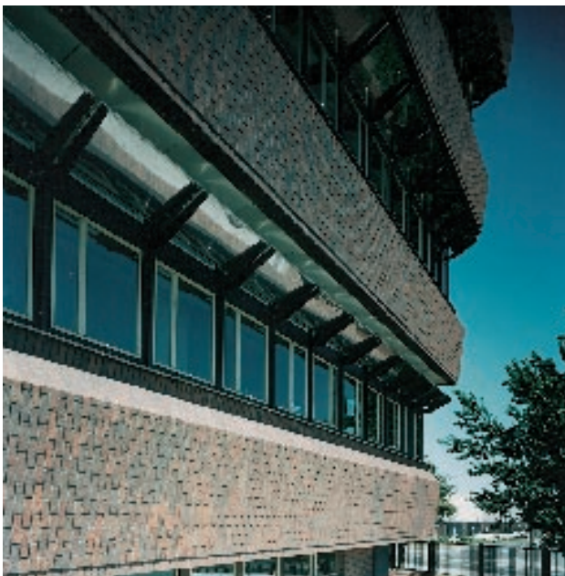
Figure 2.49 External and internal light shelves on the South Staffordshire Water Company office building. Note the sunlight reflected off the ceiling
