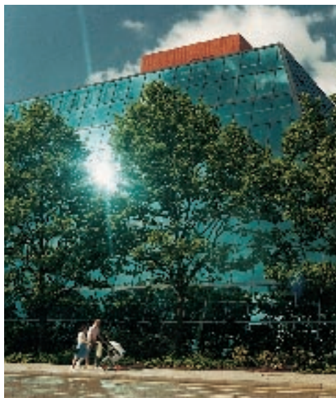
Figure 2.44 Solar reflection from a sloping façade in Aylesbury
