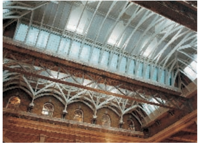
Figure 2.48 Prismatic glazing at the Billingsgate building, London, a rooflit dealing space
