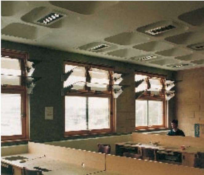
Figure 1.15 The Queens Building, Anglia Polytechnic, has light shelves on the outside façade and inside the atrium
