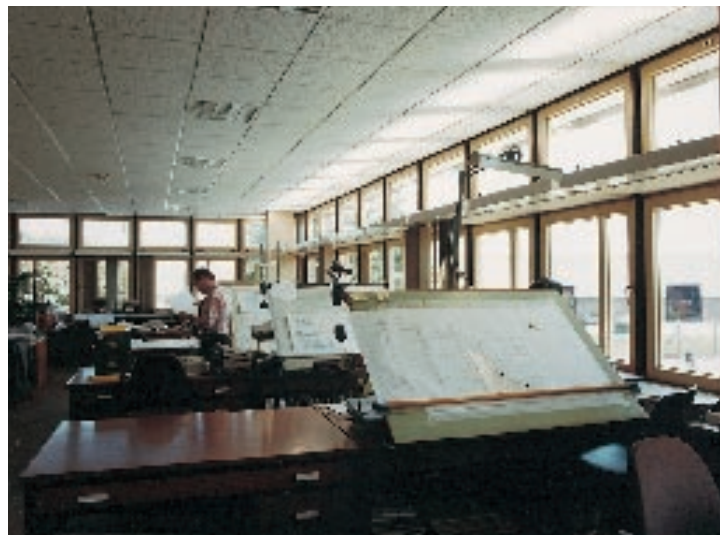
Figure 2.49 External and internal light shelves on the South Staffordshire Water Company office building. Note the sunlight reflected off the ceiling
