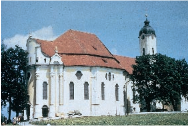
Figure 1.14 Die Weiss, typical of the Baroque churches of Southern Germany where daylight enters from windows concealed from normal points of view, focusing light on to the altar
