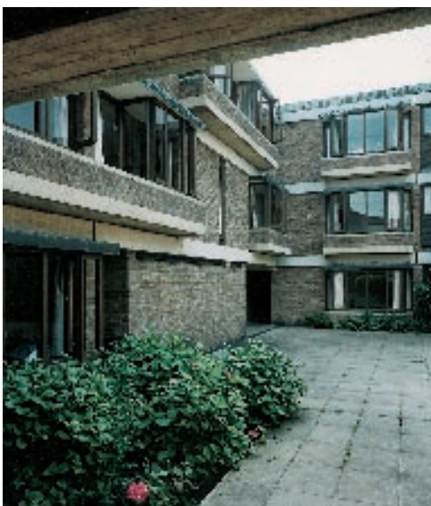
Figure 2.25 Rooms looking out from the internal corners of courtyards can often be gloomy and lack privacy
