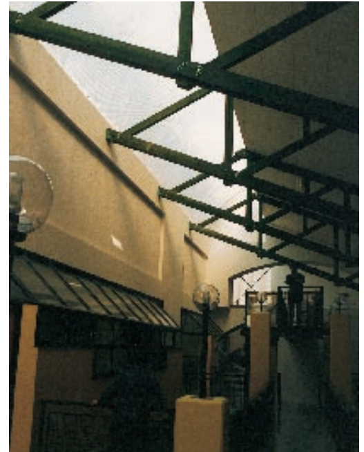
Figure 2.18 One of the linear atria between the classrooms
