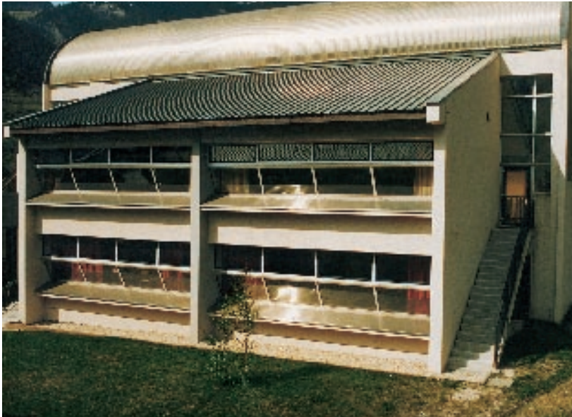
Figure 2.17 Reflective window sills provide extra light on the south-facing windows
