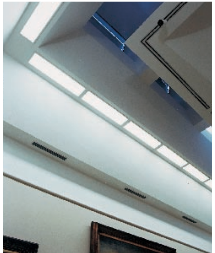
Figure 2.52 Looking up into the light scoop
