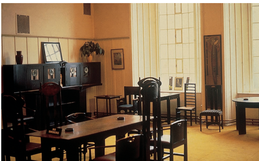
Figure 1.3 Sunlight entering the Director's Room, Glasgow Museum of Art. The windows in this sidelit room have low sills and high heads to give good daylight distribution, while the splayed reveals reduce the contrast between the exterior and the window wall
