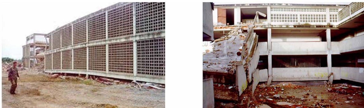
Figure 66. Raimundo Martínez Centeno high school, collapsed during Cariaco Earthquake (Venezuela) in 1997
