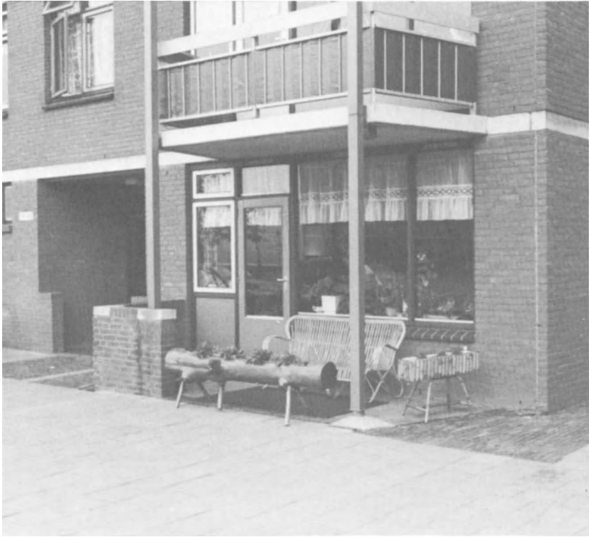
Figure 7. Ground floor residents in Simonsterrein housing personalize the territory outside their living-room door.
