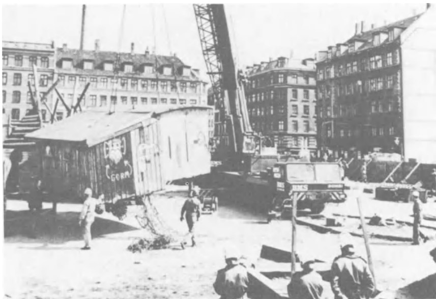
Figure 6. On April 22, under protection of 800 policemen, workers removed playing materials and structures from half the playground. After the police left, a few hundred local residents moved the materials and structures back to their original position. Copyright 1980 by Lars Bahl. Reprinted by permission.
