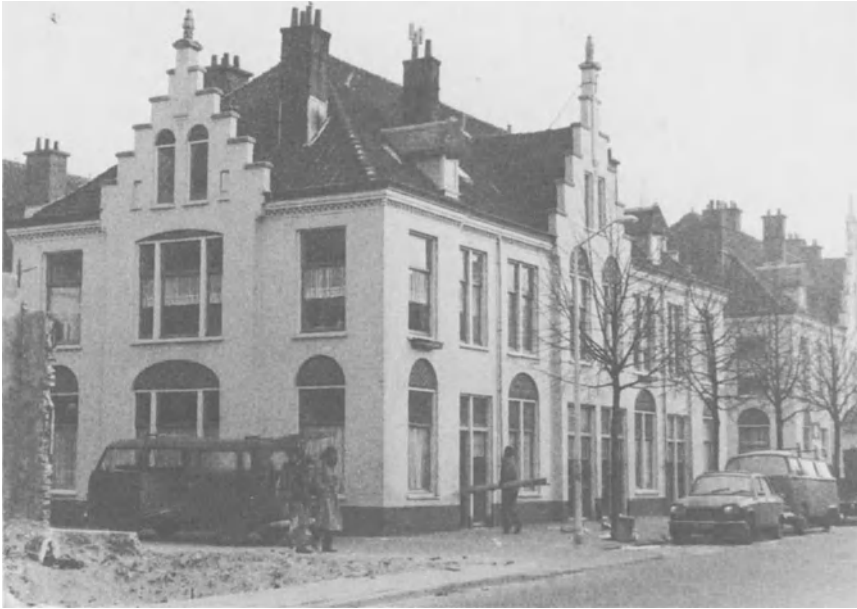
Figure 4. Rehabilitated housing in Schilderswijk.
