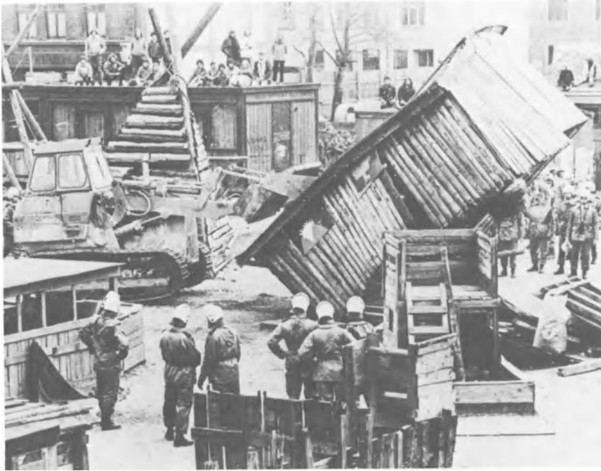
Figure 7. Police returned to Byggeren on April 29. This time, workers demolished the structures with bulldozers. Copyright 1980 by Henrik Saxgren. Reprinted by permission.
