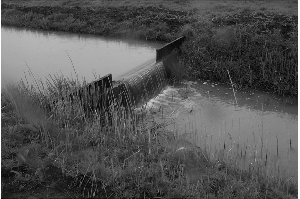
Figure 6.2 A small dam illustrating how different water levels can be regulated and fine-tuned between nature areas and agricultural areas.
