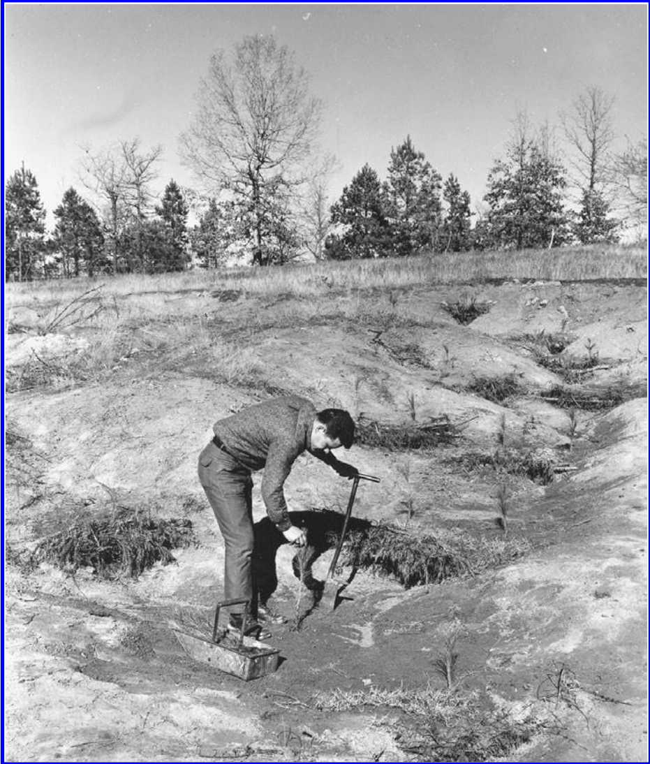
Figure 9.10 Brush dams to hold soil. Put in place before planting pines in this highly erosive Mississippi loess soil, the trees will stabilize the soil in 5 to 15 years, thus protecting the watershed. (USDA Forest Service photo)
