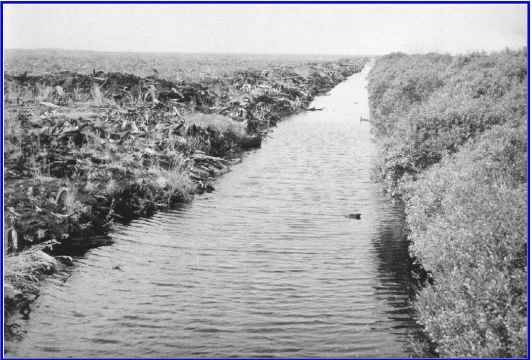
Figure 1.19 Into the 1960s, wetlands were drained for food crop production and to convert swampy sites to valuable tree species. Small ditches fed excess water into these larger canals that carried the water through locks to the sea. The locks prevented saltwater intrusion.
