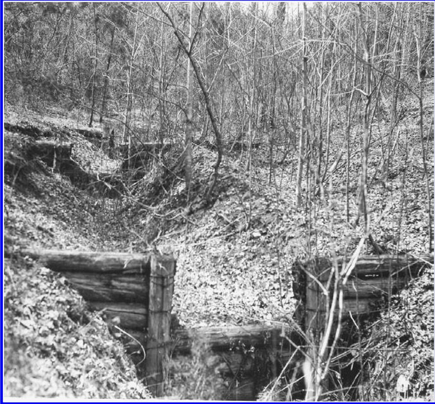
Figure 9.9 A check dam for watershed protection. These log structures in the eroded Appalachian country hold the soil, thus encouraging healing of a site as trees encroach following land abandonment from agriculture. (Tennessee Valley Authority)
