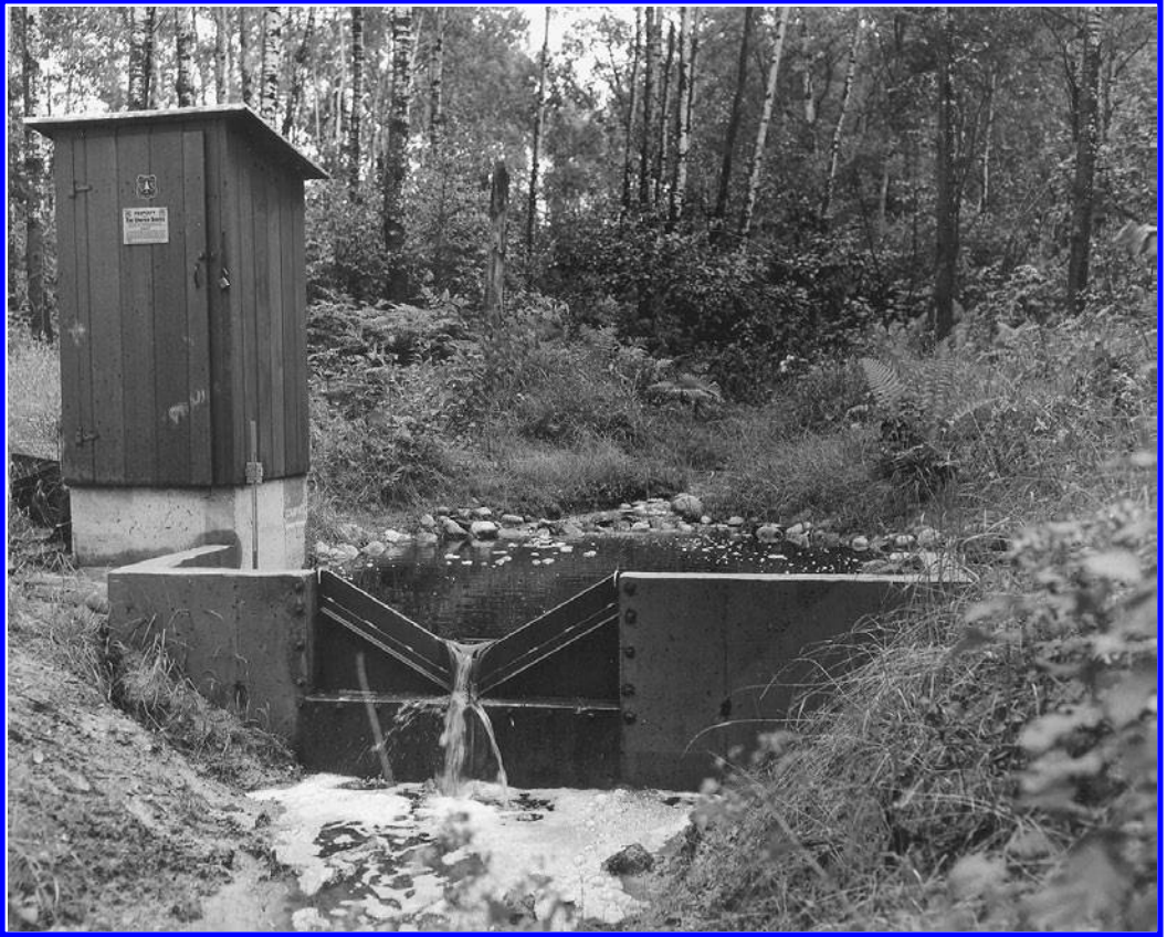
Figure 9.7 A V-notch weir. The flow of water in high-gradient creeks can be measured with 120-degree V-notch weirs. Shown is the flow from a small 30-acre watershed, tallying 0.3 cubic feet per second (cfs). The shelter houses an 8-day recording device. (USDA Forest Service photo)
