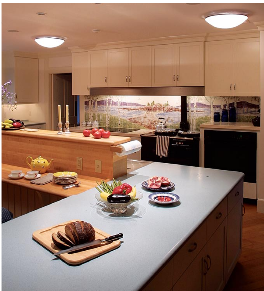
This kitchen has an amalgam of counter surfaces: a solid resin work counter in the foreground (for high resistance to staining and scratching), solid maple eating ledges and capping surfaces (for rich color and warmth where people eat), and a tile range-side work counter (for its high resistance to heat from hot pans). Each is beautiful and well serves its intended purpose.
