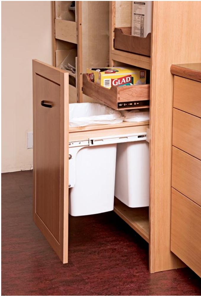
In my own kitchen, we attached a slide out platform that carries a pair of waste bins to the back of a false door front. A second pull out, also located behind the “door” and above the platform, provides storage for plastic sacks, ties and other items.
