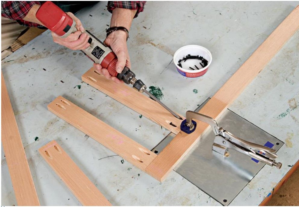
A plate-mounted clamp from Kreg Tool Co.—which I have inlayed into my work table—secures the face frame components together while I run in the pocket screws.
