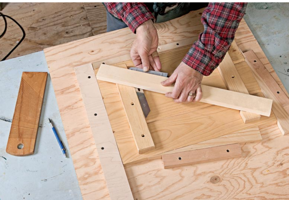
A bevel gauge determines the cut angle for the ends of the diagonal brace.
