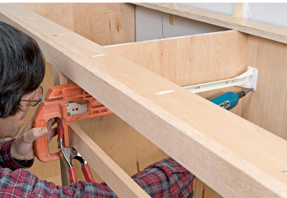
A commercially made jig holds a drawer guide rail in position, making it easy to attach the guide at the front and back of the cabinet.
