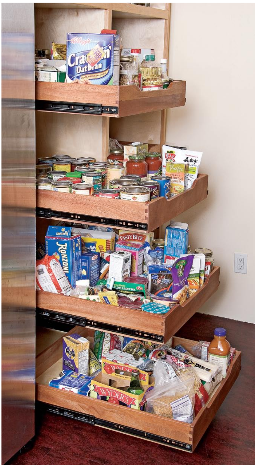
Slide-out shelves greatly improve the accessibility of kitchen cabinets. The dovetailed, solid-wood shelves shown here (in my own kitchen!) are installed on heavy-duty, full-extension slides.
