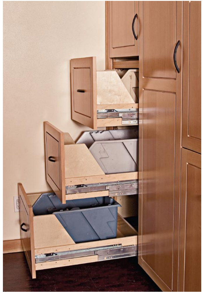
Here, three large drawer-faced pullouts make our recycling bins easy to access and to remove to place by the curb. The slides are heavy-duty Accuride® side mounts that can handle up to a 150-lb. load. (Overkill, certainly, but they should last for the life of the cabinets without a whimper!)
