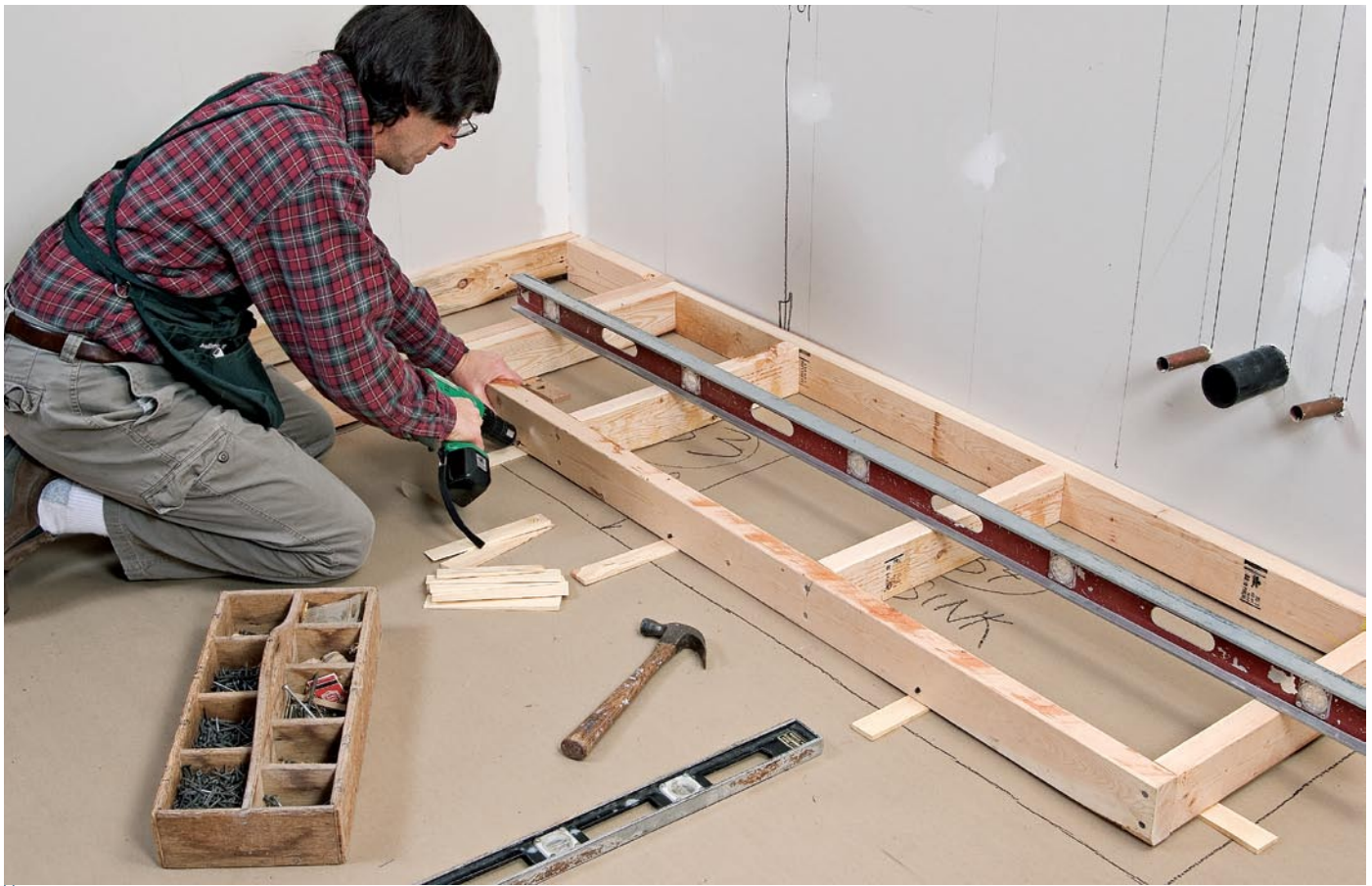
I screw the base frame to the floor, using shims where necessary to bring the frame level.
