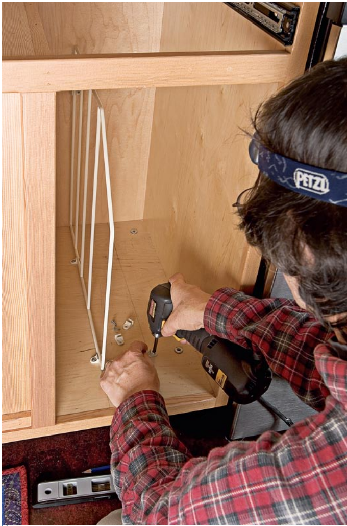
Tray dividers mount to clips screwed to the floor and back wall of the cabinet.
