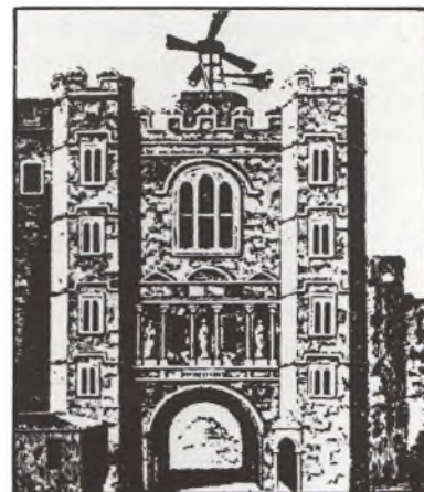
D A windmill put up at Newgate Prison by the Reverend Hales to get rid of the 'bad air' he thought caused disease. It made the prison less smelly.
