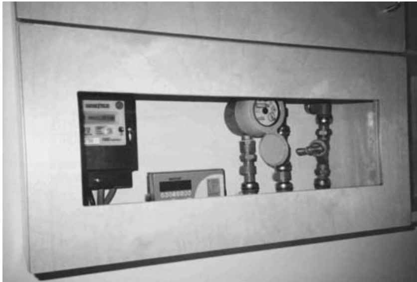
Fig. 7.1 Feedback designed into the BEDZED housing development in Sutton, UK. (a) and (b) Utility meters installed in the kitchen provide immediate feedback on resource consumption. Photographs courtesy of Bill Dunster Architects.
