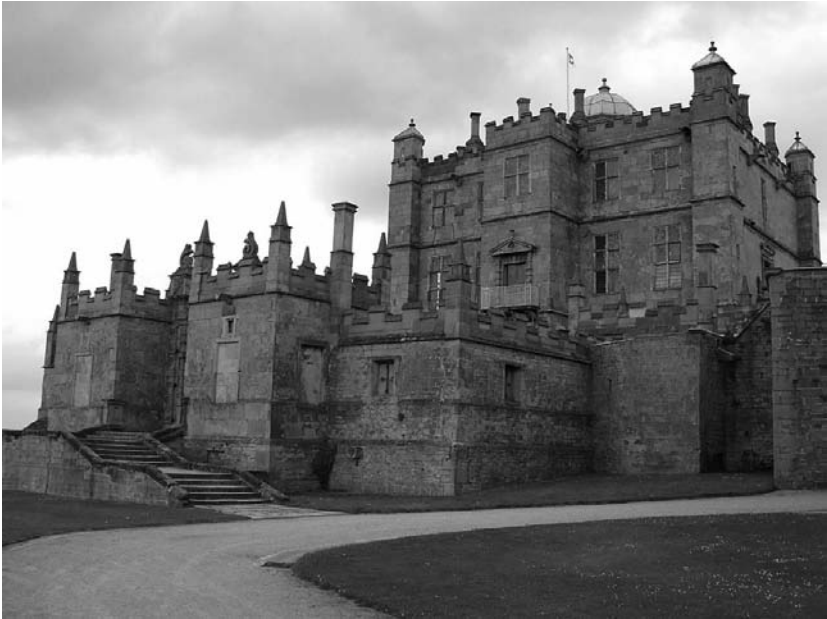
Figure 8: View of the approach to Bolsover Castle, Derbyshire. Photo: Mimi Yiu.
