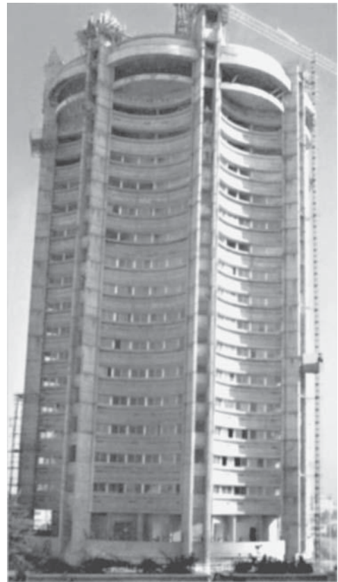
Curved beams in an office building.
