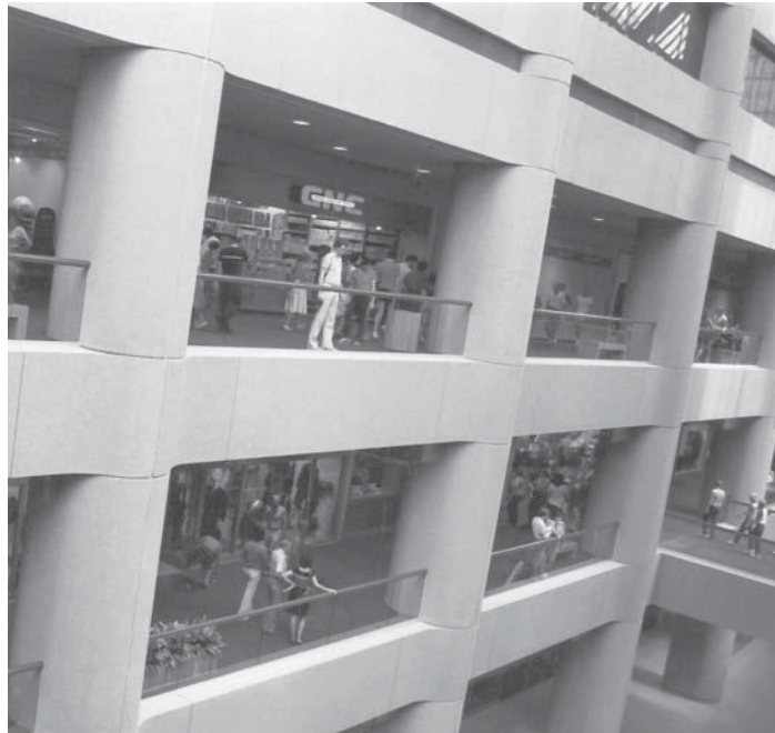
Columns supporting 52-story building, Minneapolis, Minnesota. (Columns are 96 × 64 in. with round ends.).
