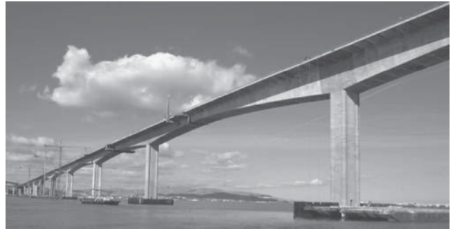
Benicia-Martinez Bridge, California.
