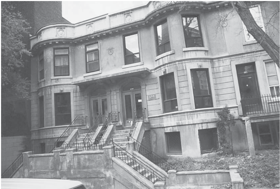
The Barkwick House, a three-story concrete building built in 1905, Montreal, Canada.
