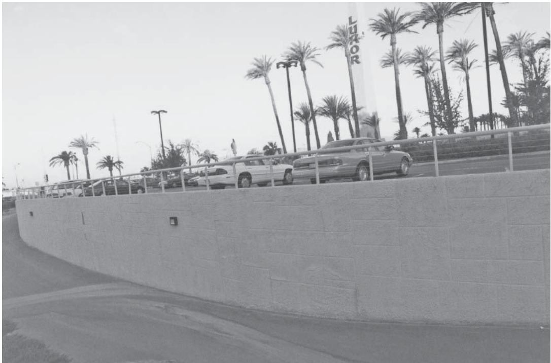
Retaining wall in a parking area.
