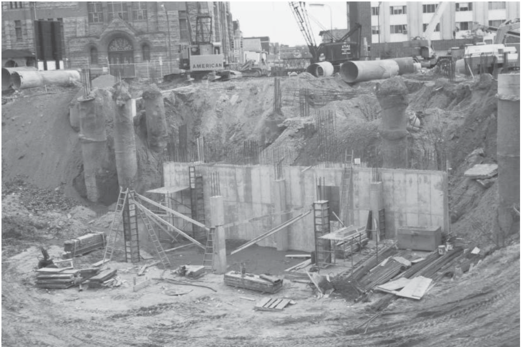
Wall and column footings, partly covered.
