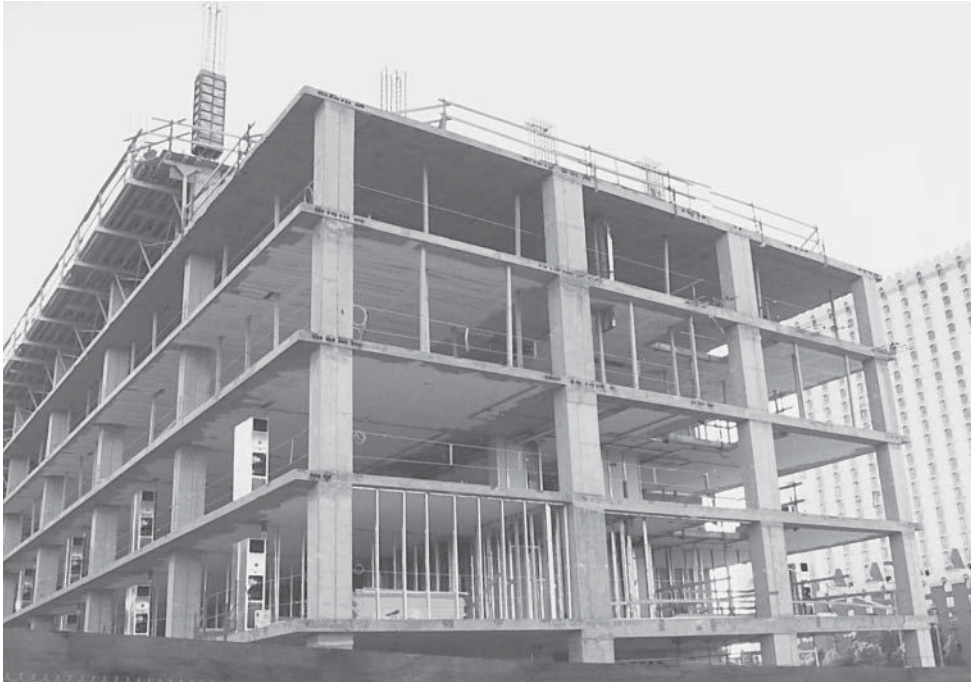
Flat-plate floor system.
