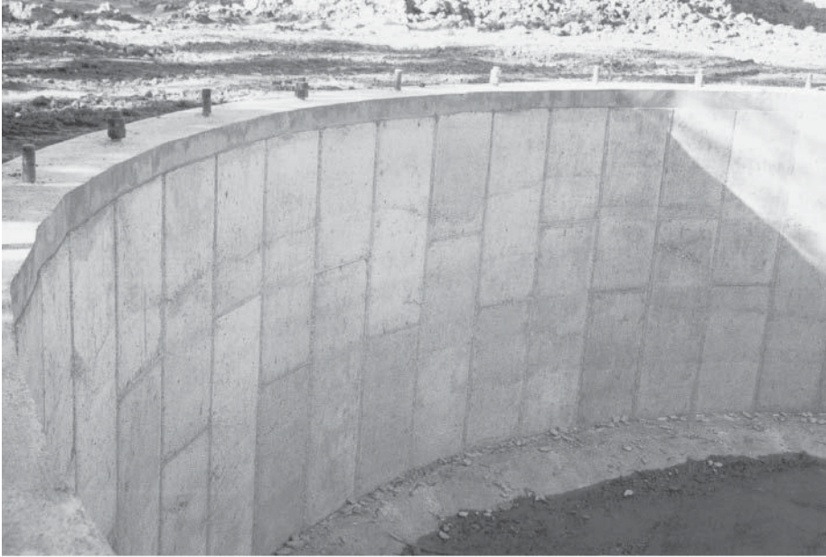
Reinforced concrete retaining wall.
