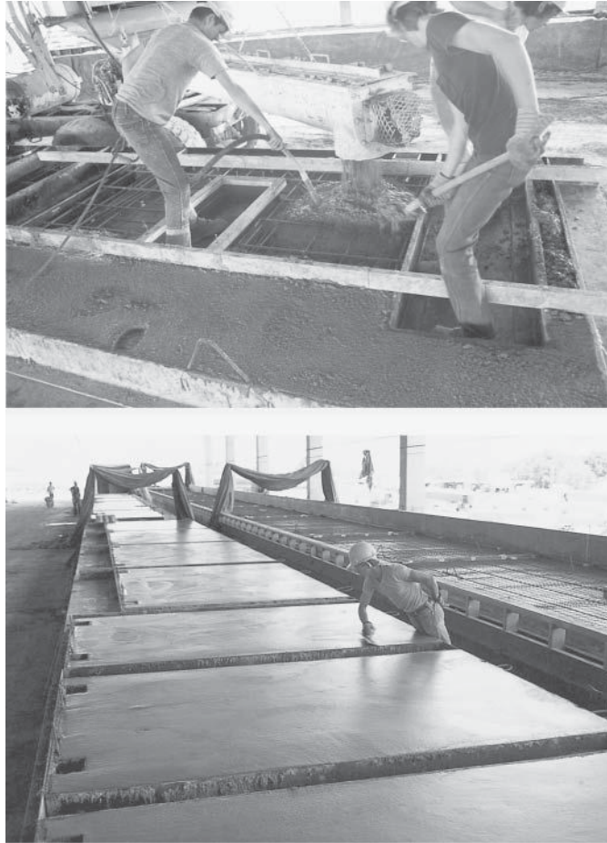
Casting and finishing precast concrete wall panels.
