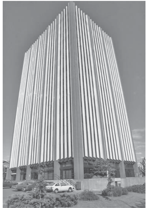
Reinforced concrete columns supporting an office building, Toronto, Canada.
