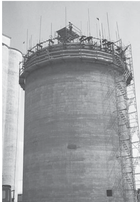
Reinforced concrete grain silo using the slip form system. Brookings, South Dakota.
