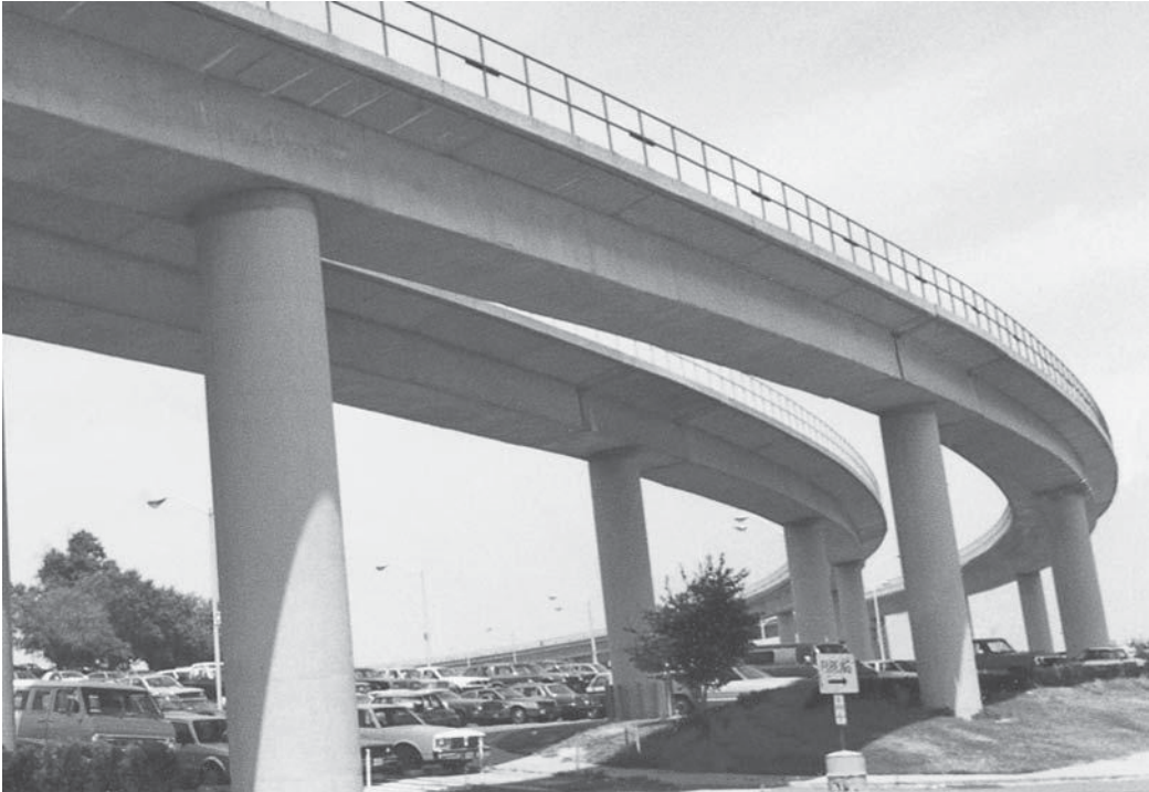
Curved-beam bridge, Washington, D.C.
