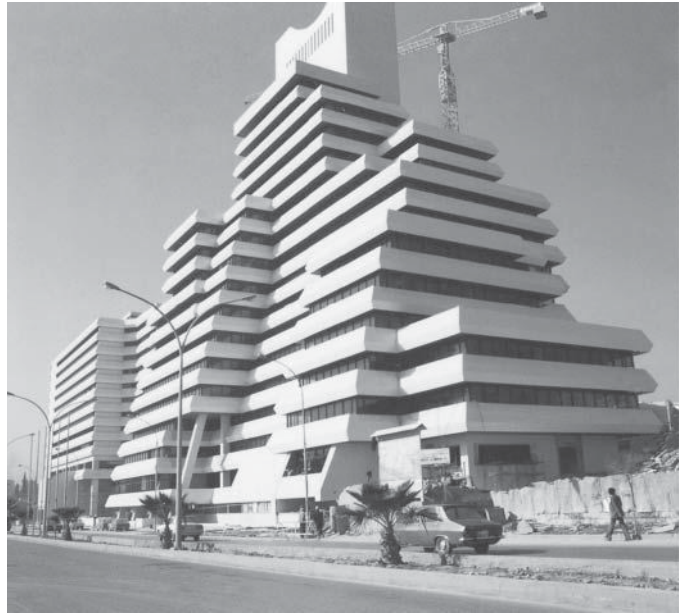
Reinforced concrete office building, Amman, Jordan.
