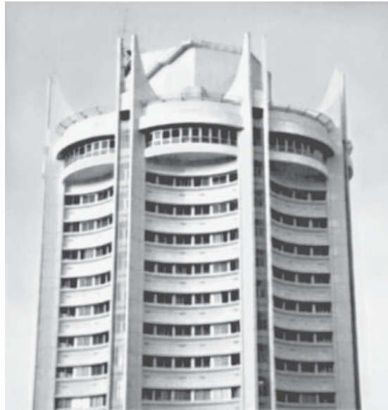
Circular beams in an office building.
