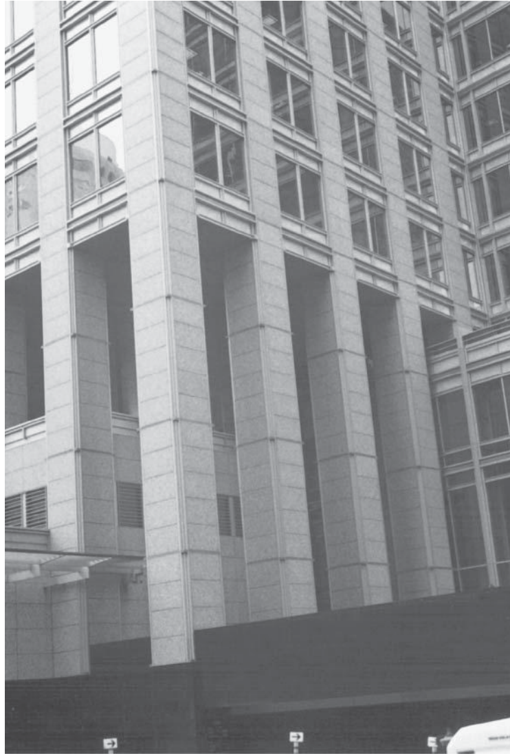
Long columns in an office building.
