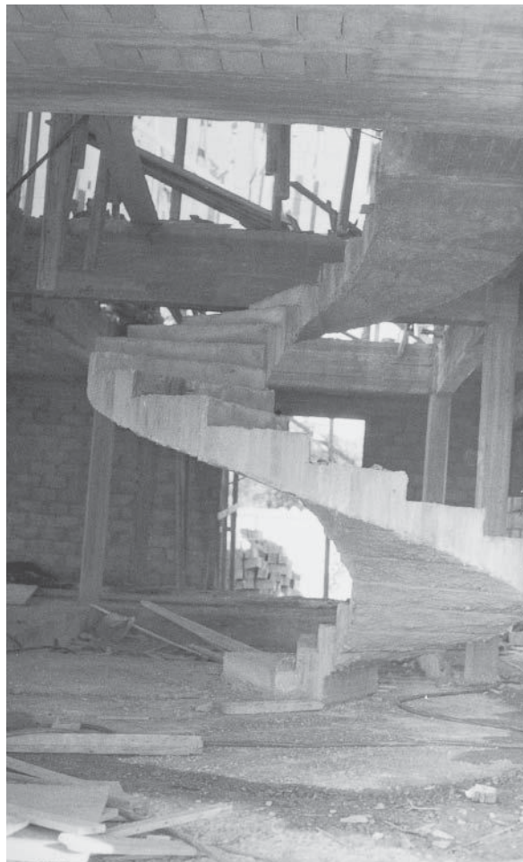
Reinforced concrete helical staircase.
