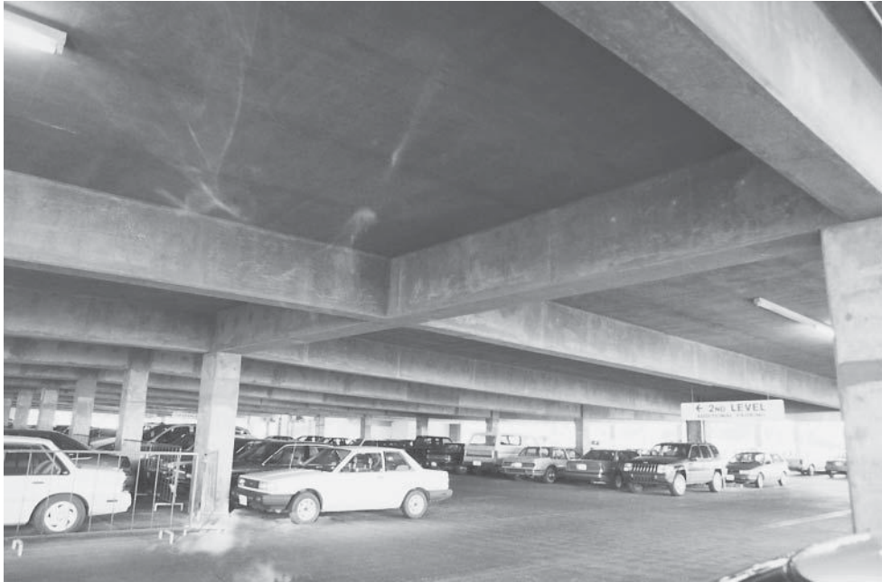
Slab on beams.
