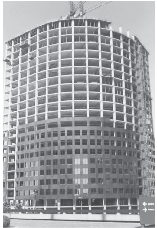
Office building under construction, New Orleans, Louisiana.
