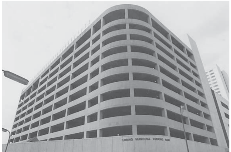
Reinforced concrete parking structure, Minneapolis, Minnesota.
