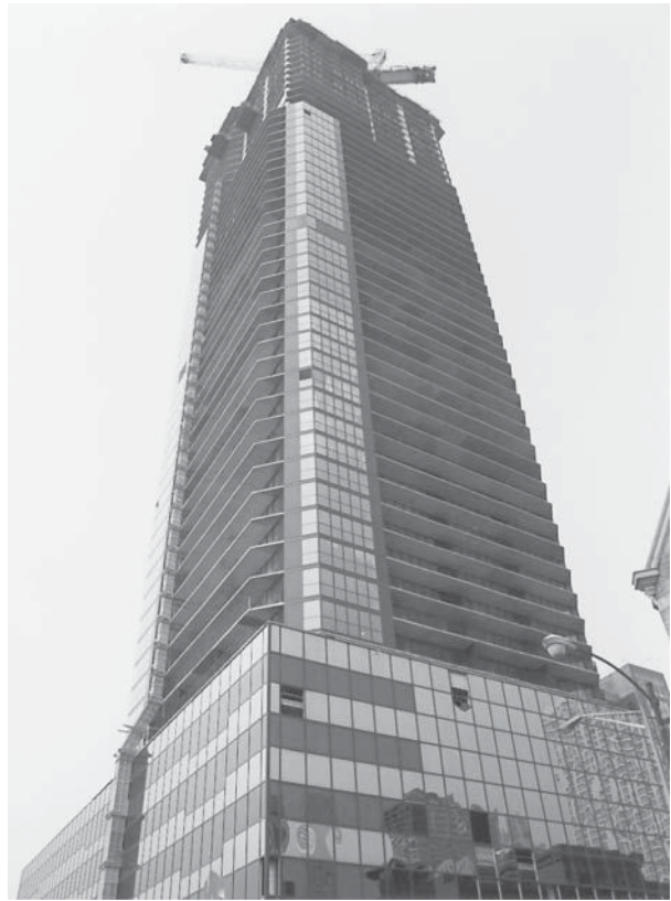
Office building under construction, Chicago, Illinois.
