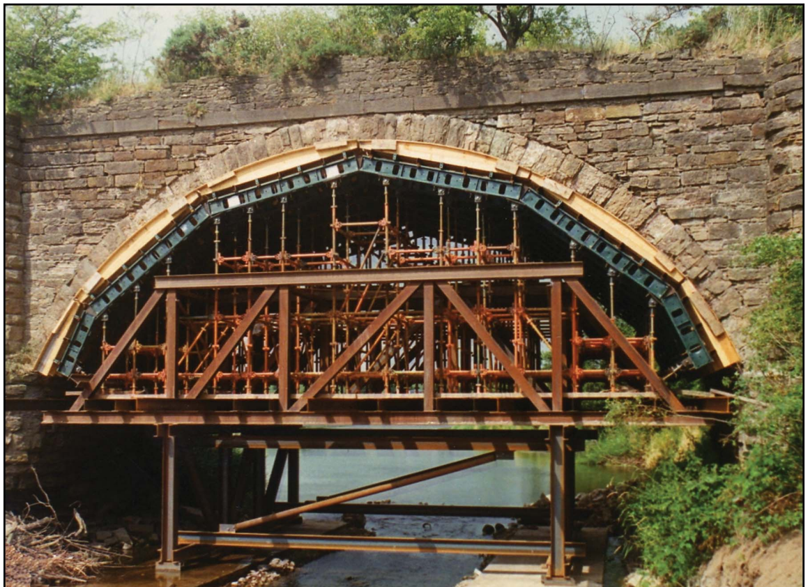
Figure 16 Structural engineers also work for constructors, designing complex temporary supports. This example is for the refurbishment of a historic railway viaduct near Kilmarnock in Scotland
