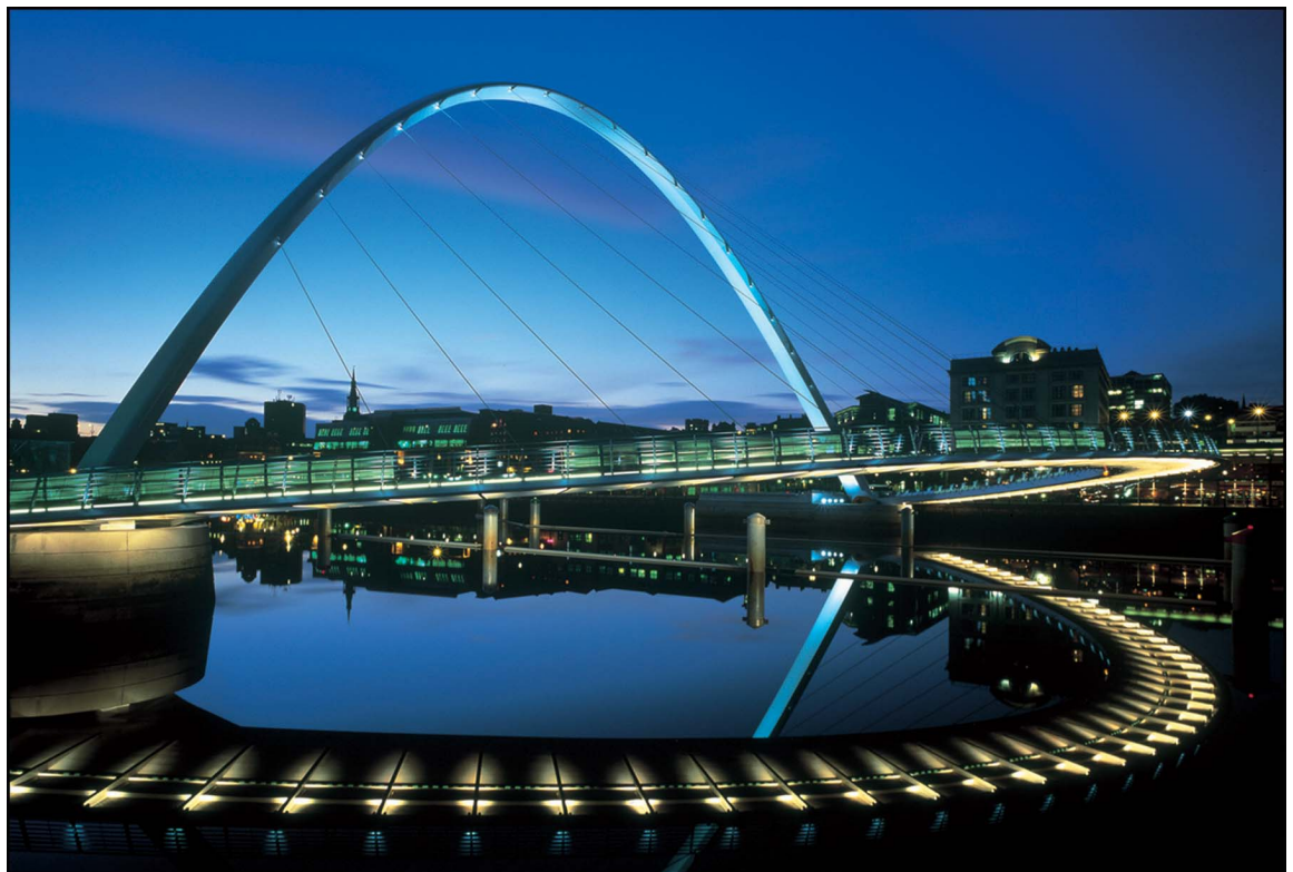
Figure 2 Structural engineers devised this new take on the idea of a rotating bridge. This is the Gateshead Millennium Bridge across the River Tyne
