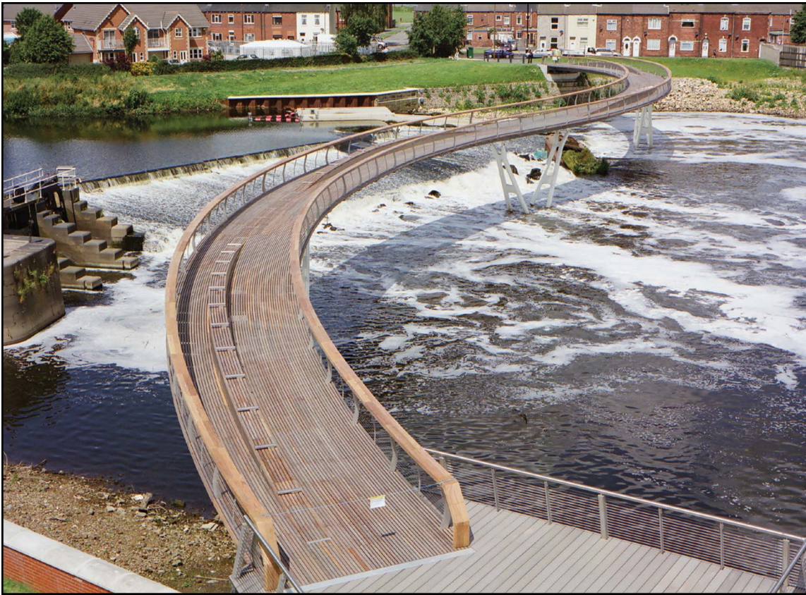
Figure 8 The art of the structural engineer lies in being able to use simple sketches as in the previous illustration to understand and develop complex designs, as the finished Castleford Bridge shows
