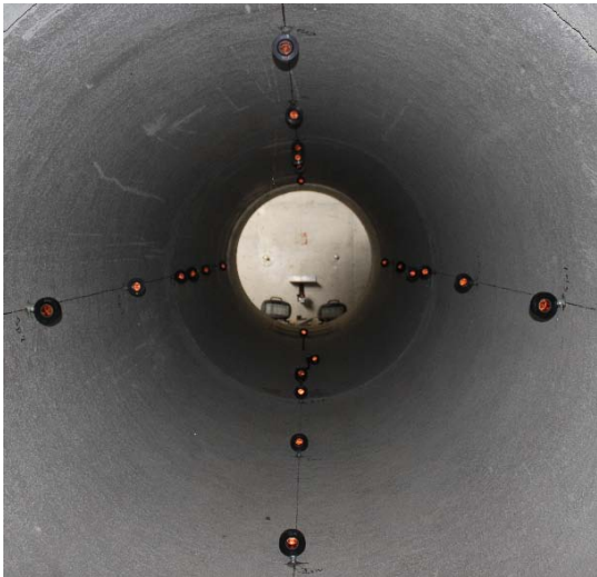
Figure C.11. View of the prisms after placement in the 48 in (1220mm) diameter reinforced concrete pipe.
