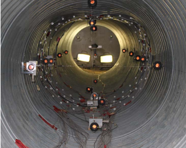
(a) Internal view
