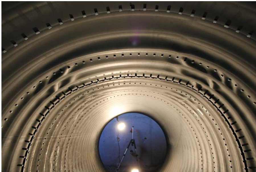
Figure C.97. HDPE pipe after ultimate limit state test.
