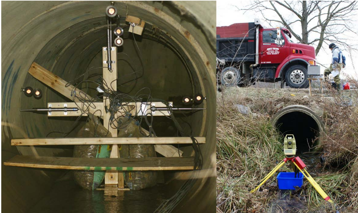
a) Close-up view of instrumentation
