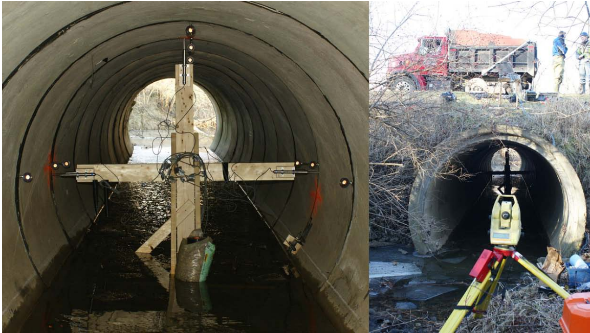
a) Instrumentation setup inside the culvert
