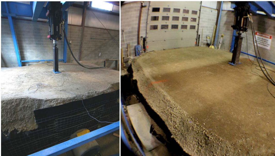
Figure C.16. Actuator on the reaction frame, applying load to steel pad on the ground surface over the reinforced concrete test pipes (24 in diameter specimen left hand side and 48 in diameter specimen on the right hand side)
