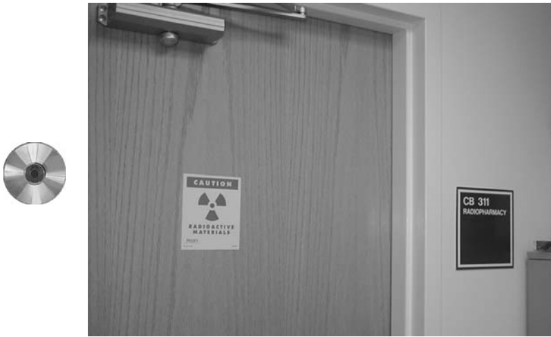
Fig. 1-4. Entrance door to the radiopharmacy must be locked at all times and show a caution sign for radioactive materials.
