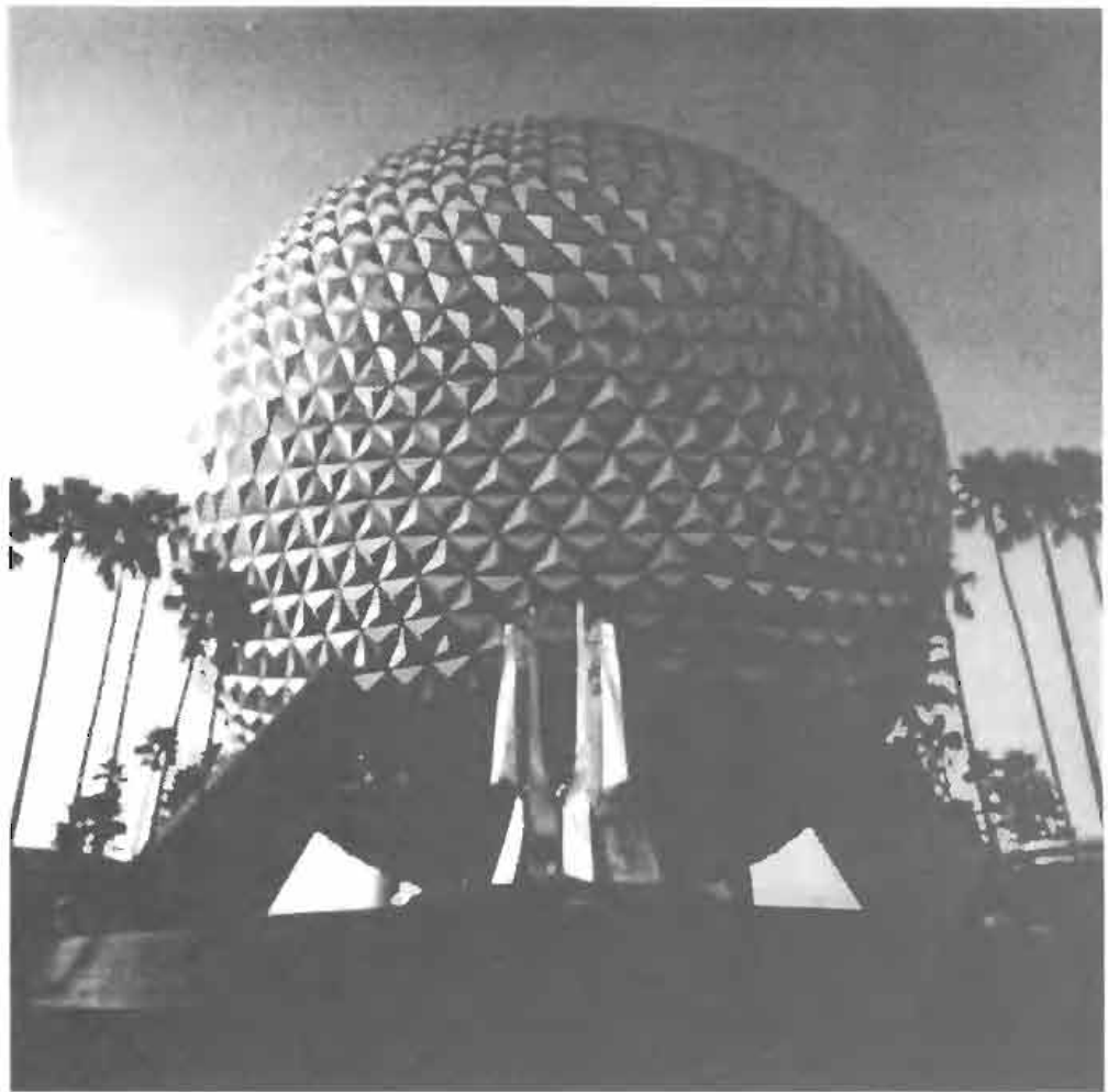
Figure 3 Geodesic globe named Spaceship Earth , the symbol of Disney Epcot Center in Orlando, Florida. Fifty meters in diameter, it contains a ride highlighting the history of communication from cave dwellers to the present. The spherical shells surrounding our black hole are openwork lattices, not a closed surface as shown here © Disney Enterprises, Inc
