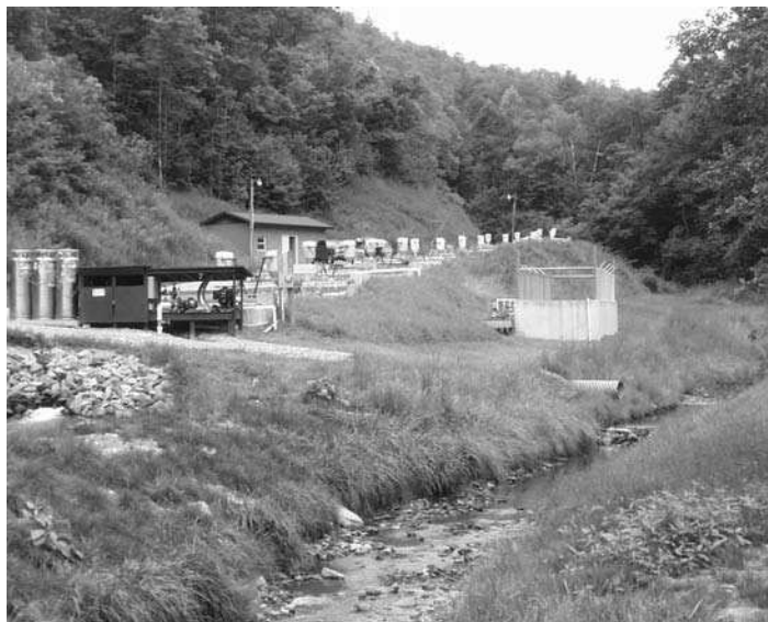
Fig. 9.3. A small flow-through facility producing rainbow trout in the Appalachian Mountains of North Carolina. Water from a small stream is diverted into the raceways in the distance and then returned to the stream, after treatment, in the foreground.
