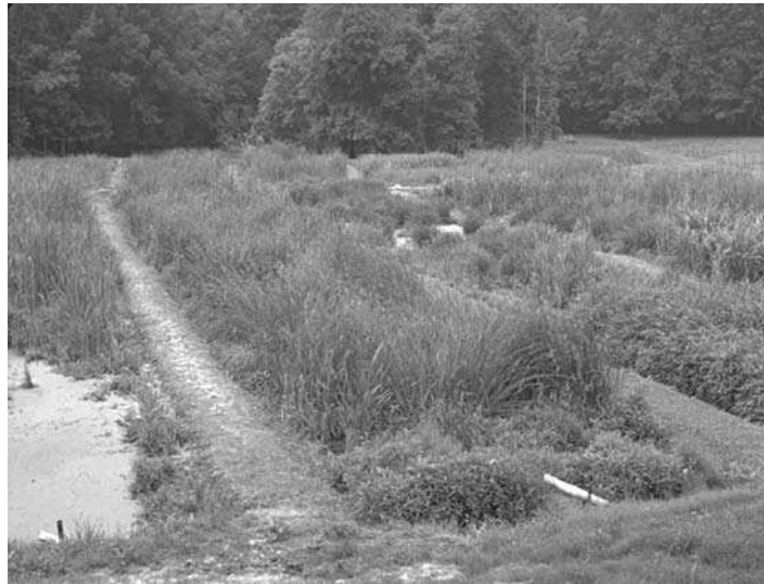
Fig 6.8. Constructed wetlands used to treat effluents from a fish pond. Water enters the center cell near the bottom of the photograph, flows through the emergent vegetation, and exits the cell in the distance.
