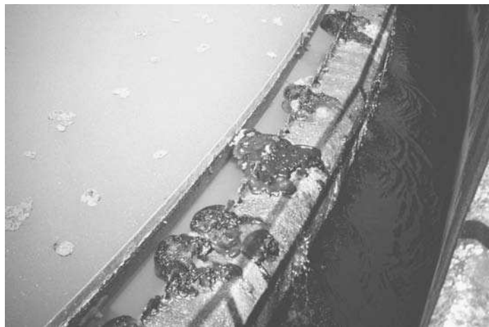
Fig. 10.9. Some floated solids are captured by a scum baffle in the radial-flow, offline settling tank at the Pennsylvania Fish and Boat Commission's Big Spring Fish Culture Station, Newville, Pennsylvania.
