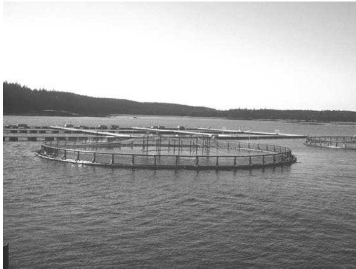
Fig. 8.7. Two styles of modern net pens. In the foreground is a round pen made of high-density polyethylene. In the back are square, steel-collared pens. Choosing the proper pen design for prevailing site conditions can significantly reduce risk of escapes. Barely visible in the photograph is netting over the round pen to prevent access by birds.
