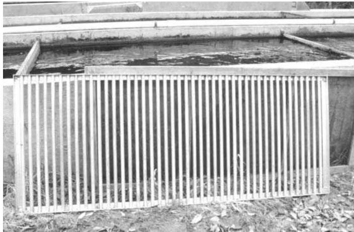
Fig. 9.9. A fish barrier screen of vertical metal bars.
