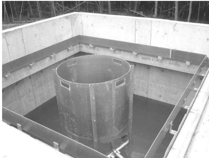
Fig. 10.8. A center-fed radial-flow settler (without water) at the Maine Department of Inland Fisheries and Wildlife's Enfield Fish Hatchery contained in a rectangular concrete vessel. Note the turbulence dampening cylinder for the inlet flow (located at the center of the vessel) and the effluent collection launder (located about the perimeter of the vessel).
