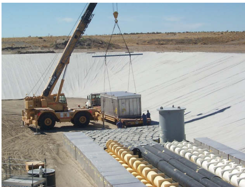
FIGURE 2.4 RCRA requirements for disposal of MLLW include use of an impermeable liner and leachate collection system to provide total containment of hazardous chemicals for at least 30 years. Here, a large box of macroencapsulated waste is being placed in a RCRA-compliant disposal facility at Hanford. Source: DOE Richland Operations Office.
