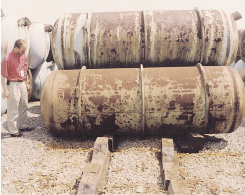
Figure 6.1 Cylinders containing about 14 tons of depleted-uranium hexafluoride are stored outdoors. These cylinders are made of carbon steel with wall thickness of 1/4 or 5/16 inch. The stacking arrangement often prevents worker access for inspection or maintenance. Source: http://web.ead.anl.gov/uranium/guide/ .
