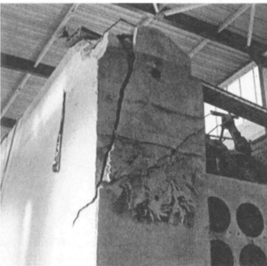
Figure 11-6. The PLUTO Test Reactor External Storage Block Split Using Expansive Grout.
