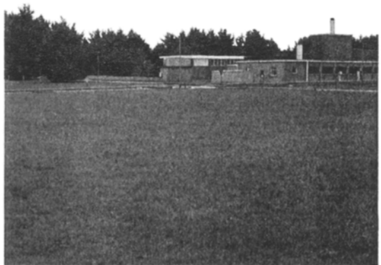
Remediated site following demolition and restoration
