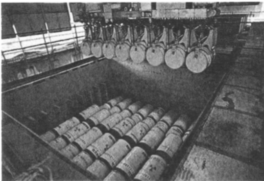
Figure A1-5. (a) Japan HLW Disposal Concept (photo courtesy of JNC); (b) Low Level Waste Disposal at Rokkasho-Mura (photo courtesy of JNFL); (c) Spent Fuel Storage Facility at Rokkasho-Mura (photo courtesy of JNFL).
