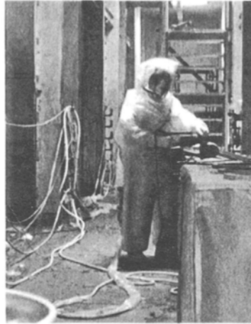
Figure 7-1. Full Pressurised Suit Working During Decommissioning of an Alpha Laboratory.
