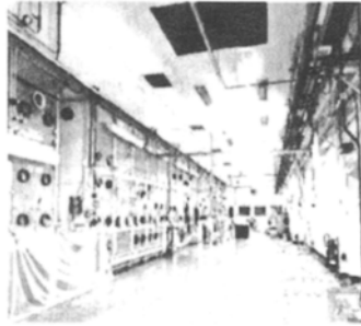
Figure 7-8. Harwell Glovebox Dismantling.
