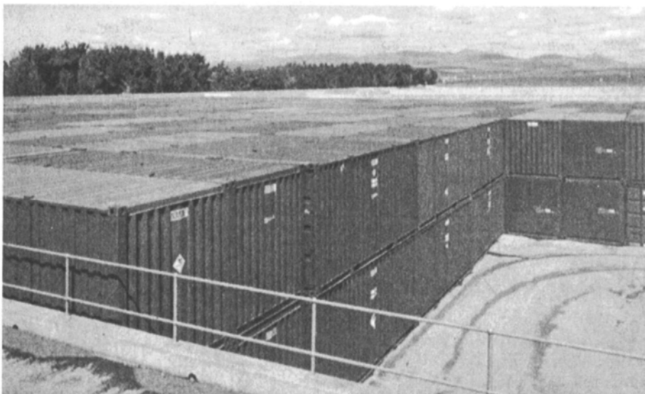
Figure 19-6. Stacked Full Height LLW ISO Containers in Concrete Vaulted Disposal Facility (Photograph courtesy of BNFL).
