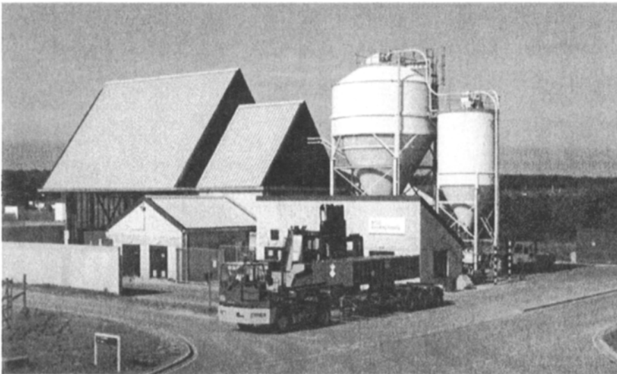
Figure 19-8. Grouting Facility for Containerised LLW (Courtesy BNFL).
