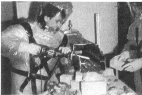
Manual dismantling of glovebox within pressurised suit area
