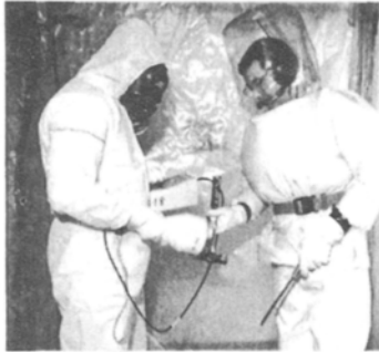
Figure 7-1. Full Pressurised Suit Working During Decommissioning of an Alpha Laboratory.
