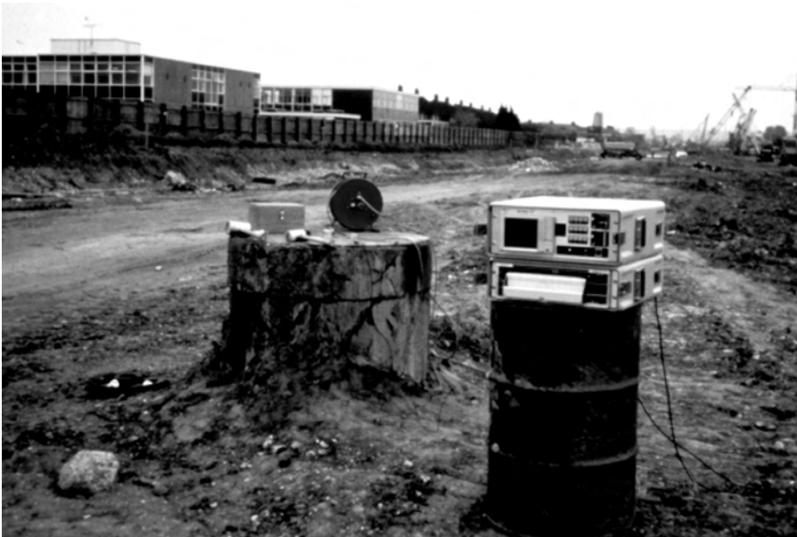
Figure 8.3 The 'MIMP' equipment set up to test a drilled shaft
