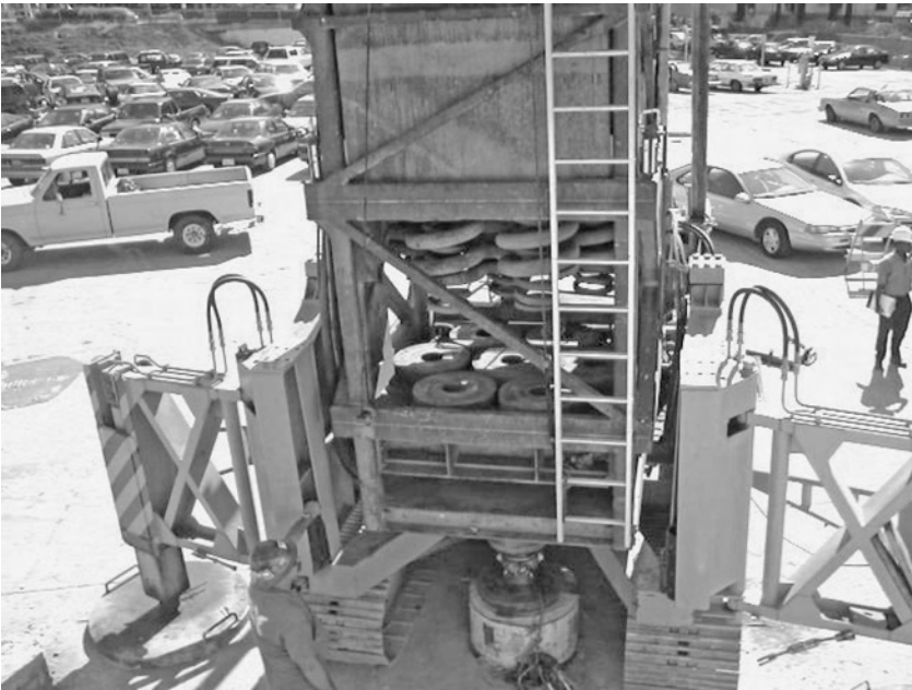
Figure 6.19 The Fundex pile-load test (PLT) drop-mass showing the multiple springs. Reproduced by permission of American Piledriving, Inc., California, USA
